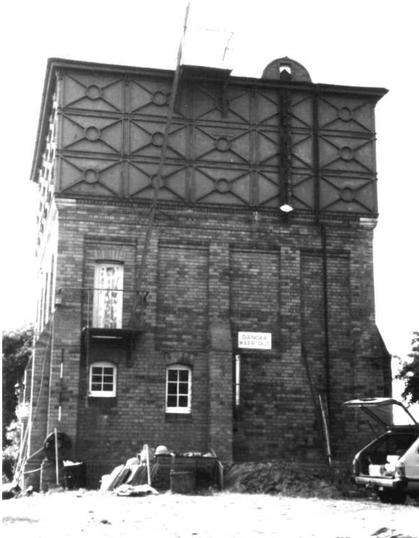
Figure 18.3: An industrial archaeological problem – Dark Lane Water Tower, Wellington. This unlisted, redundant structure was altered to extend domestic accommodation but recording was assisted by the discovery of the original construction drawings of 1896 (Murless 1995).
