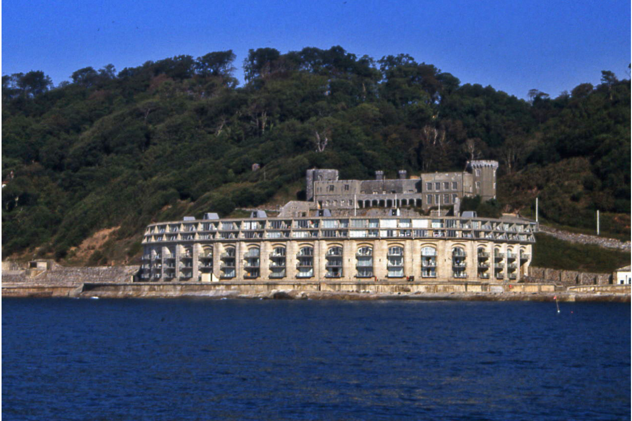
Figure 14.3: Picklecombe Battery. The castellated barracks of the 1840s battery can be seen at the rear with the 1860s multi-tier casemated battery, converted to flats, in front. Photograph: Andrew Pye, Exeter City Council.
