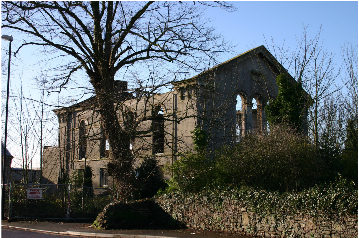
Figure 14.2: Wesley Chapel, Kingswood, built in 1844 as the successor to the original Colliers' School and Meeting House. It closed in 1978. It is increasingly apparent that nonconformity played an integral part in the industrial development of the South West, promoting entrepreneurship and education, and providing centres of social activity. Photograph: David Dawson.
