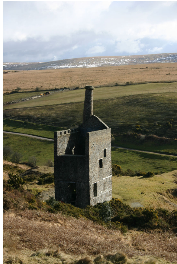
Figure 14.1: Wheal Betsy in the care of the National Trust on the western fringes of Dartmoor. A type of engine house once commonly found from Gloucestershire to Cornwall and a reminder of the rich mineral heritage of the South West and of how little is known and understood about the archaeology of its exploitation. Photograph: David Dawson.
