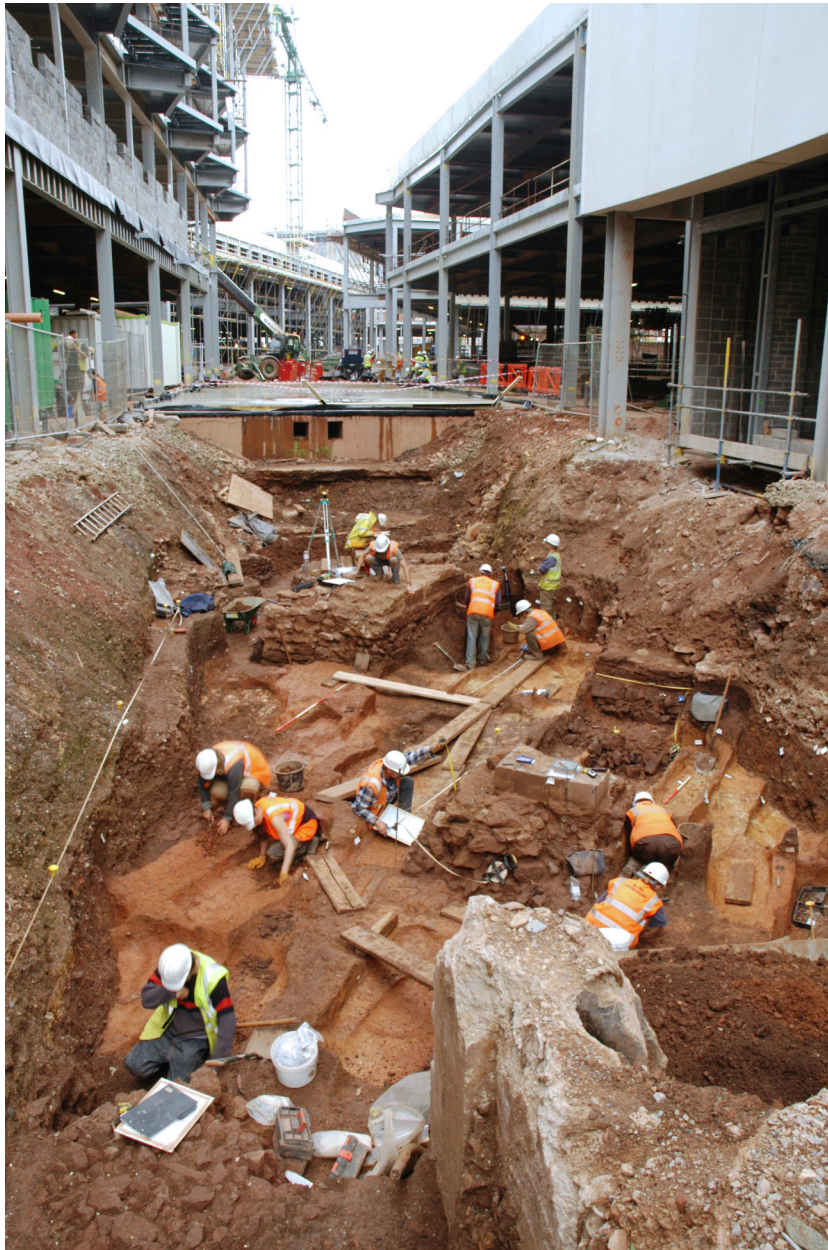
Figure 12.1: View east up the new Princesshay, Exeter, during the excavation of a large tank. The remnants of the north aisle of the medieval Blackfriars' church can be seen, including the north wall (top centre) and a pier base (centre) of the nave arcade. More than 50 separate graves, often intercutting, were discovered, the bases of several of which can be seen in the underlying clay subsoil. Photo: Gary Young, ©Exeter Archaeology
