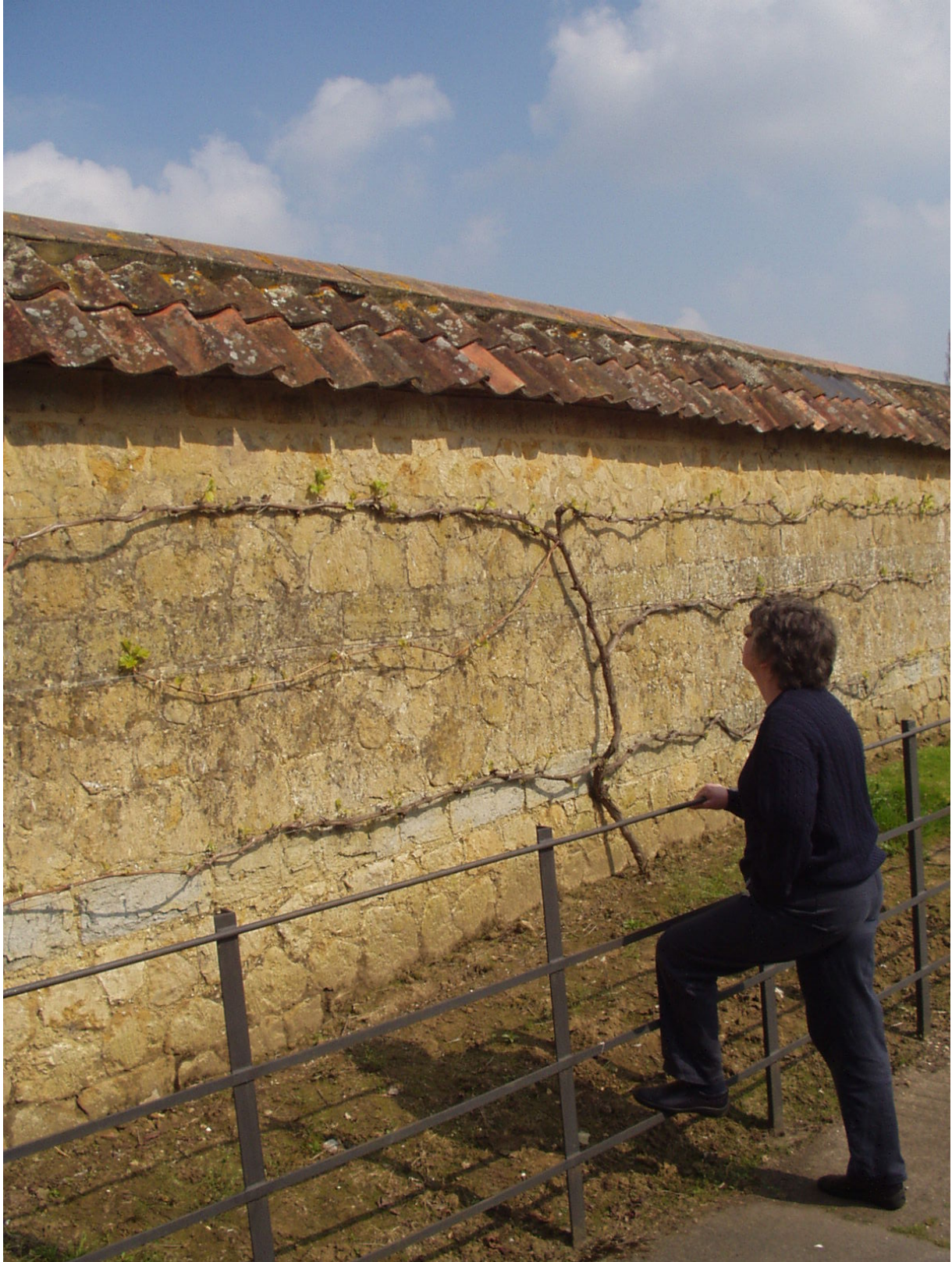
Figure 2. Tile coping of the walled garden wall at Barrington Court, Barrington. The wall is made of Moolham Stone and Blue Lias limestone laid in decorative alternating courses.
