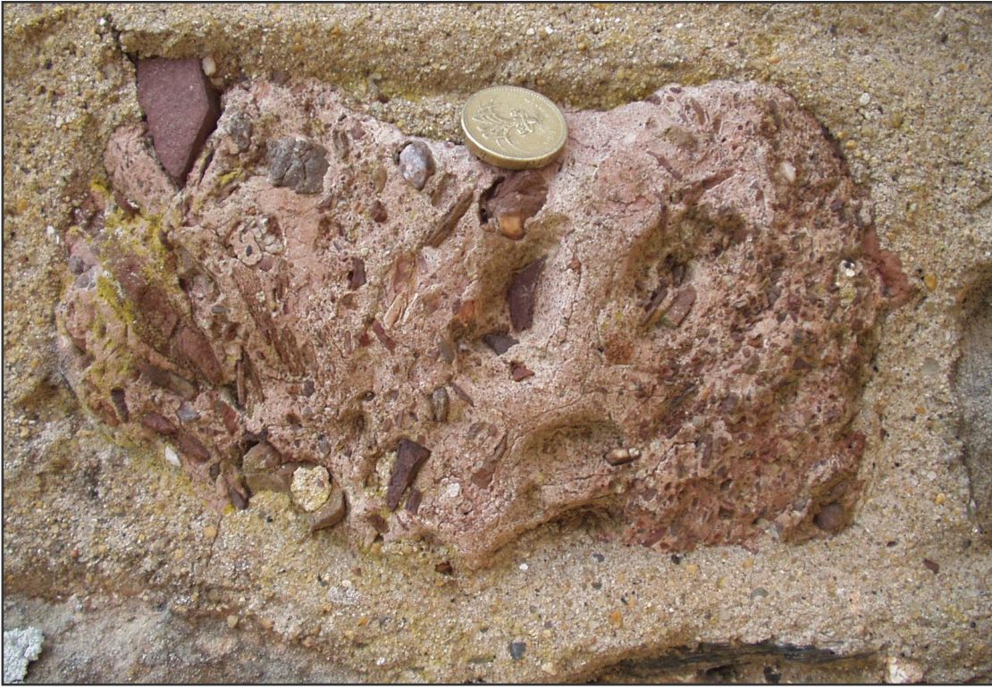
Figure 1. Block of matrix-supported red breccia, south porch of St. Swithin's church, Woodbury.
