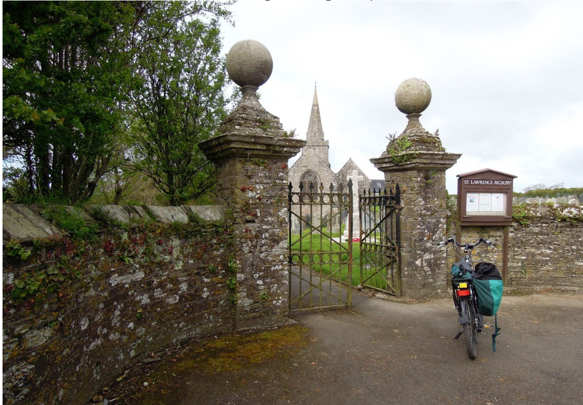
Figure 7. Entrance to the churchyard, St Lawrence' church, Bigbury. The wall and gateposts are of the local slate from the Bovisand Formation. The gateposts are topped by granite balls.
