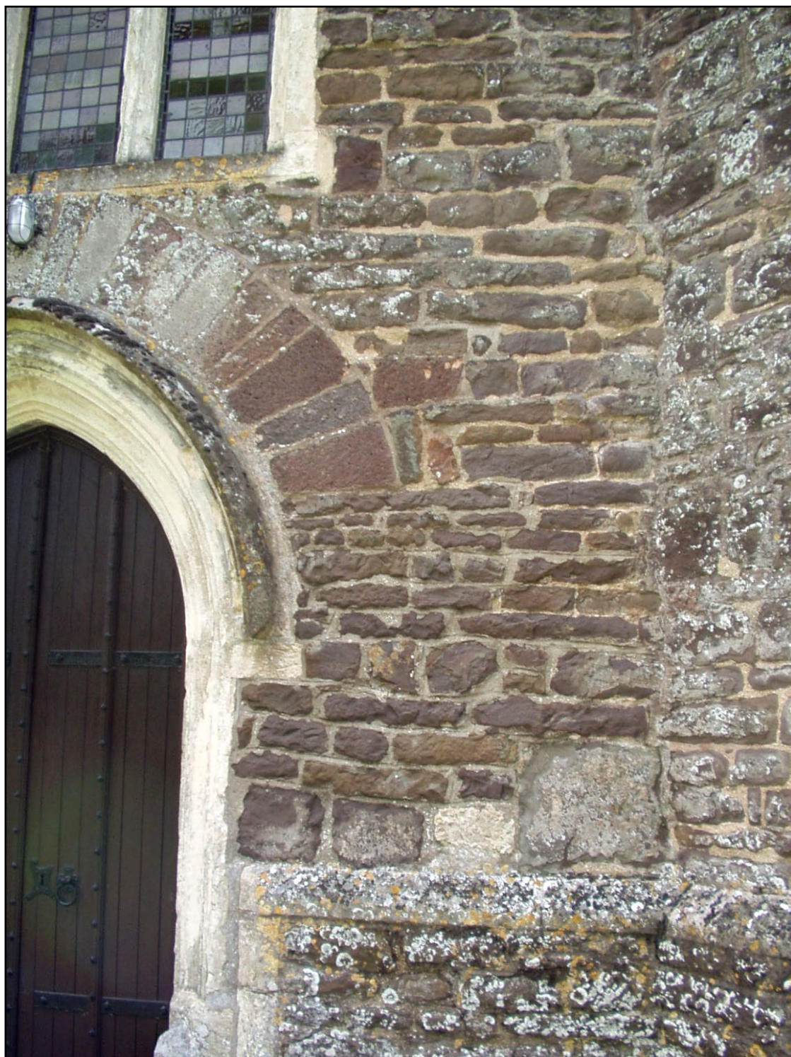
Figure 1. Tower of St John's church, Plymtree. Vesicular lava is used for the relieving arch above the doorway and a few blocks occur also in the wall but most of the stone in the wall is from Bude Formation sandstone from Upton Farm quarry. The dressings round door and window are of Beer Stone.
