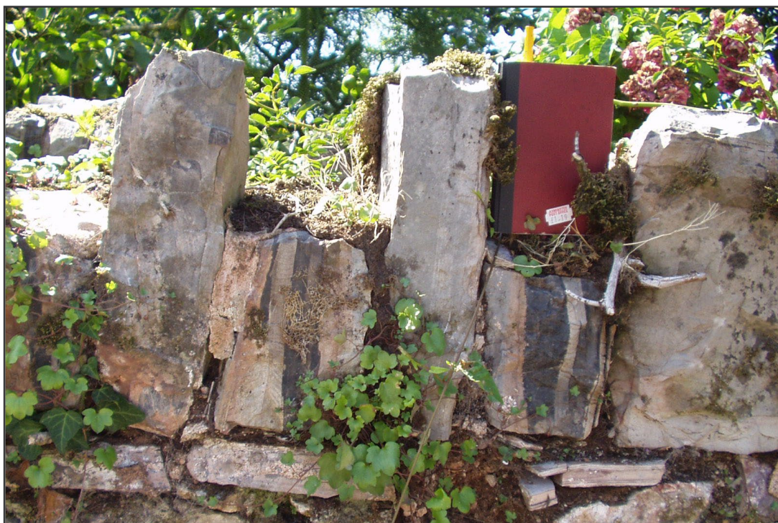
Figure 2. Coping of roadside wall, Smithincote. Pale grey limestone with black chert bands.
