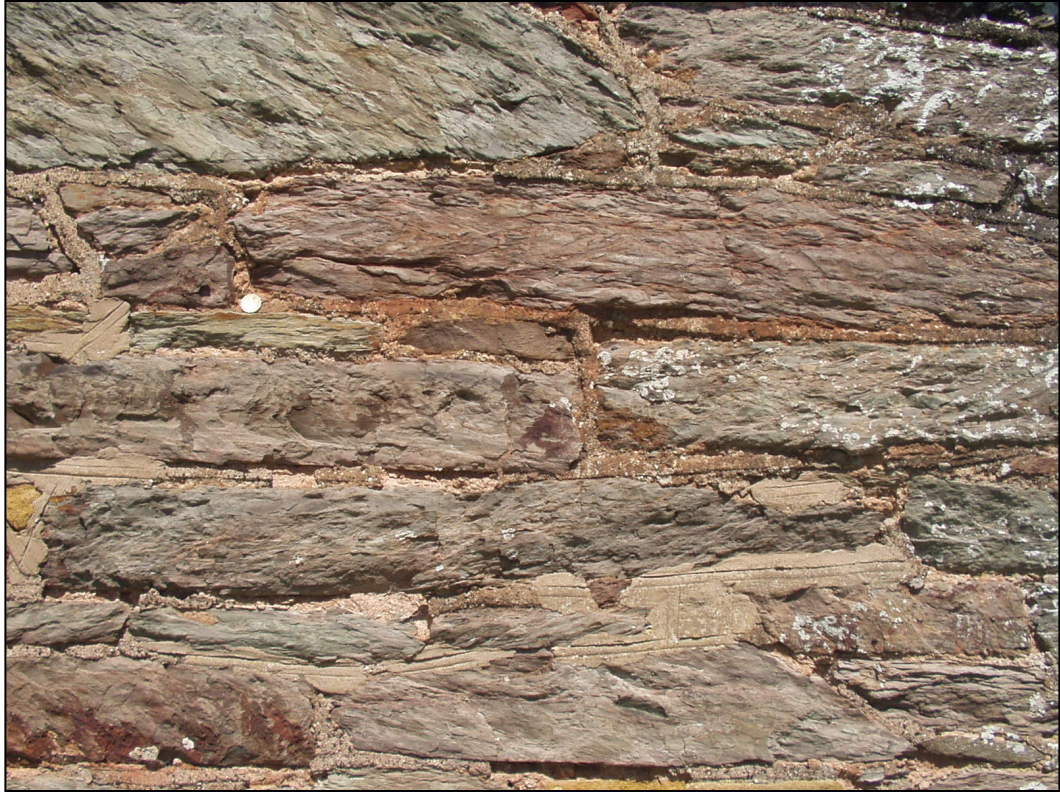
Figure 1. Typical Mortar Slate, St John's church, Durston.
