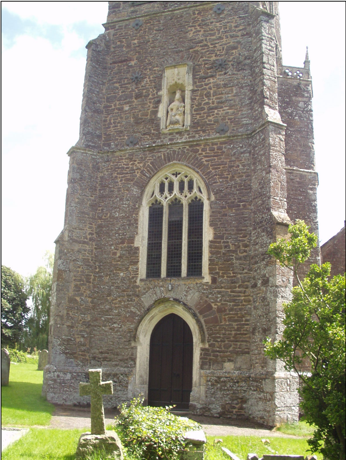
Figure 2. Tower of St John's church, Plymtree. The quoins of the buttresses and relieving arch over the door are a mixture of Exeter Volcanic Series lava and pale grey calcarenite (Rock-type 52). The dressings of window and door are of Beer Stone. The rubble wall is a mixture, mainly of Bude Formation sandstone with some Exeter Volcanic Series lava.
