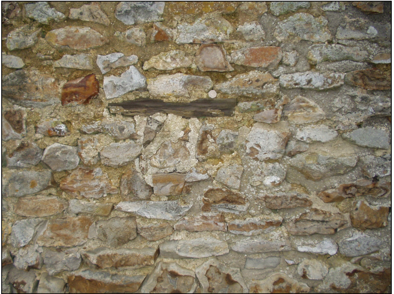
Figure 1. Black shale referred to Building Stone Code 6 in chert rubble wall, St Gabriel's chapel, Morecombelake.
