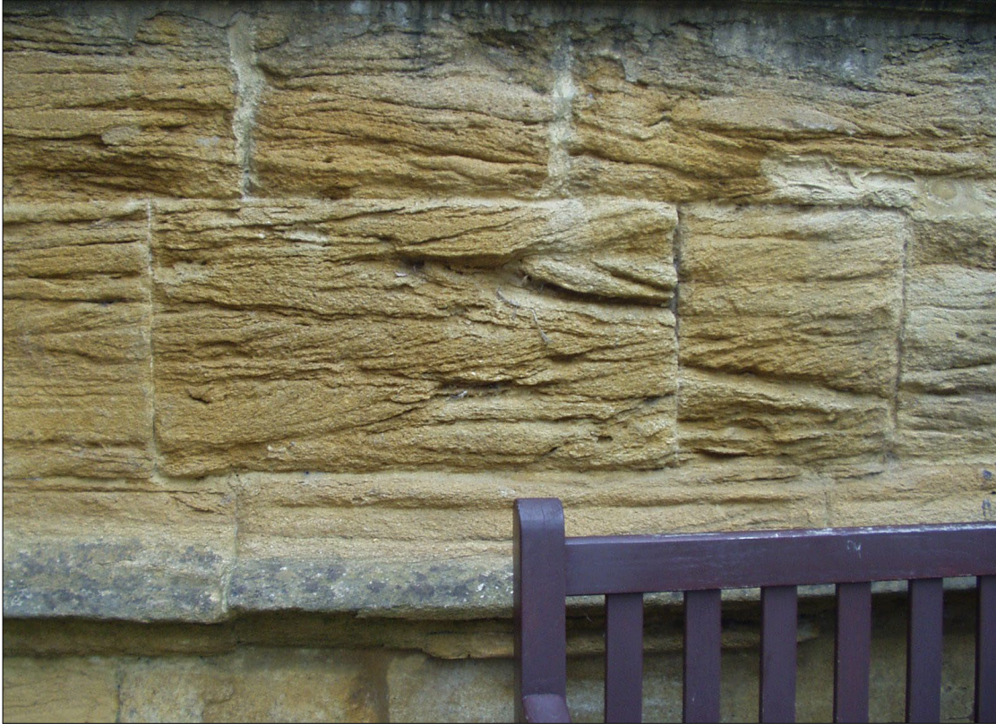
Figure 2. South aisle, St Mary Magdalene's, Taunton. Differential weathering has picked out the cross-bedding.
