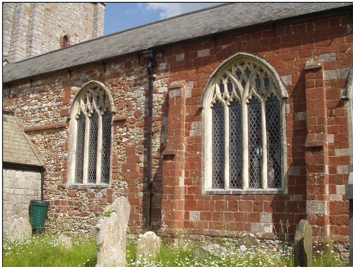
Figure 1. South aisle of St Michael's church, Kingsteignton. The eastern bays are composed of local red sandstone with a few pale grey blocks of calcarenite from the Upper Greensand (Rock-type 52). The window tracery is of Beer Stone.
