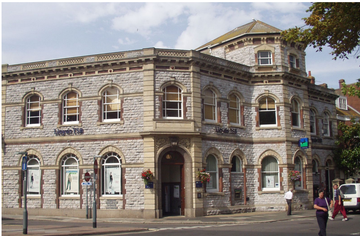
Figure 8. Lloyd's Bank, Exmouth. The walling is of mid-Devonian limestone from Torbay on a plinth of granite, and with dressings of yellow Bath Stone and purple Pocombe Stone (Exeter volcanics).
