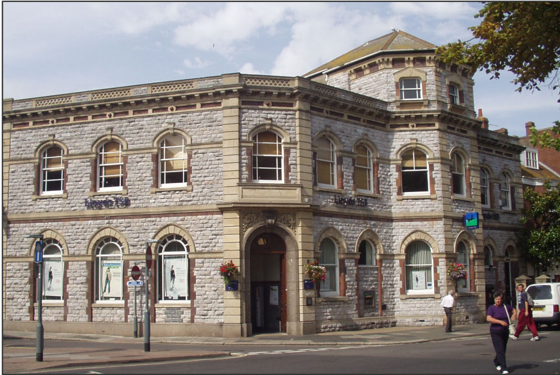
Figure 1. Lloyds Bank, Exmouth. Pale grey limestone rests on a plinth of Dartmoor granite. The dressings are mainly of Bath Stone but include some granite with window jambs of Poccombe Stone.
