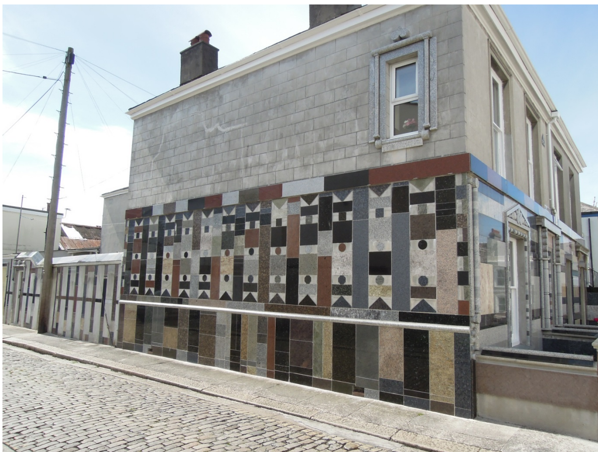
Figure 1. 73 Cecil Street, Plymouth. The house is clad in polished stone including black gabbro, salvaged by the owner over the years from washstands and kitchen worktops, cut up and affixed to the walls of his house both inside and out.
