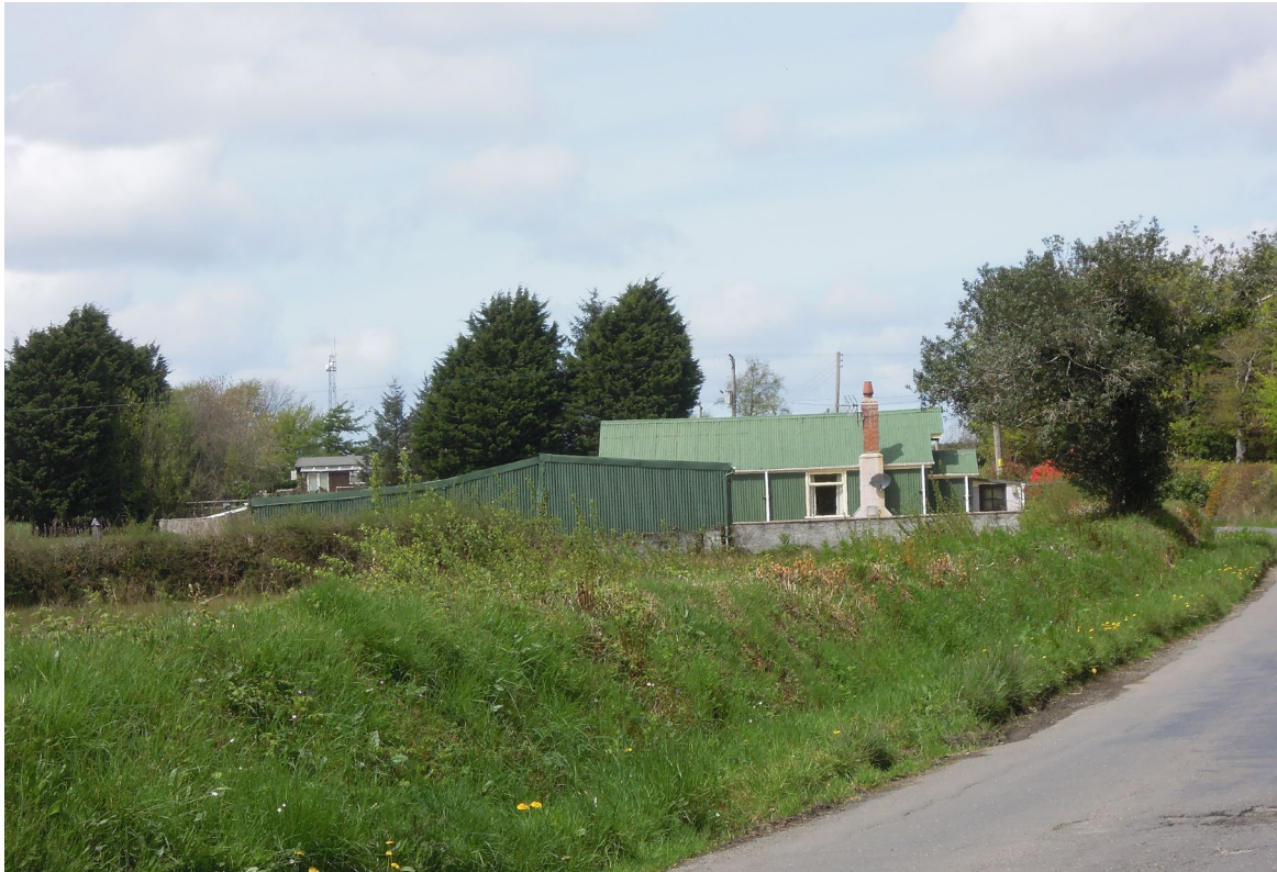
Figure 2. Sunnyside, near Broadwoodwidge. House and outbuilding clad almost entirely in corrugated iron with matching roof.
