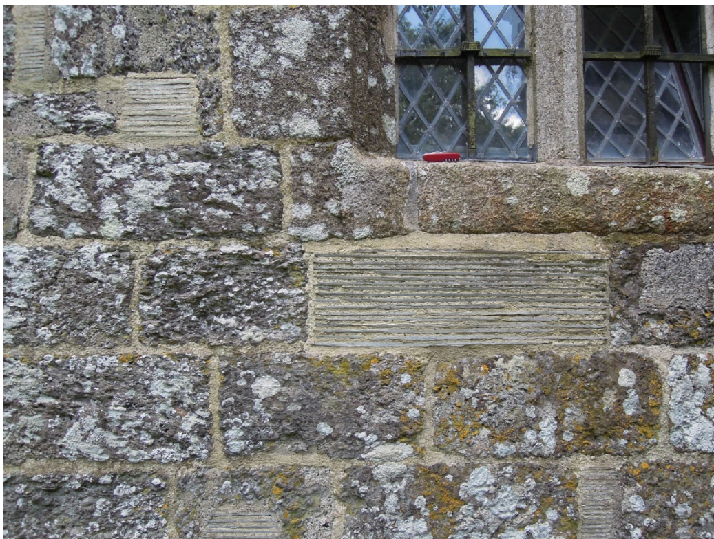
Figure 4. North side of St Nonna's church, Bradstone. Stacks of roofing slate used to replace defective building blocks. The main building stone is hornblende-chlorite slate (metavolcanics). The window dressings are of Dartmoor granite.
