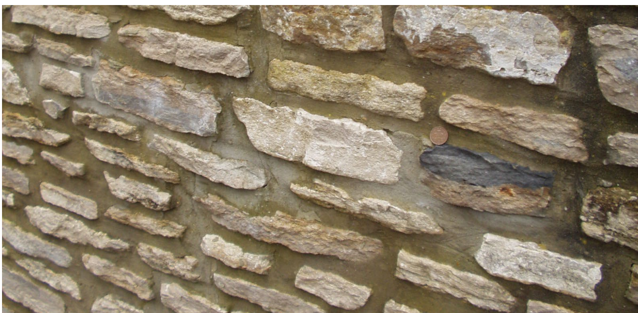
Figure 4. Thin blocks of limestone, some blue-hearted, providing a link with stone coded 19, Forest Marble. Wall on north side of road to Sockery, South Perrot.
