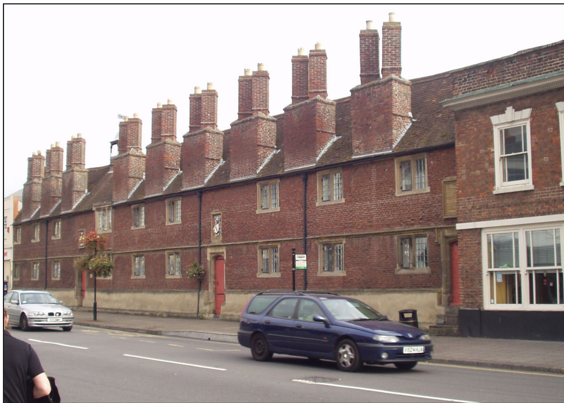
Figure 2. Grey's Almshouses, East Street, Taunton. The window dressings are of Doultling Stone. The string course, plaque and shedding course above the footing are of Ham Hill Stone.
