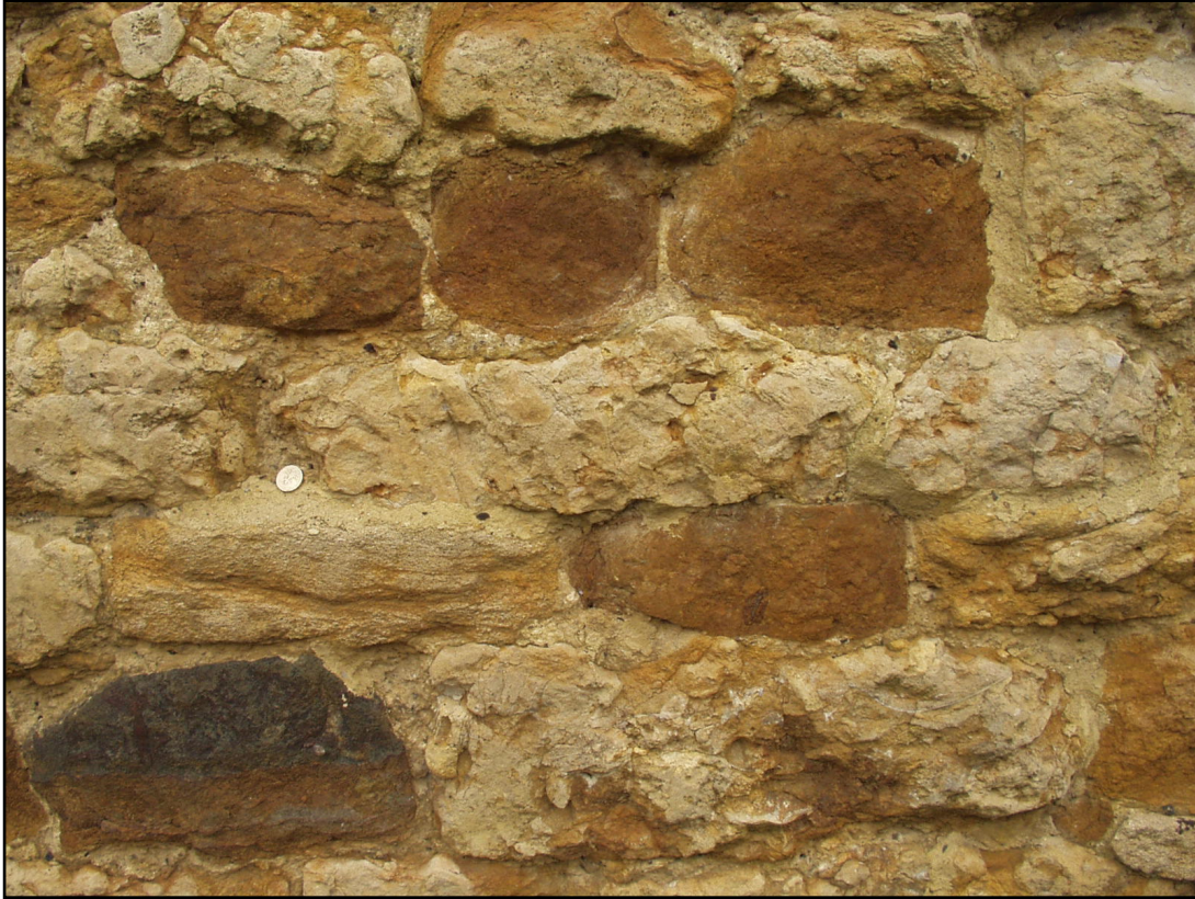
Figure 1. Garden wall, Farthings, Abbey Street, Hinton St George. The primrose yellow colour and nodular structure are typical of the Inferior Oolite limestone coded 15. The darker orange and black blocks are coded 18.
