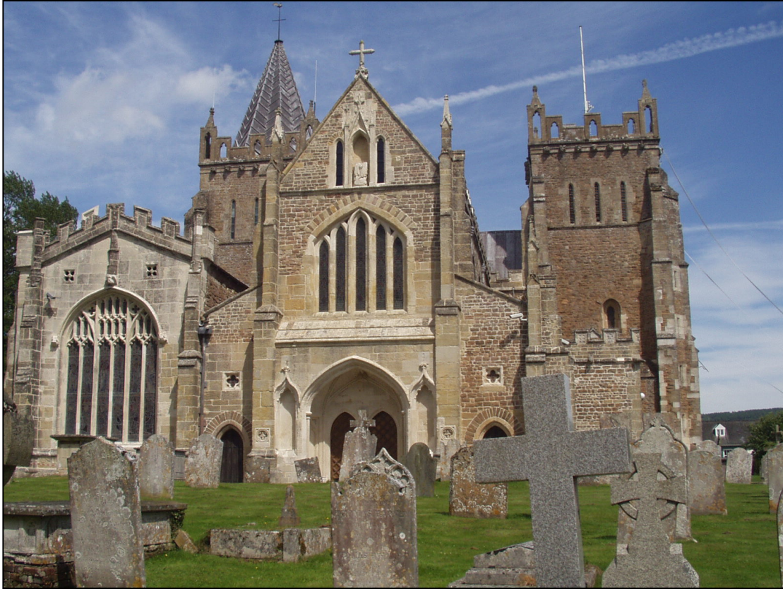
Figure 3. St Mary's, Ottery St. Mary, west end. The lower part of the wall of the nave is of Salcombe Stone ashlar. The upper part of the wall is coursed rubble, of mud pebble conglomerate from the Otter Sandstone. Note the polychrome relieving arch over the grouped lancets composed of alternating Salcombe Stone and mud pebble conglomerate from the Otter Sandstone.
