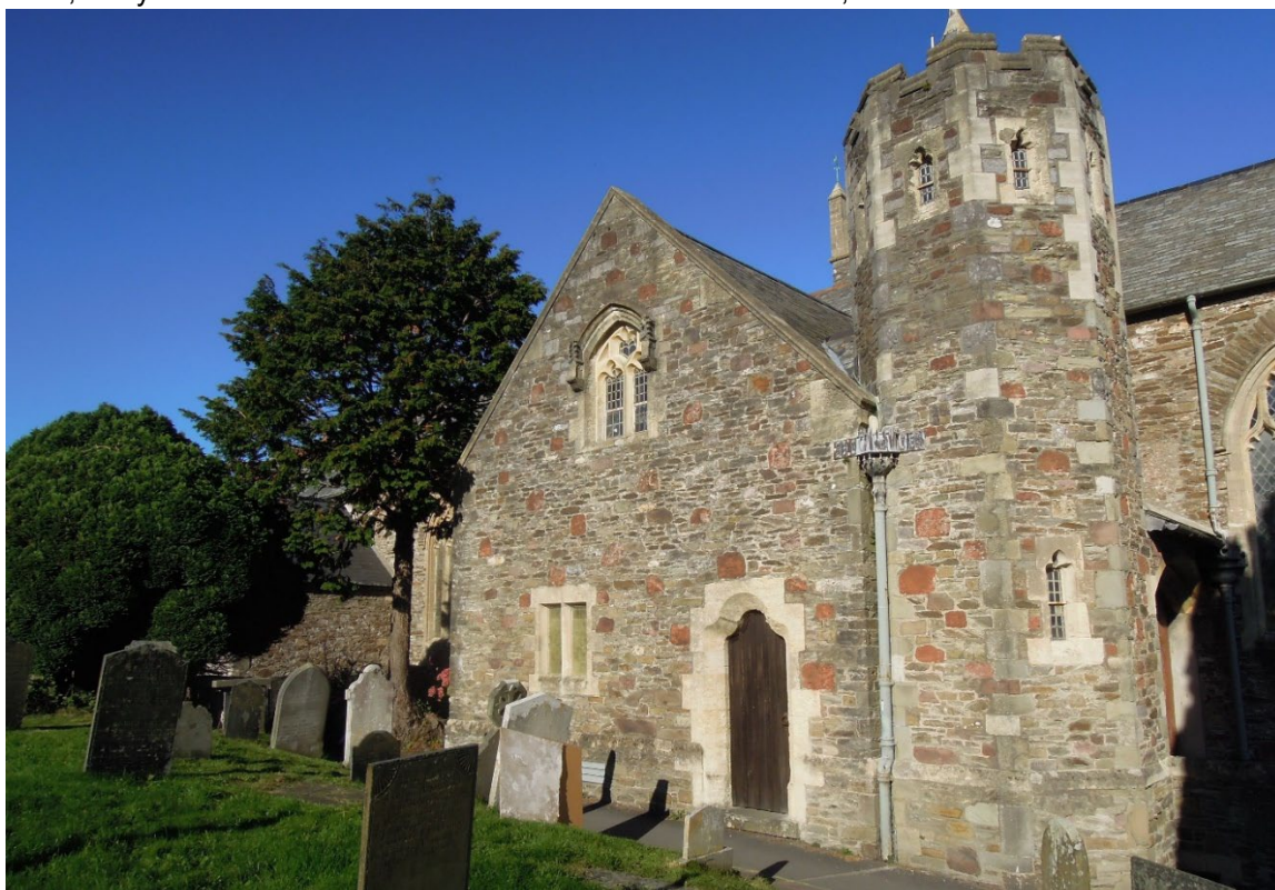
Figure 2. South side of Holy Trinity Church, Ilfracombe. Larger decorative blocks of red sandstone (Code 213) set in a mixture of grey-buff sandstone (Code 96) and slate (Code 93).
