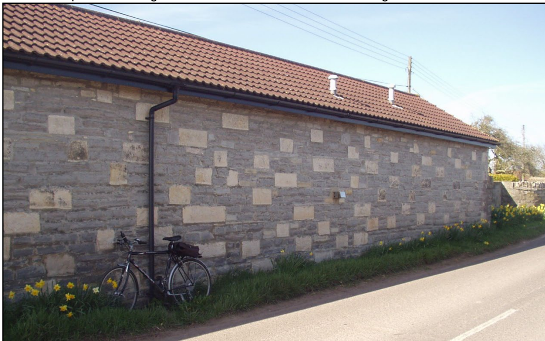
Figure 4. Outbuilding, Holly Farm, Mere Green. Decorative use of White Lias blocks spanning several courses of Blue Lias limestone.
