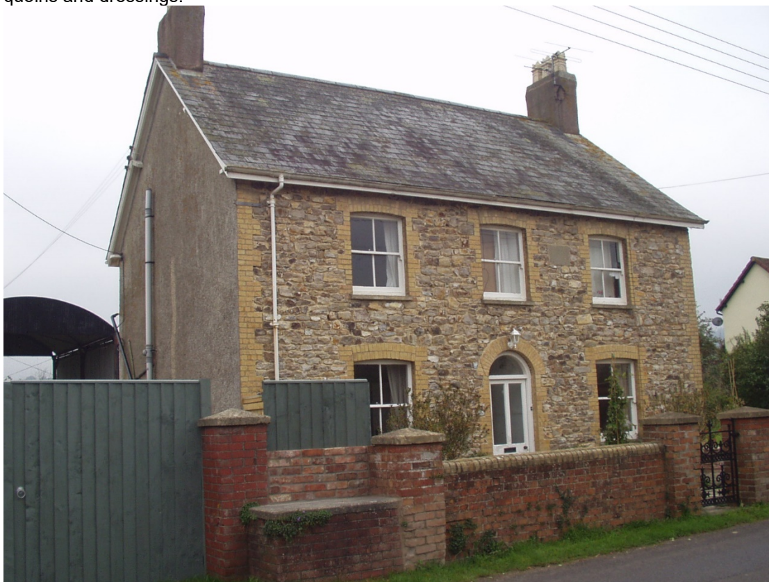
Figure 14. Typical C19 house of chert rubble with brick quoins and dressings and rendered gable end. Sellick's Green, Blagdon Hill.
