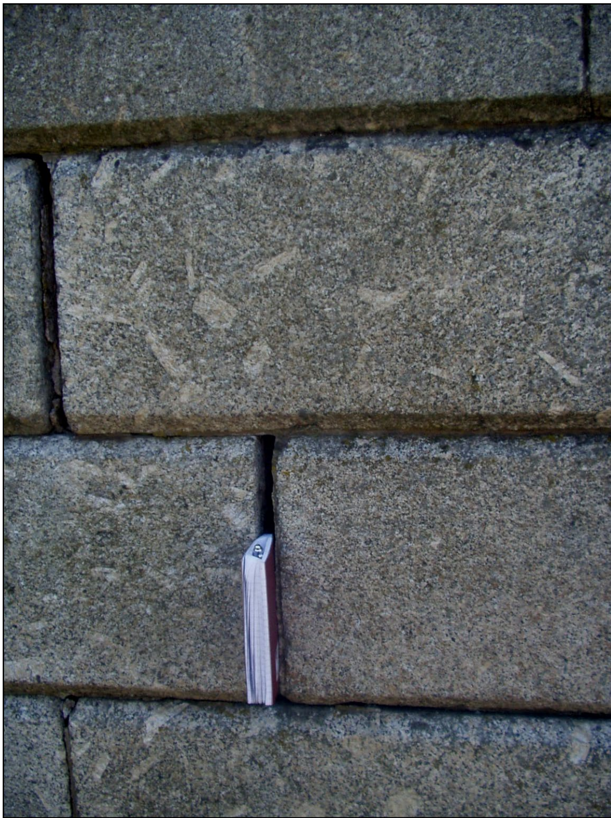
Figure 10. Entrance gateway to Teignmouth Castle. The granite contains alkali feldspar phenocrysts with more-or-less random orientation.
