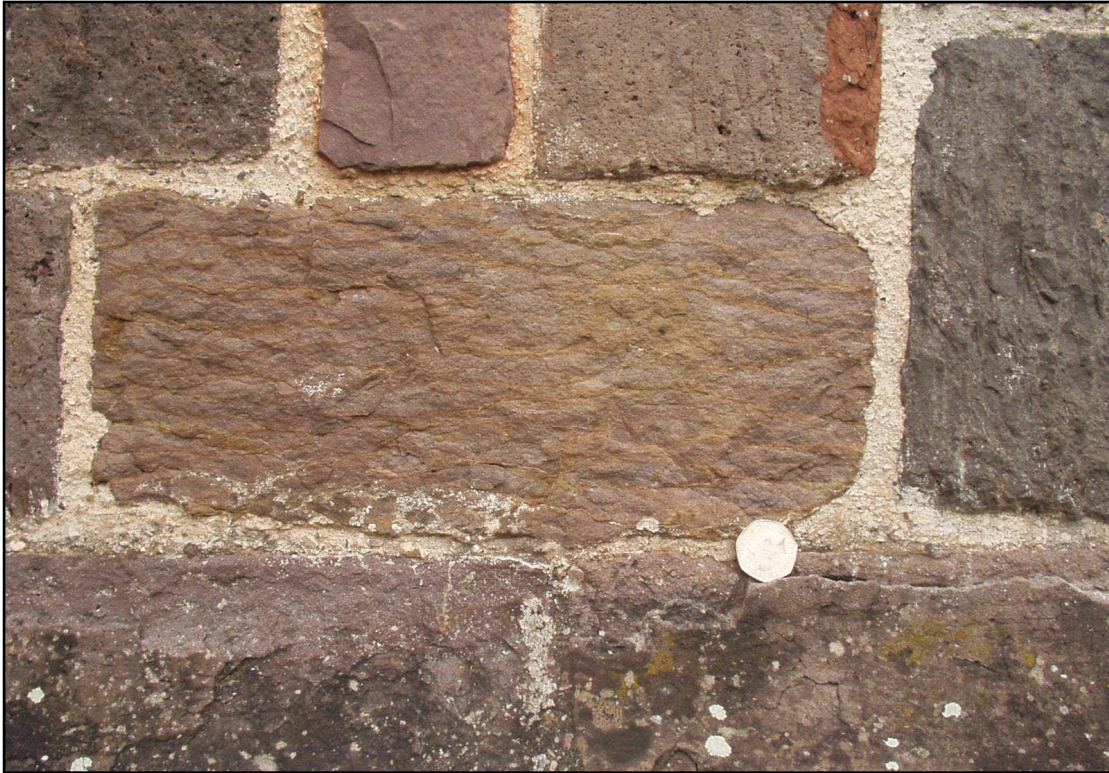
Figure 2. South aisle, St Mary's church, Whimble. All the blocks in the photograph are of lava, mainly lacking obvious vesicles and showing a range of textures and colours.
