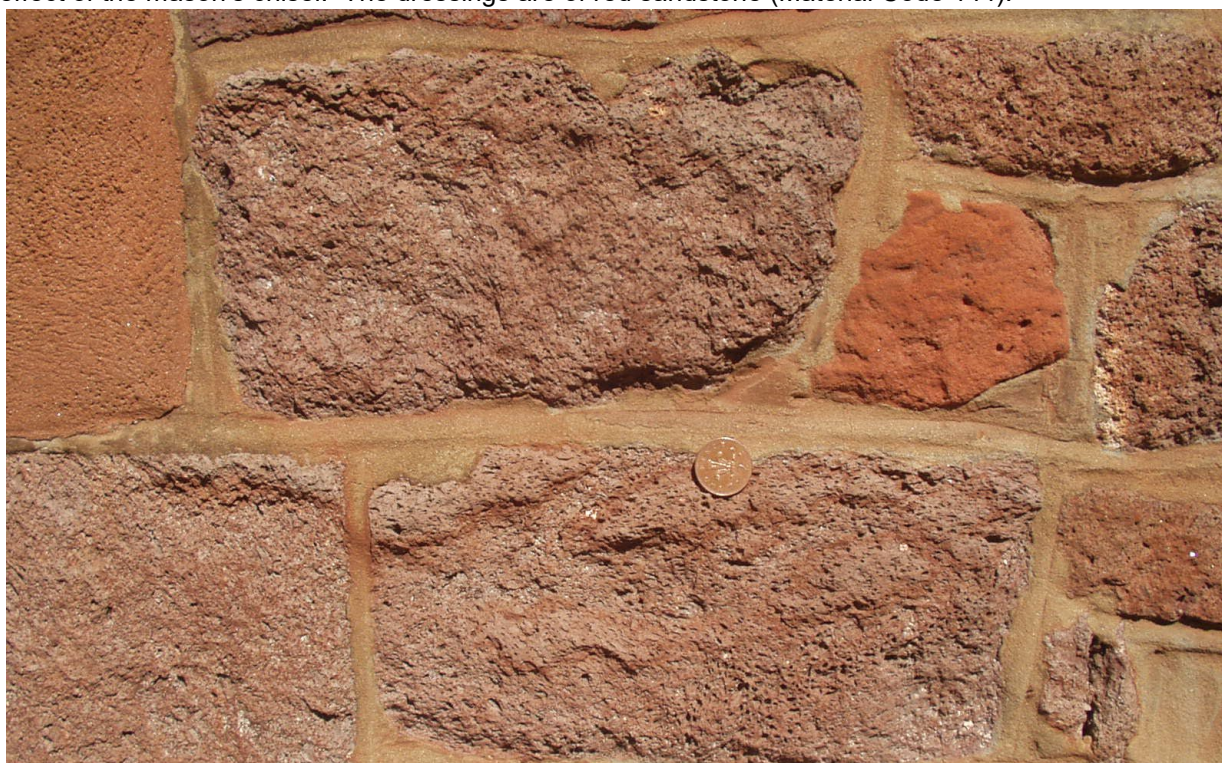
Figure 3. Chapter House of the Church of the Holy Cross, Crediton. The main building stone is pink Exeter volcanics from Posbury Clump with one smaller piece of red sandstone towards the right. The block of smooth stone top left is a skimming of artificial material designed to repair the original stonework and to mimic the volcanics. The repairs were applied in Victorian times and were not successful since water got in behind them and the skimmings spalled off.
