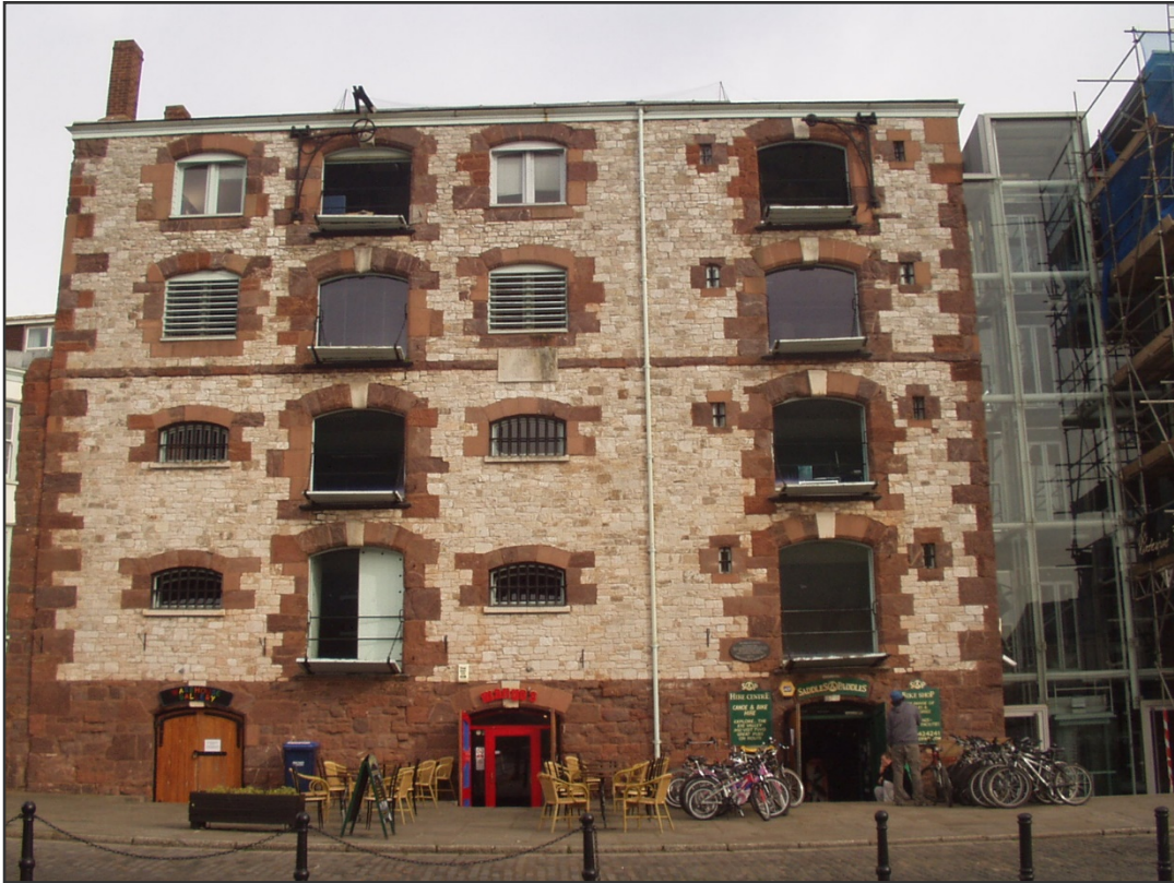
Figure 3. The Bike Shop, The Quay, Exeter. Pale grey limestone over Pocombe Stone footing with Pocombe Stone and red sandstone quoins and dressings.
