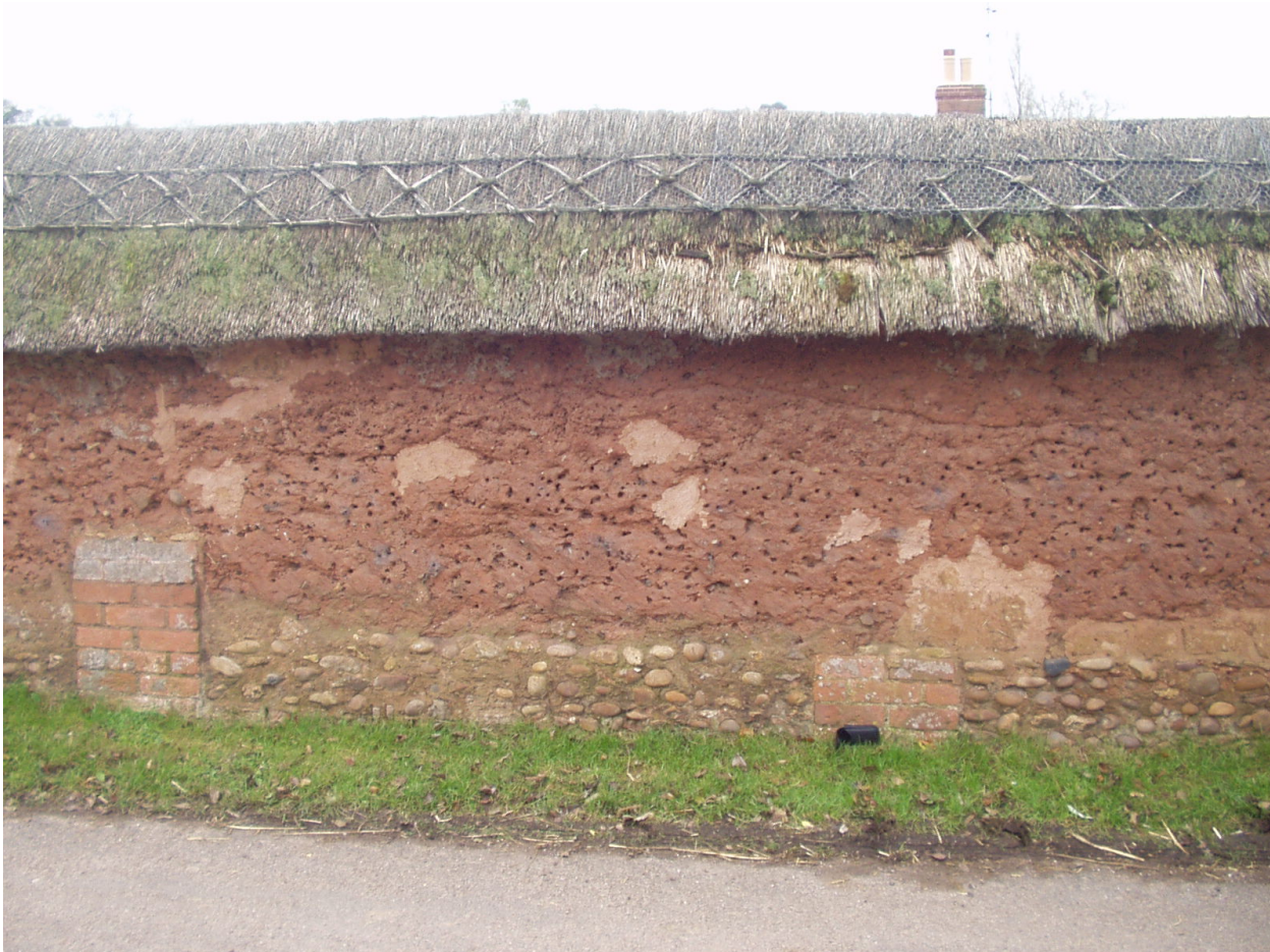
Figure 1. Place Court, Colaton Raleigh. The wall is of cob full of the burrows of solitary bees, on a footing of “Budleigh Buns”.
