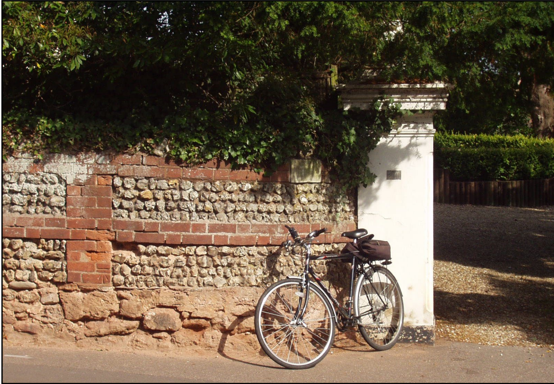
Figure 2. The Old Vicarage, West Hill, Budleigh Salterton. Red conglomerate and sandstone from the Otter Sandstone below, flint in brick panels above.
