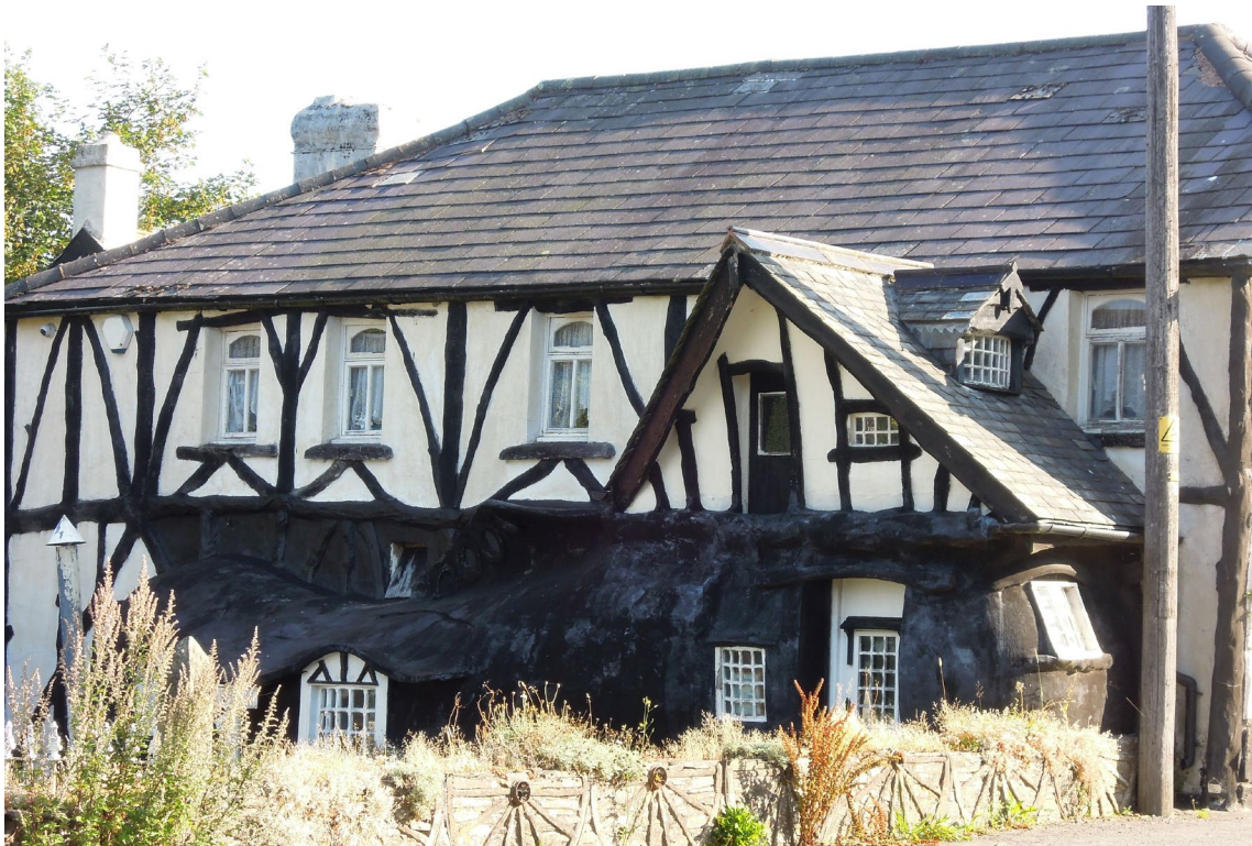
Figure 8. Annex to the Highwayman Inn, Sourton. I think this must be spoof timber framing.
