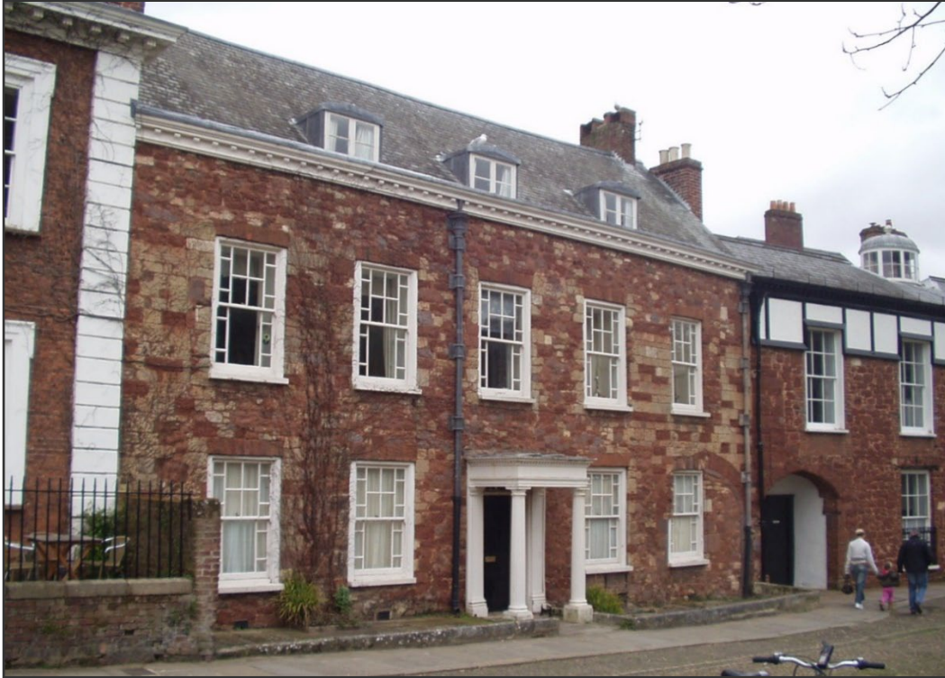
Figure 8. 6 Cathedral Close, Exeter. The Georgian front wall including the dressings is a mixture of red Heavitree Breccia, purple Exeter volcanics and brown Salcombe Stone.
