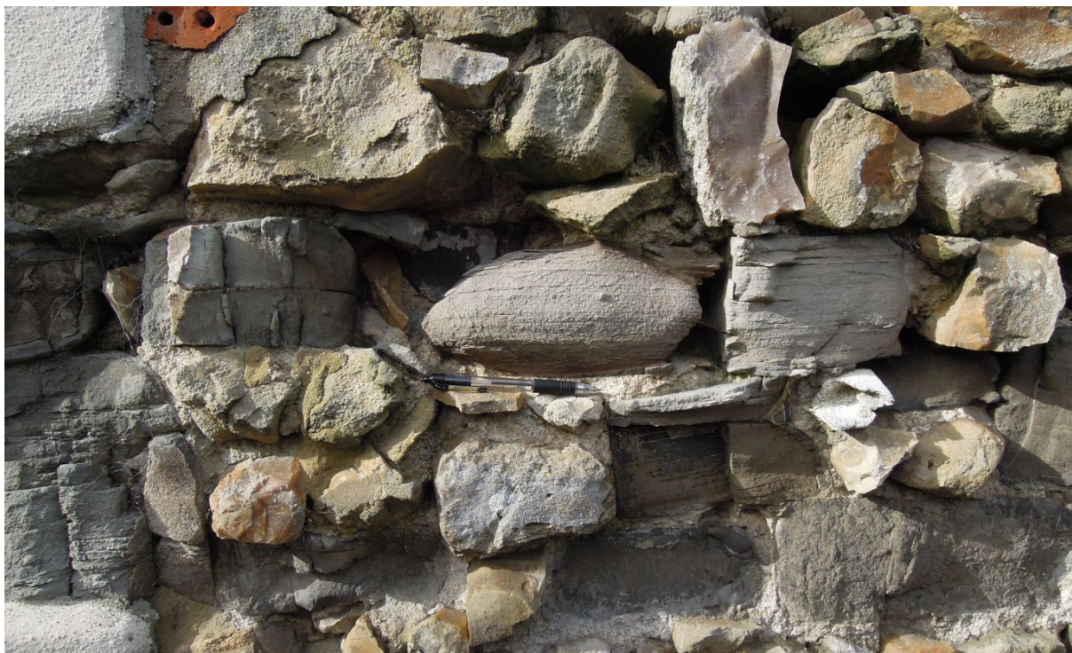
Figure 1. Rounded cobble of grey marly siltstone (centre) along with Blue Lias limestone, and Upper Greensand chert and sandstone. Wall in Devonedge Lane, Charmouth.
