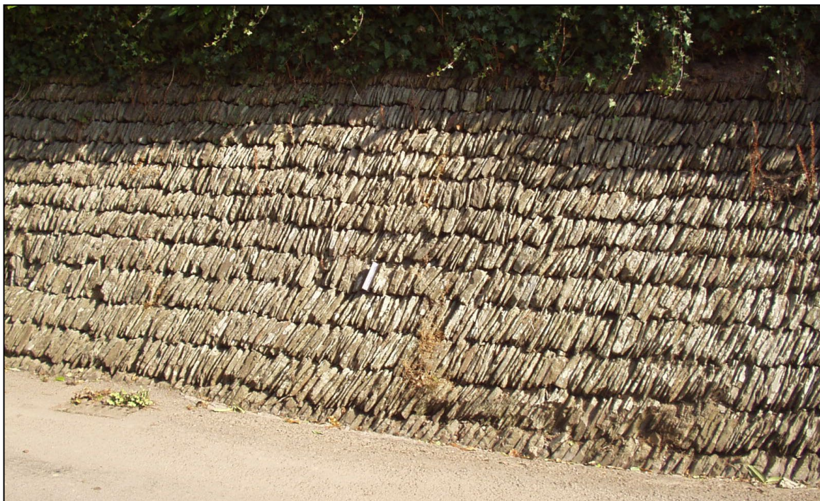
Figure 4. Roadside wall, Langley Marsh. Strongly and regularly cleaved slate from Oakhampton Quarry.
