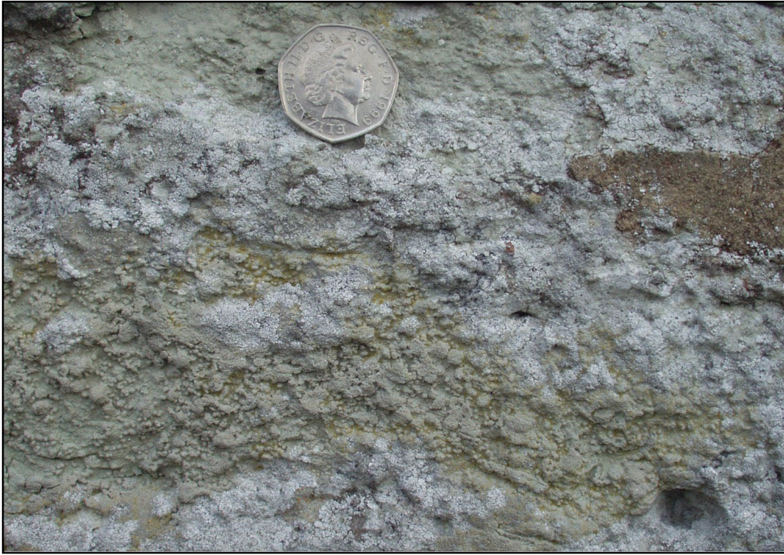
Figure 4. Tower of St Nicholas' church, Combe Raleigh. "droplet" texture developed on the surface of a block of green sandstone with sparse disseminated glauconite.
