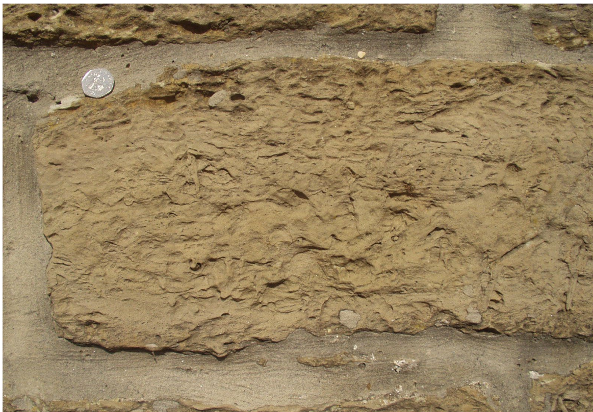
Figure 4. Wall behind the beach, West Bay. Yellow sandstone that can be matched with the sandstone forming the adjacent cliff.
