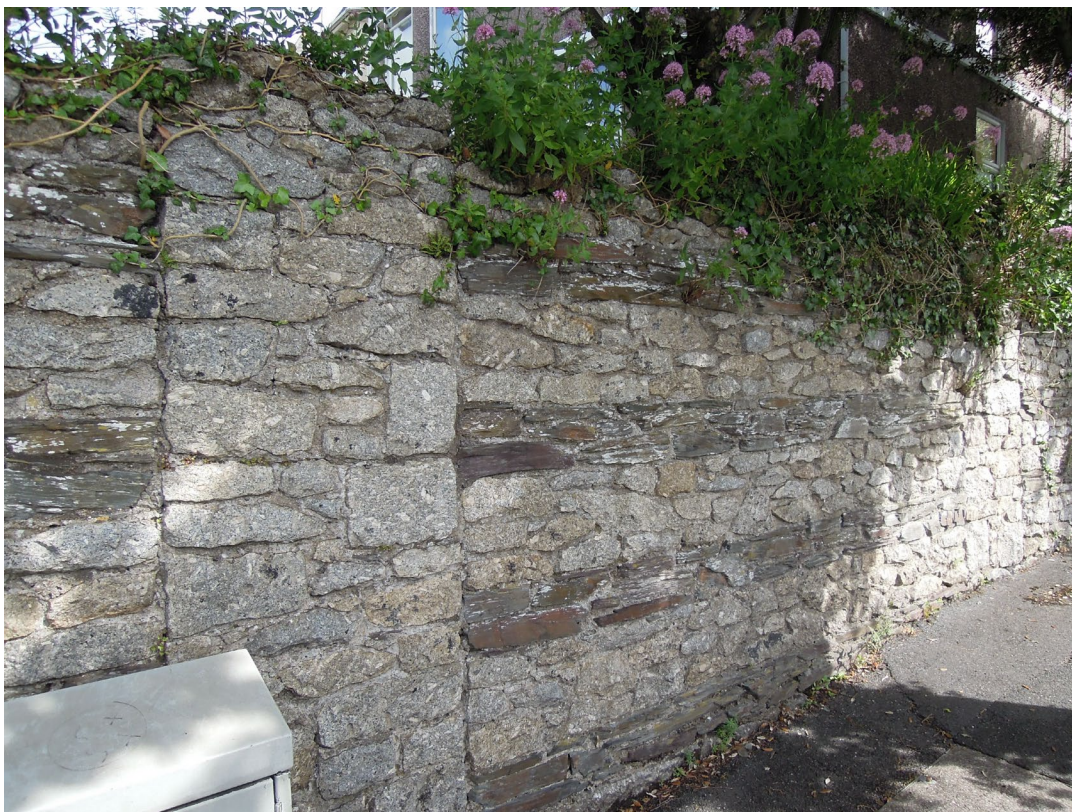
Figure 14. Roadside wall with alternating courses of granite and dark slate. East side of Alma Road, Pennycomequick, Plymouth.
