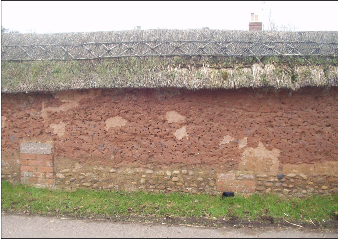
Figure 2. Place Court, Colaton Raleigh. Boundary wall of cob with footing of Budleigh Salterton pebbles and coping of thatch. The cob is riddled with the burrows of solitary bees.
