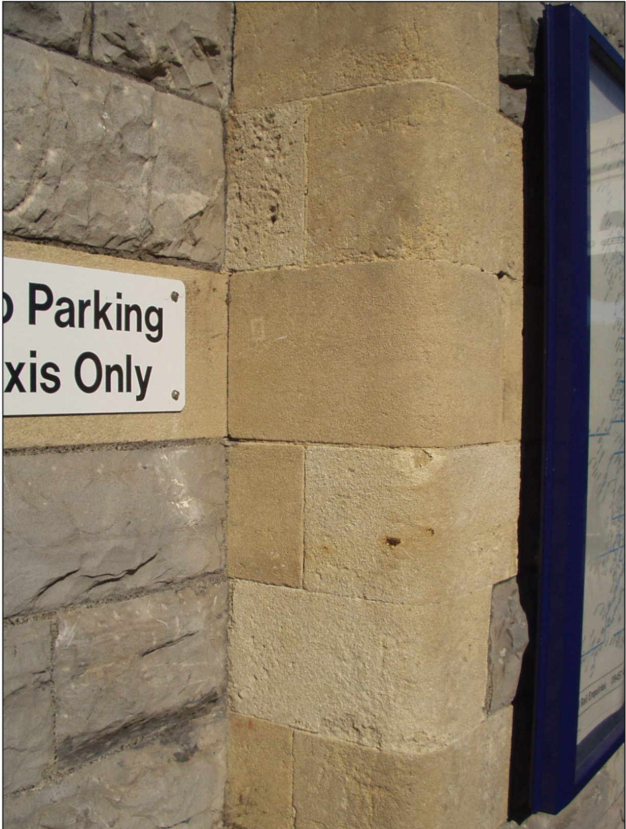
Figure 4. Torquay railway station. The paler of the two kinds of stone used for the dressings is Bath Stone; the darker and better preserved is Douling Stone.
