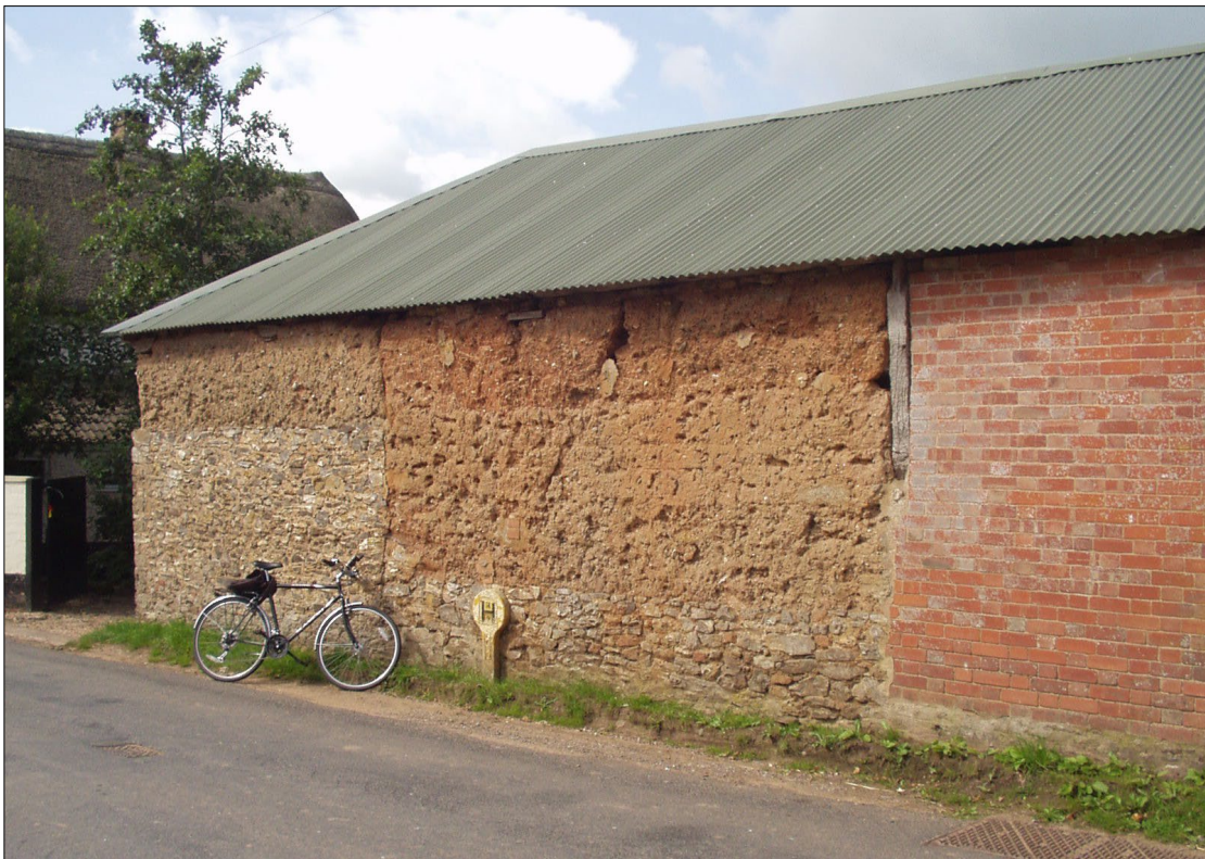
Figure 3. Salter's Farm, Luton. Lower parts of the cob walls are of chert.
