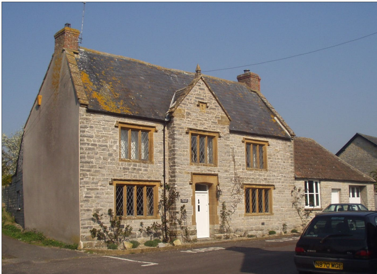
Figure 1. Peace Lane Cottage, Long Sutton. Ham Hill Stone dressings round door and windows. The front wall is of Blue Lias limestone.
