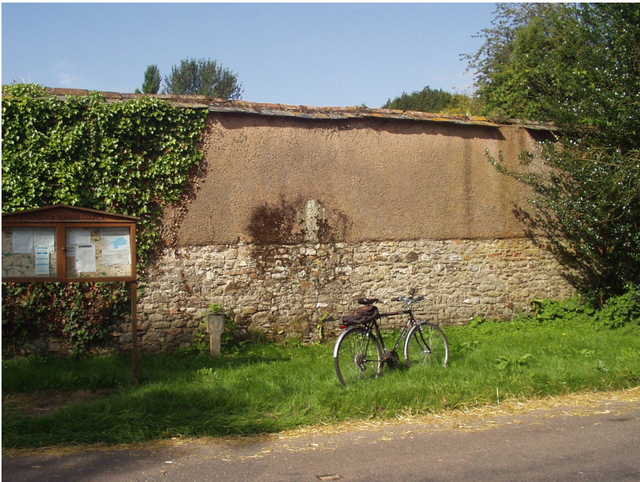
Figure 1. Slate coping to wall of rendered cob on a deep stone rubble footing. Wall behind village notice board, Payhembury.
