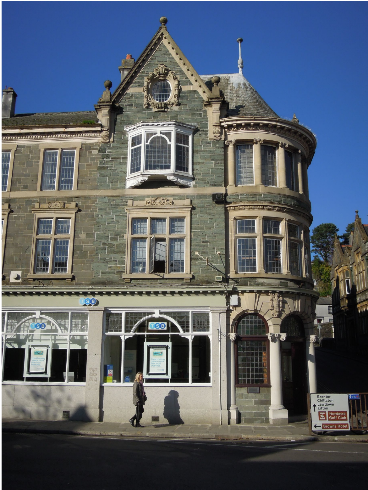
Figure 7. Trustees Savings Bank, Tavistock. The building is mainly of Hurdwick Stone but with dressings of Portland Stone for the pillars on the ground floor and of Douling Stone (yellowish) for the dressings on the upper floors.
