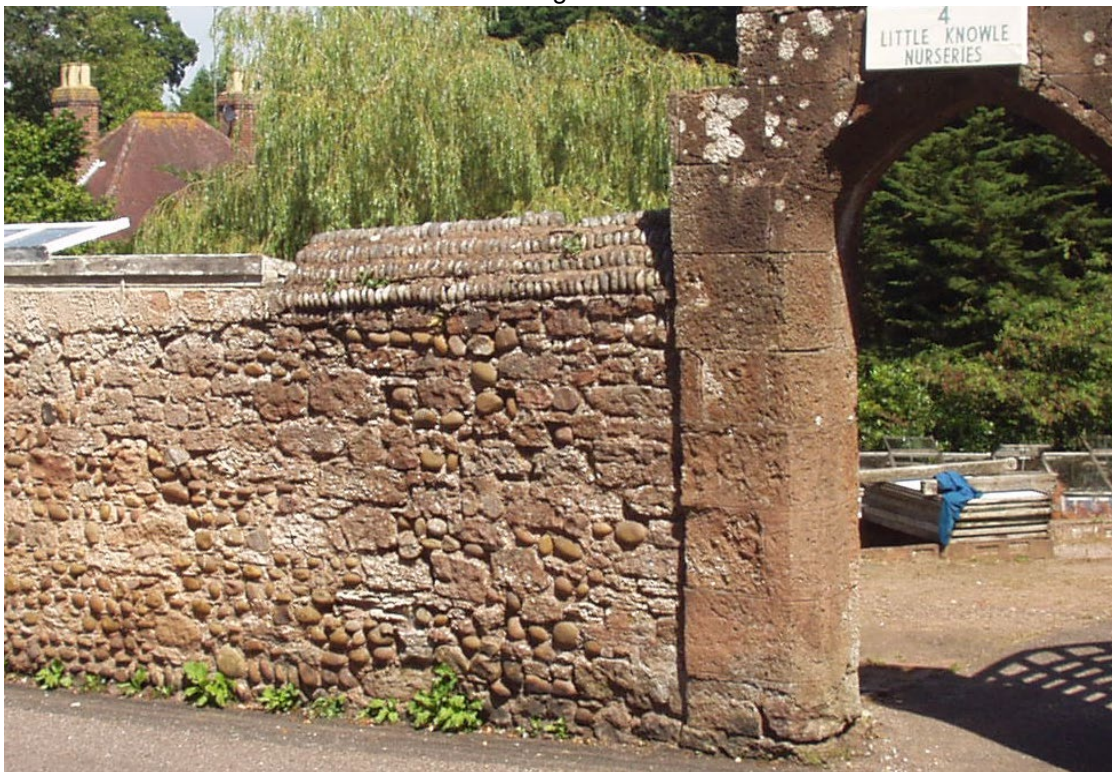
Figure 3. Little Knowle (east side), Budleigh Salterton. The wall is of mixed “Budleigh buns” and mud-flake conglomerate from the Otter Sandstone. The coping is of carefully sized quartzite pebbles and the gateway of mud-flake conglomerate from the Otter Sandstone.
