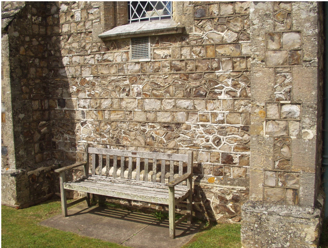
Figure 11. Church of St. Philip and St. James, Escot. Alternating courses of squared and random-rubble chert blocks. The cornerstones of the buttresses are of calcareous sandstone from the Upper Greensand.
