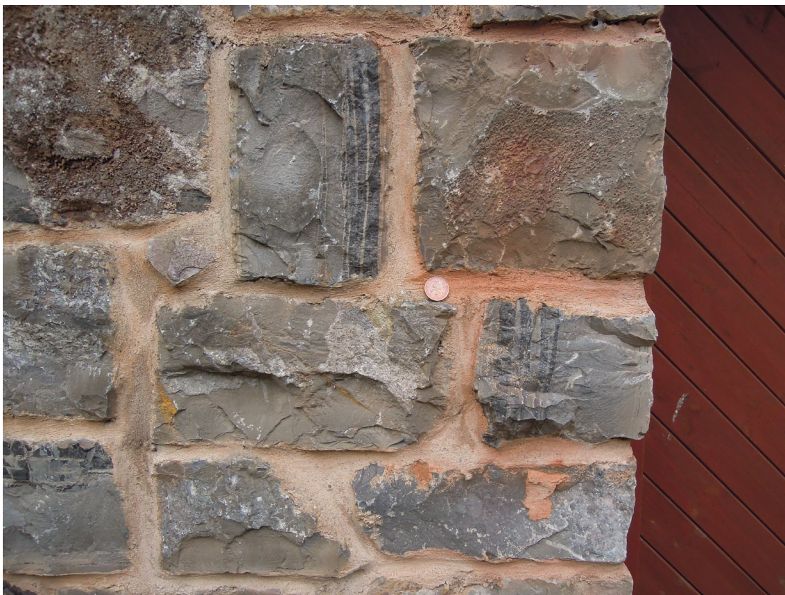
Figure 3. Grey fine-grained limestone with black chert bands, outbuilding, Upcott, Somerset.
