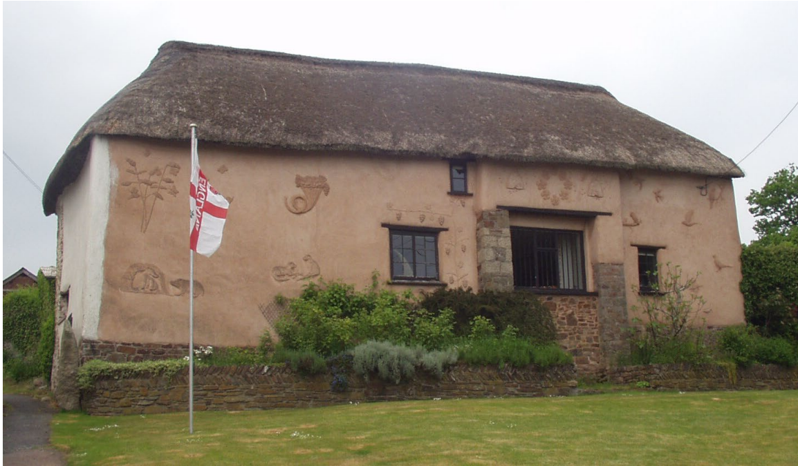
Figure 5. Decorated cob cottage on a footing of sandstone from the Crackington Formation. Chapple Lane, Sampford Courtenay.
