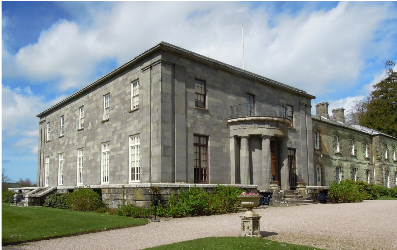
Figure 11. Arlington Court. This wing is composed of purple and green Pickwell Down Sandstone ashlar.
