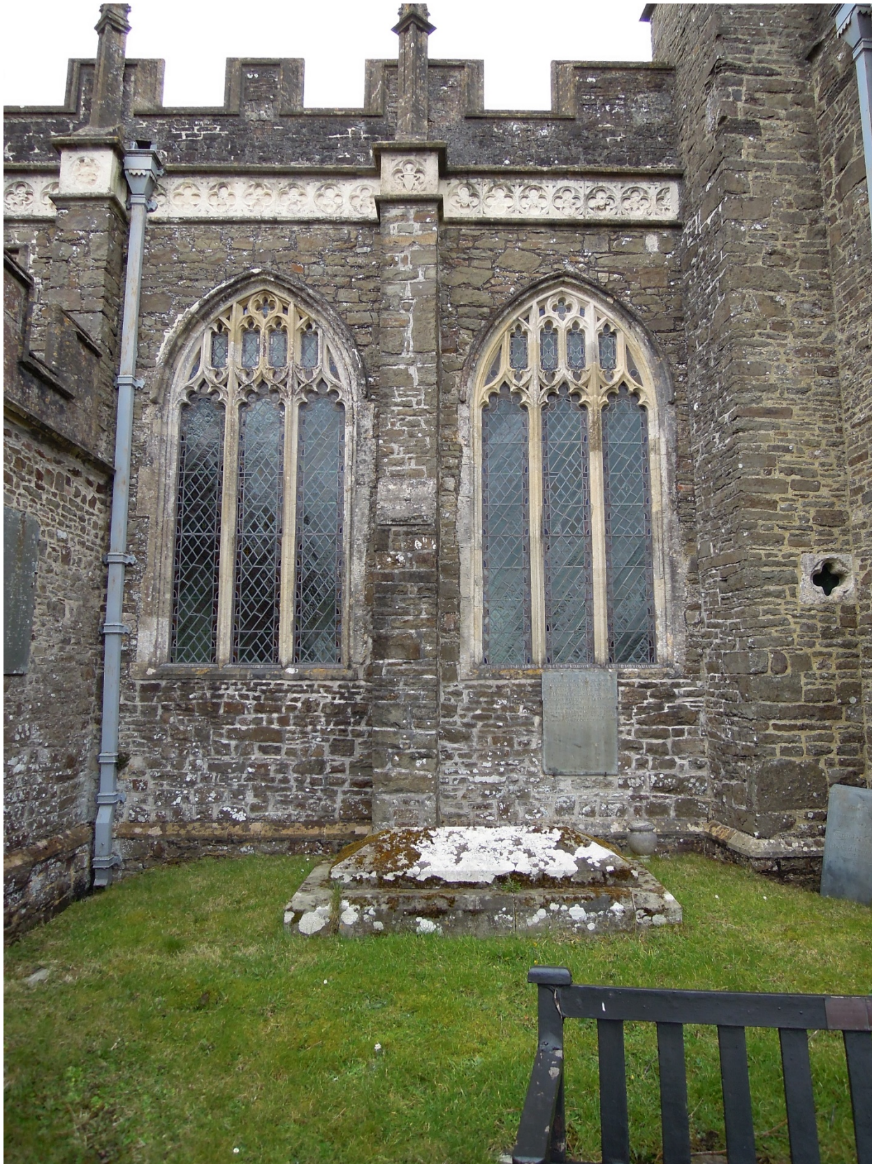
Figure 3. South aisle windows of Beer Stone with carved Beer Stone frieze over. Church of St Hieritha, Chittlehampton. The walls are made of Bude Formation sandstone.
