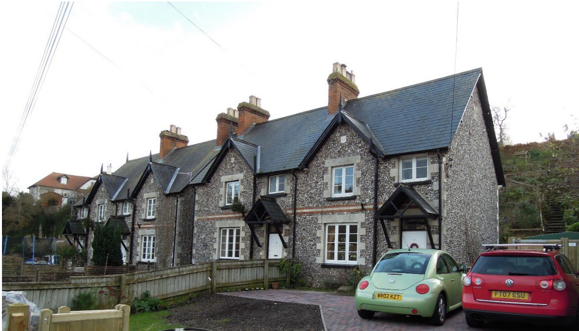
Figure 6. Jubilee Cottages, The Causeway, Beer. The walls are finished with flint. The quoins and dressings are of Beer Stone with decorative brick string course.
