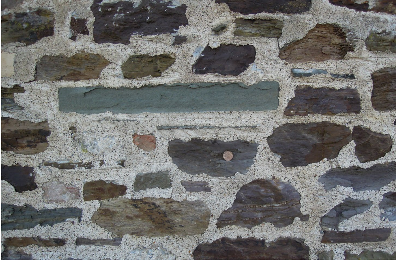
Figure 8. Variegated sandstone, garden wall of Myrtle Cottage, 1.5km south of Fremington.
