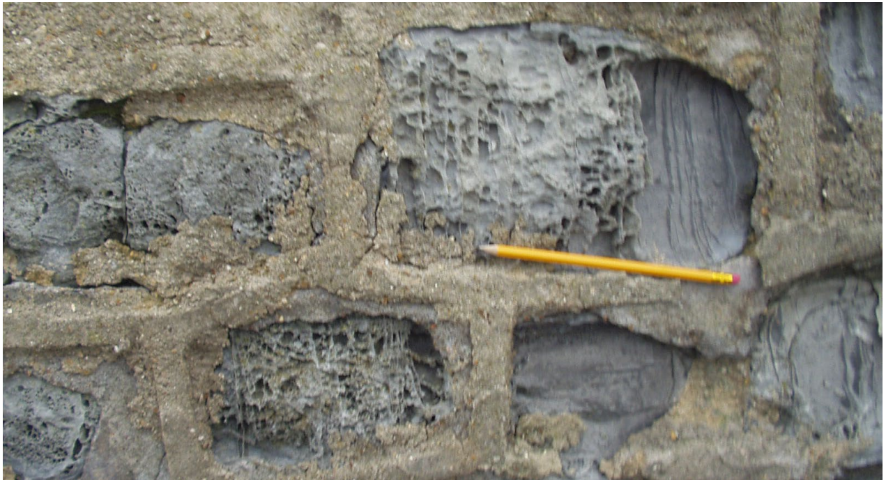
Figure 16. Former sea wall below the Marine Theatre, Lyme Regis. Erosion has washed out the soft limestone leaving stringers of calcite standing proud.
