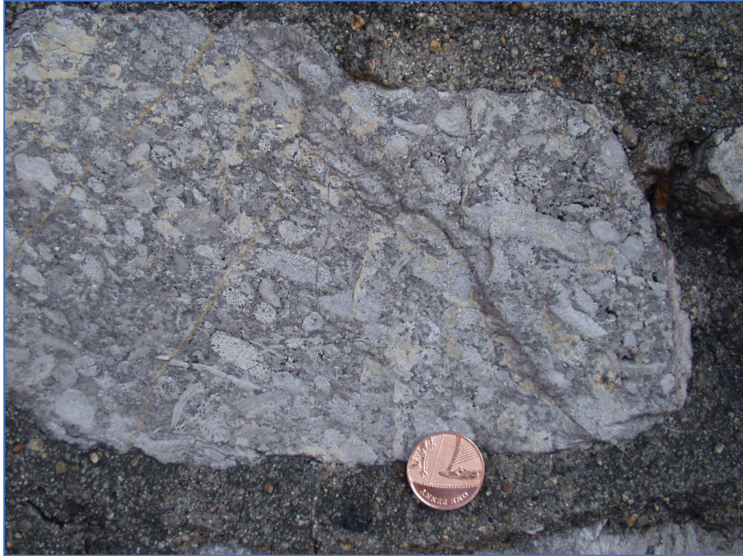
Figure 7. Block of coarse-grained pale-grey limestone composed mainly of coral fragments, garden wall, Westhill Road, Torquay.
