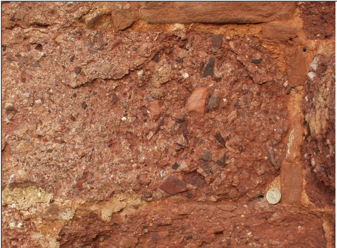
Figure 2. Red breccia, St Michael's church, Clyst Honiton. Note the use of thin sandstone blocks to compensate for the rather rounded outlines of the breccia blocks.
