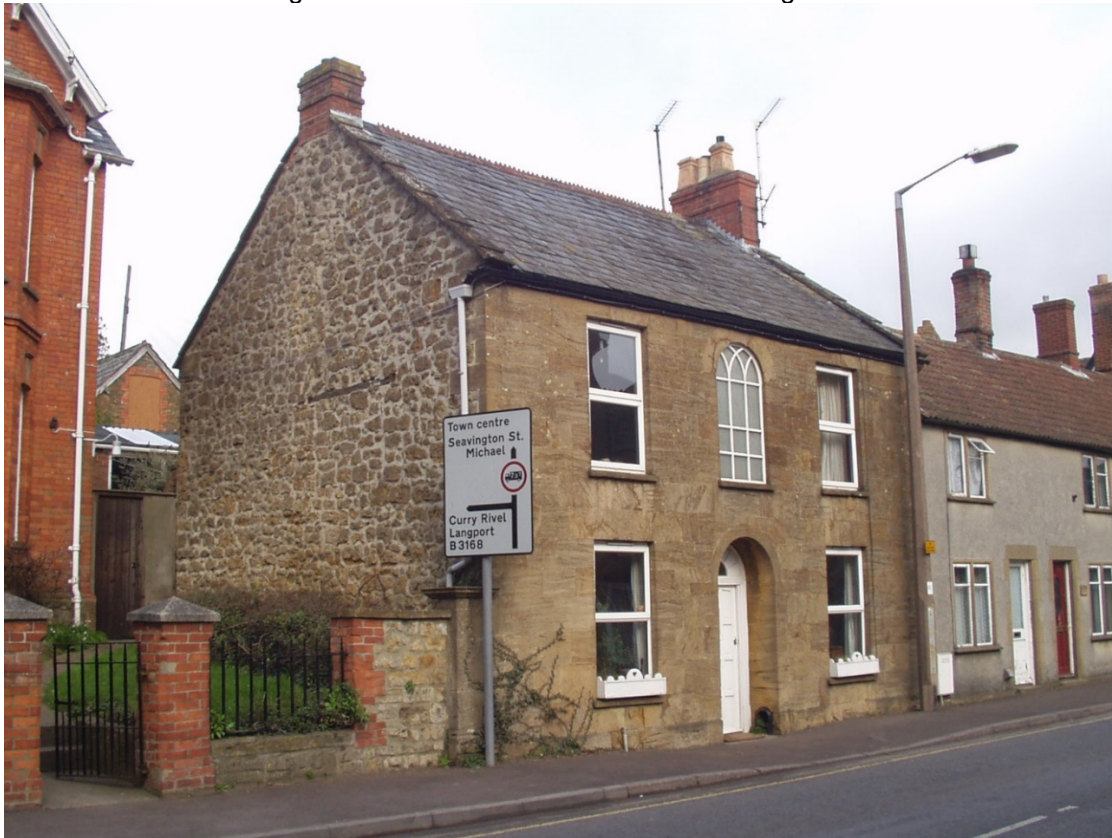
Figure 8. 8 Station Road, Ilminster. The front wall is of Ham Hill Stone ashlar. The side wall is of Moolham Stone rubble.
