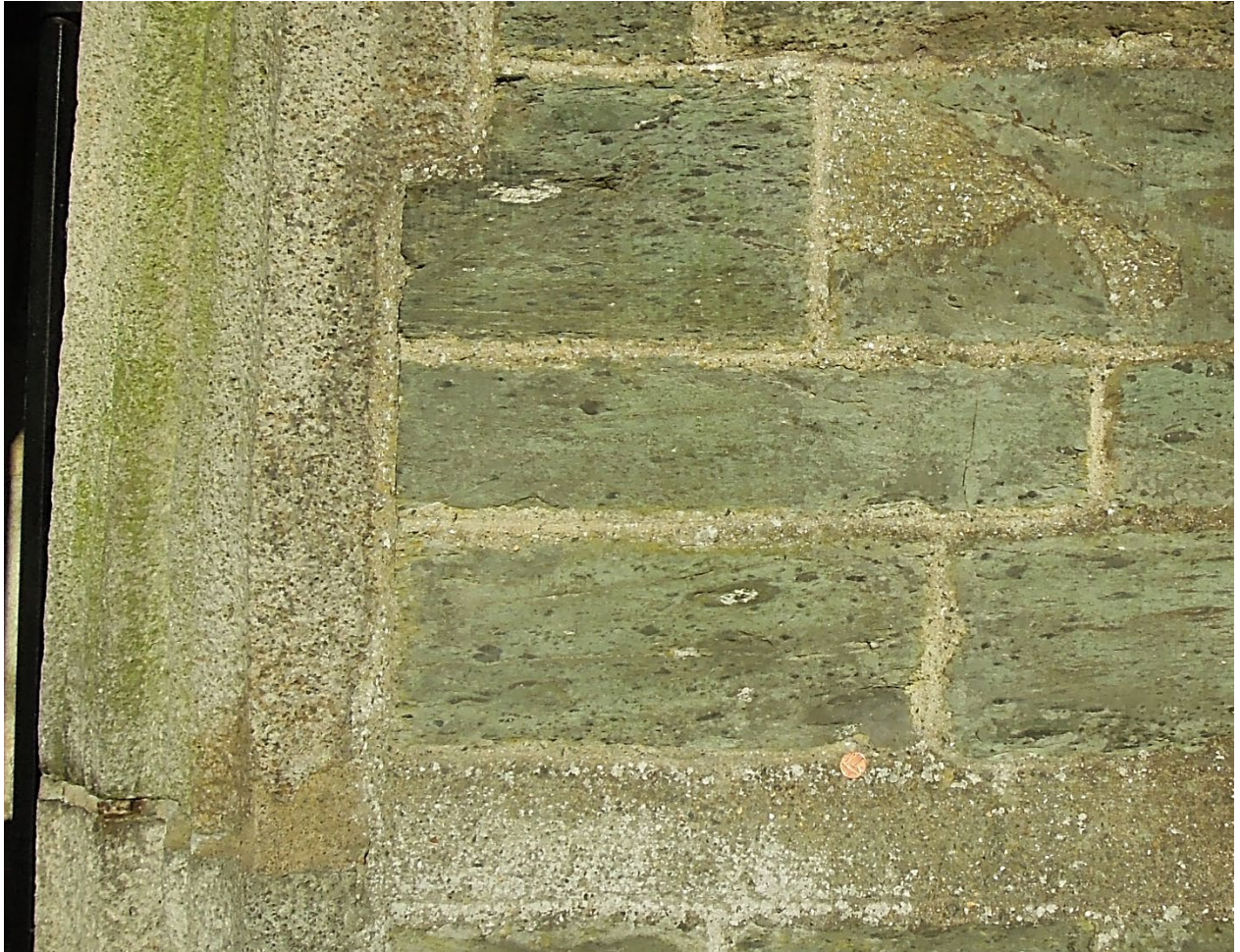
Figure 1. South porch of St Eustacius' church, Tavistock. The green Hurdwick Stone of the walling is repaired with neutral artificial stone resembling concrete more than the Hurdwick Stone. The jamb on the left is of Roborough Stone.
