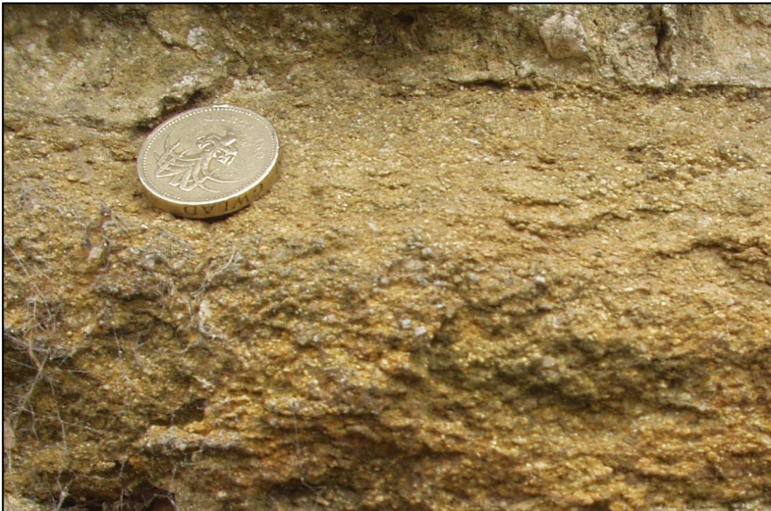
Figure 2. Garden wall, Farthings, Abbey Street, Hinton St George. Detail of homogeneous block showing disseminated coarse grains of paler calcite, probably crinoid ossicles.
