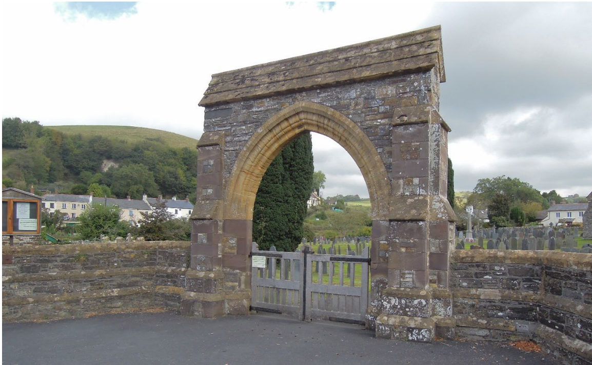
Figure 6. Gateway to the churchyard of St James' church, Swimbridge. The upper part of the archway and the string courses and coping of the flanking walls are of Ham Hill Stone.
