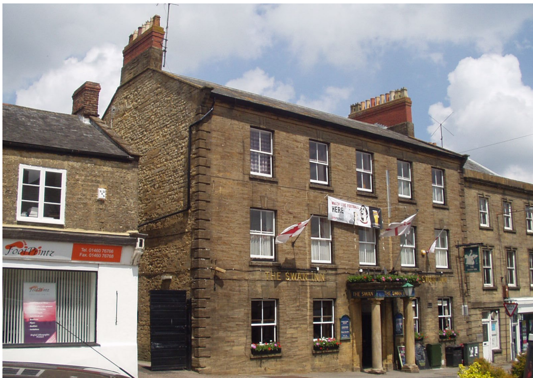
Figure 7. The Swan Inn, Church Street, Crewkerne. The gable end is of Inferior Oolite coursed rubble; the front façade is of Ham Hill Stone ashlar, a common arrangement in West Dorset and South Somerset.
