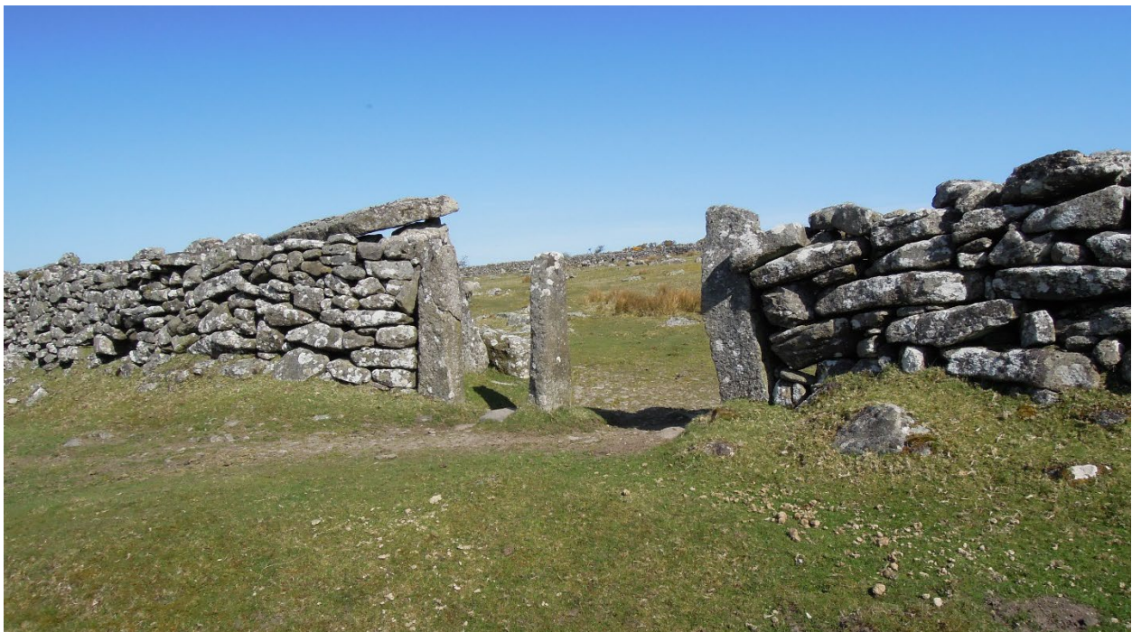
Figure 15. Monolith granite gateposts, Two Bridges, Dartmoor.
