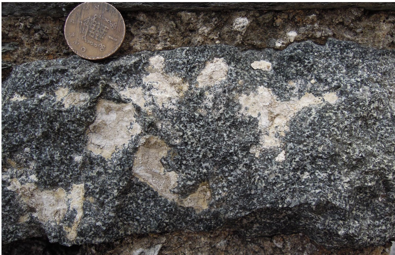
Figure 7. Amphibolite with adhering patches of pale plaster. Outbuilding, Roman Way, Plymouth.
