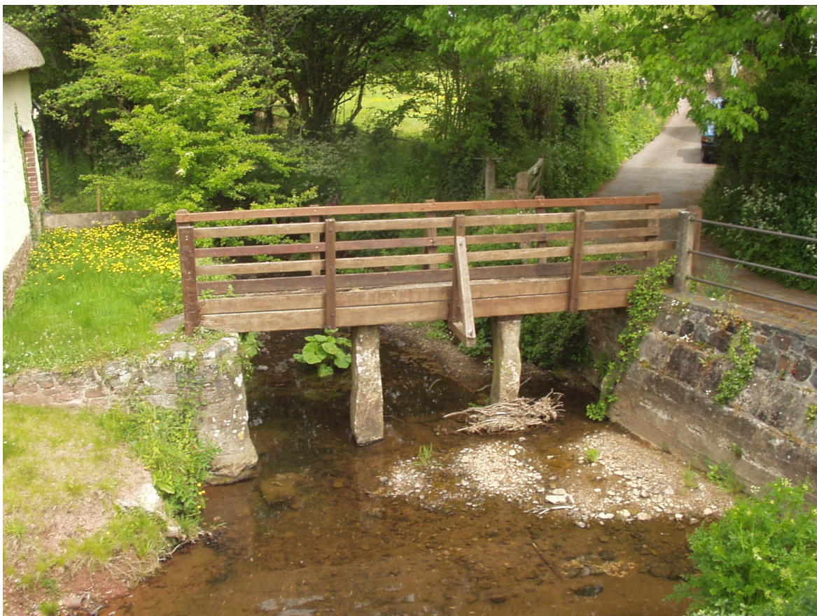
Figure 17. Wooden footbridge set on granite monolith uprights. Sampford Courtenay.
