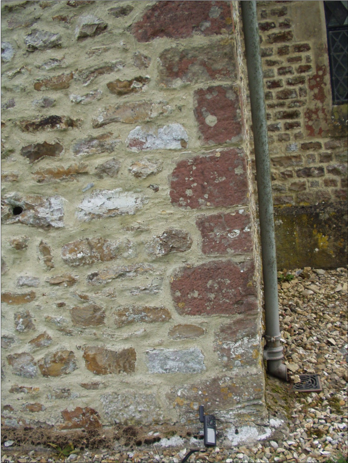
Figure 4. Tower of St Cuthbert's, Widworthy. Wall of chert rubble with quoins of calcareous sandstone showing the growth of characteristic crimson algae.
