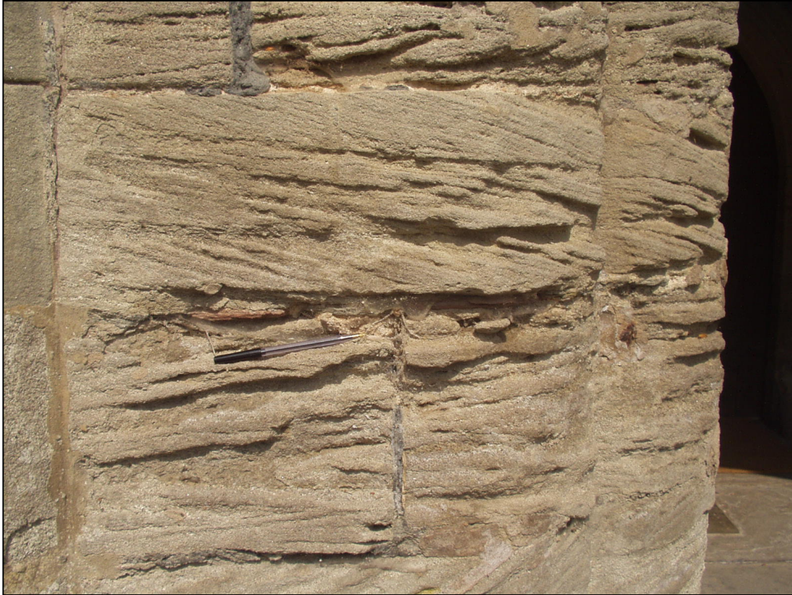
Figure 5. St Giles' church, Bradford-on-Tone. Cross-bedded North Curry Sandstone. Once again, the blocks have been laid upside-down.
