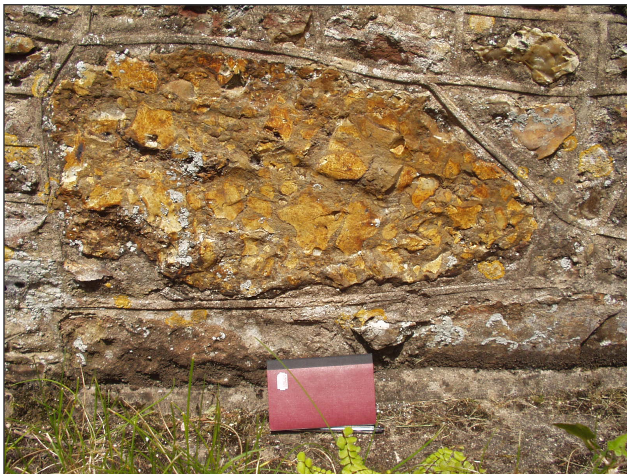
Figure 1. Block of chert breccia in the footing of St Gregory's church, Harpford. The yellow or toffee colour of the chert fragments is characteristic.
