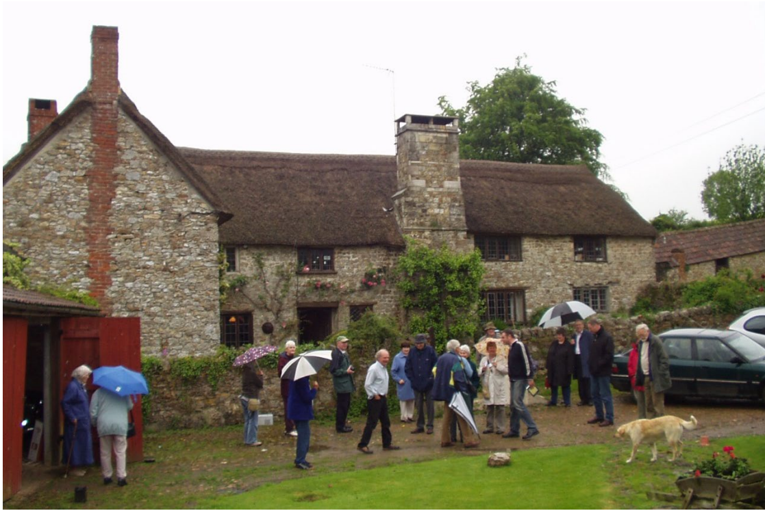
Figure 3. Poltimore Farm, Farway (C15), almost all of chert rubble with minor cob and timber framing. The cross wing on the left with brick-lined flue is Victorian.
