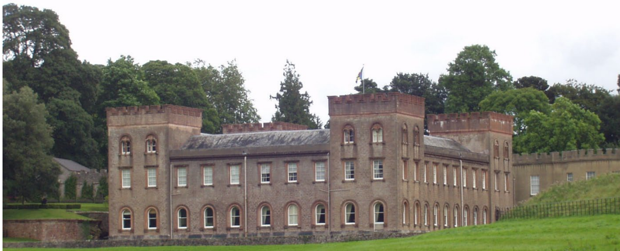
Figure 2. West elevation of Ugbrooke House. The artificial stone of which the west wall is made has been marked out with outlines to look like snecked construction and the material resembles Ugbrooke Sandstone of which the rest of the house is constructed. Each “stone” has been finished so as to mimic the effect of the mason’s chisel. The dressings are of red sandstone (Material Code 144).
