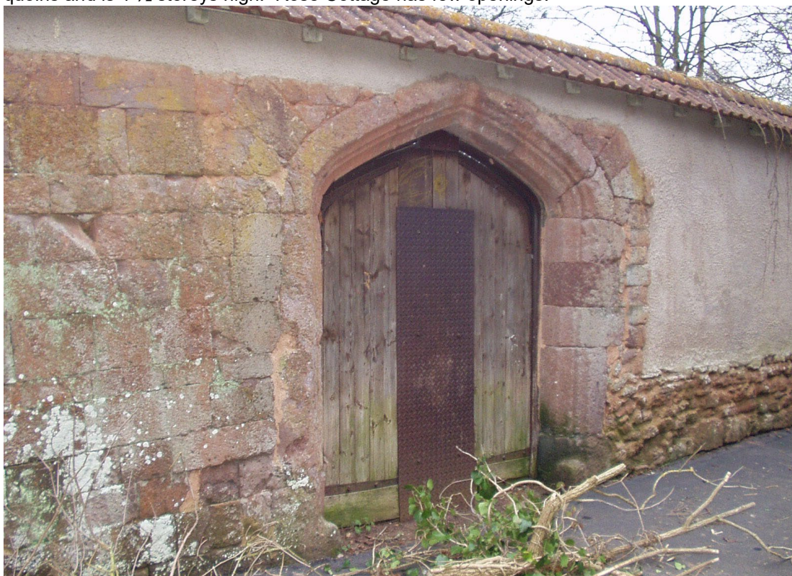
Figure 8. Entrance to Polsloe Priory precinct, Exeter. Rendered cob on a footing of red breccia, red sandstone and Exeter volcanics with new tile coping. The dressings round the door are of Exeter volcanics.
