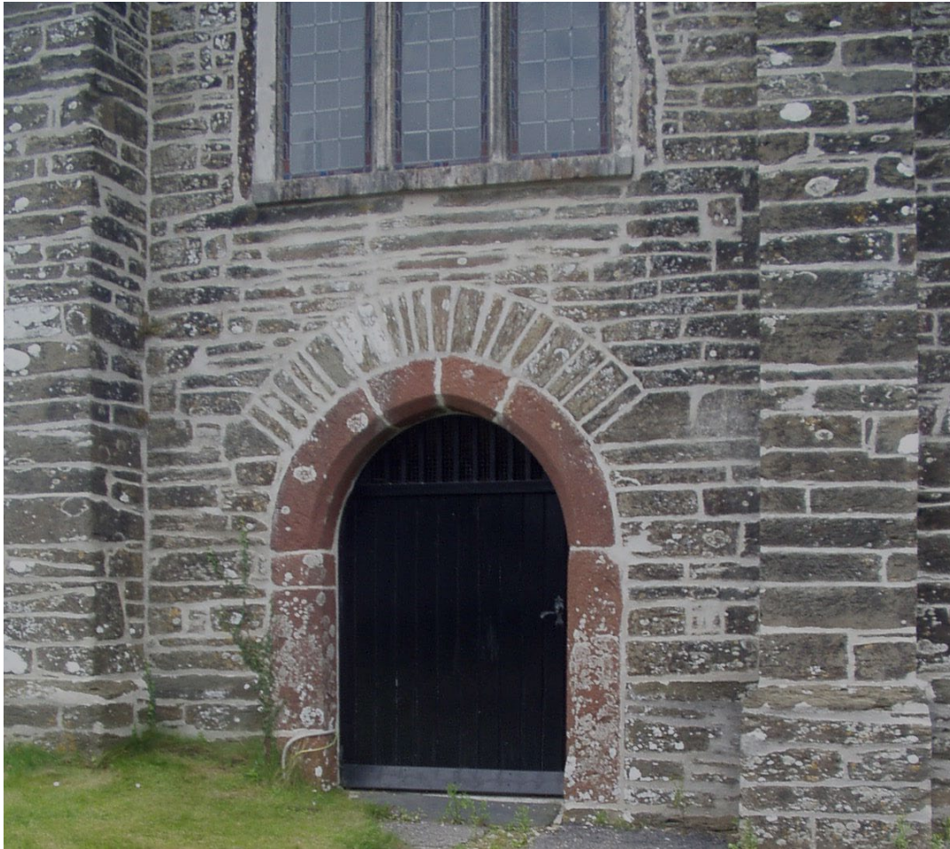
Figure 6. Black-stained slate with red sandstone dressings round door, west end of St Peter's, Cornworthy. Detail of the right buttress below shows the characteristic buff weathering.
