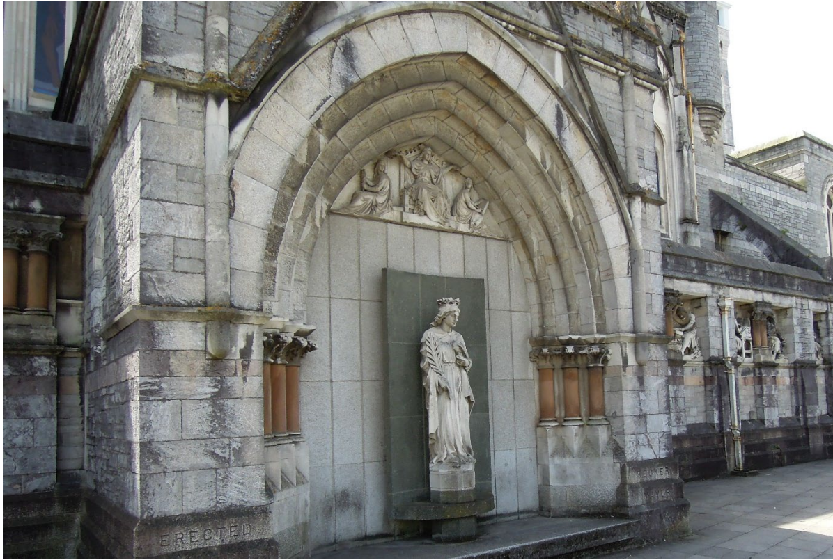
Figure 6. The Guildhall, Plymouth. The elaborately detailed façade is mainly of local mid-Devonian limestone with some Portland Stone detailing and red granite pillarettes
