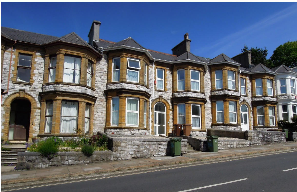
Figure 8. Terrace of C19 houses, of Middle Devonian limestone with dressings of Ham Hill Stone, Sutherland Road, Plymouth.
