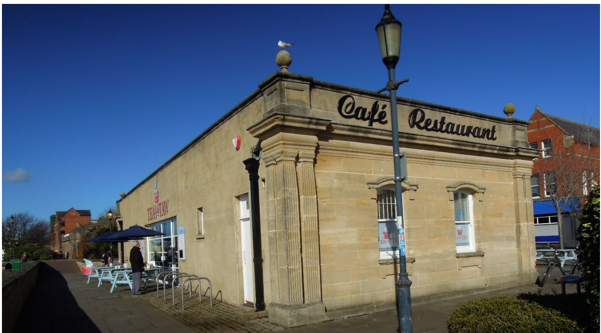
Figure 7. Tea by the Taw Restaurant, Barnstaple. The wall facing the river (left hand side of photo) is of artificial stone, the rest is finished in Doultong Stone.
