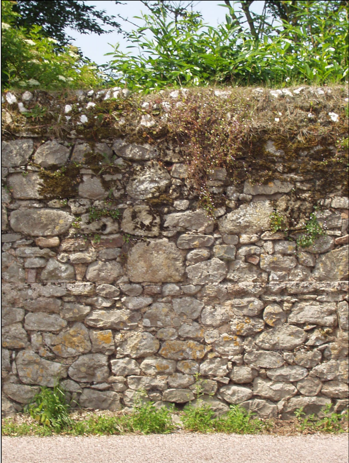
Figure 2. Rounded boulders of glauconitic sandstone probably collected from Sidmouth beach. Boundary wall of Sid Abbey estate, Sid Road (West), north of Sidmouth. The coping is of flint cobbles.
