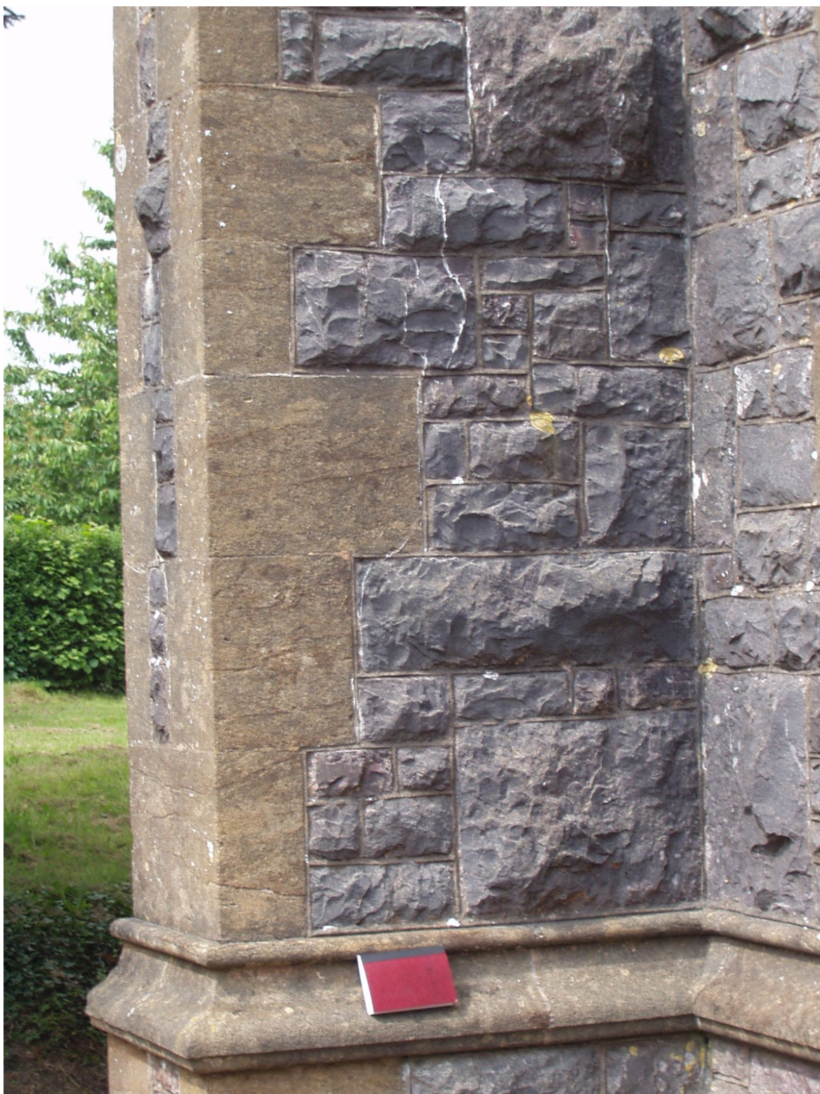
Figure 6. Tower of St John the Baptist' church, Ashbrittle. The dark grey Westleigh limestone lacks noticeable chert bands. The quoins are of Ham Hill Stone.
