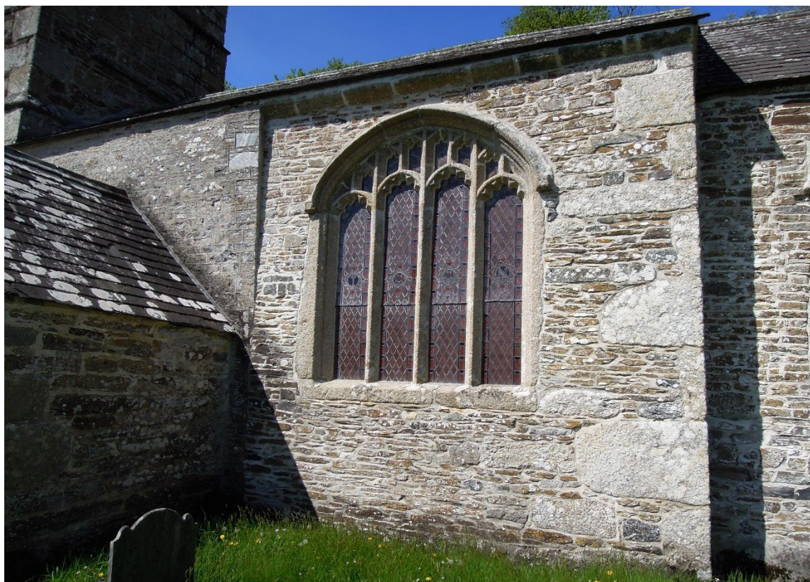
Figure 13. St Peter's church, Lewdon, south side of nave. Slate and granite rubble walling with huge blocks of Dartmoor granite used for the quoins and granite dressings round the large Perpendicular window.
