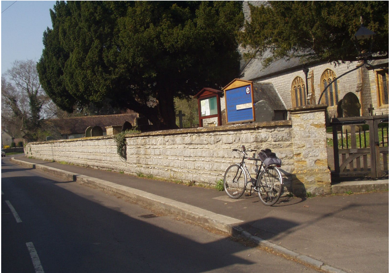
Figure 13. Wall of St Catherine's churchyard, Drayton. Blue Lias limestone laid in courses of different thickness.
