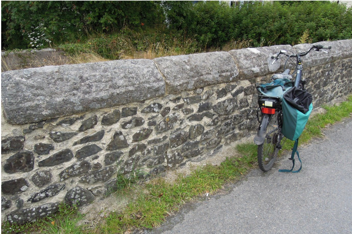
Figure 29. Bridge over the mill leat, Peter Tavy. The parapet is of altered gabbro with coping of Dartmoor granite.
