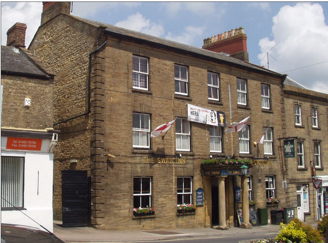
Figure 3. Swan Inn, Church Street, Crewkerne. Ham Hill Stone ashlar front wall, Inferior Oolite limestone gable end.
