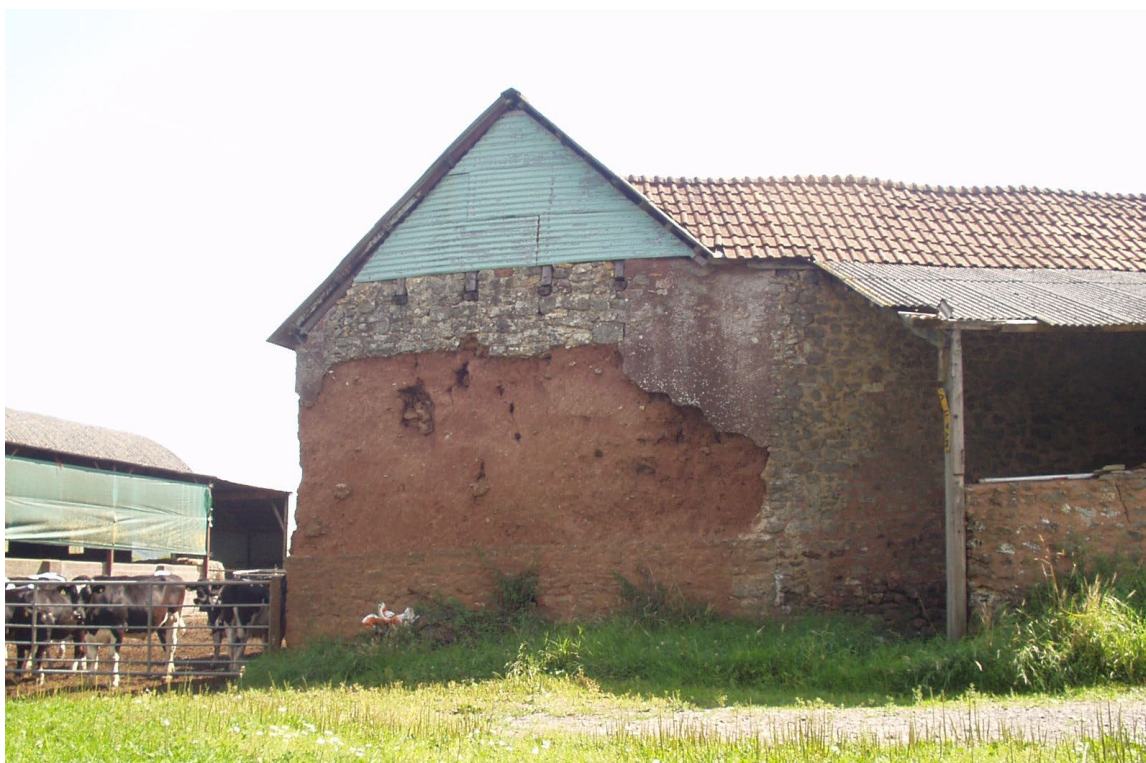
Figure 4. Outbuilding, Allercombe Farm, Ashill. Corrugated iron cladding in the apex of the gable end. The building is otherwise composed of cob on a chert rubble footing with a tile roof. Unusually, parts of the gable end other than the footing are of stone. It is probable that the tiles replace original thatch and the gable end was probably originally half hipped.
