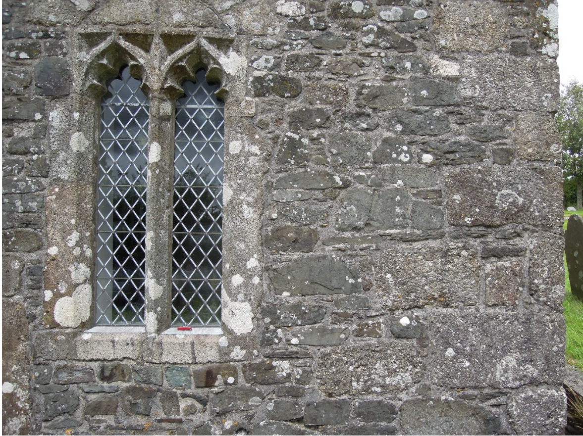
Figure 8. Chancel of St Peter's, Peter Tavy. The walling is of altered gabbro coded 91. The window dressings are of granite and Roborough Stone and the quoins of granite.
