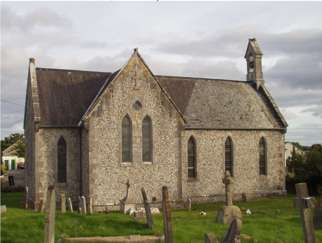
Figure 3. St Paul's church, Chudleigh Knighton, finished almost entirely with flint which is not knapped. Quoins and dressings are of grey limestone from Torbay.
