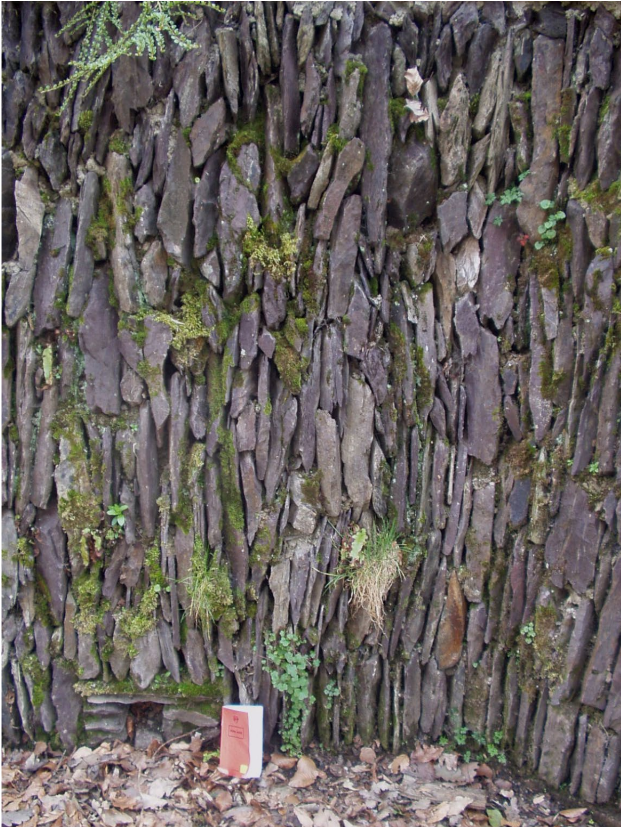
Figure 3. Cleaved sandstone with violet pigmentation, laid on edge; embankment to Northmoor Road, Near Dulverton.
