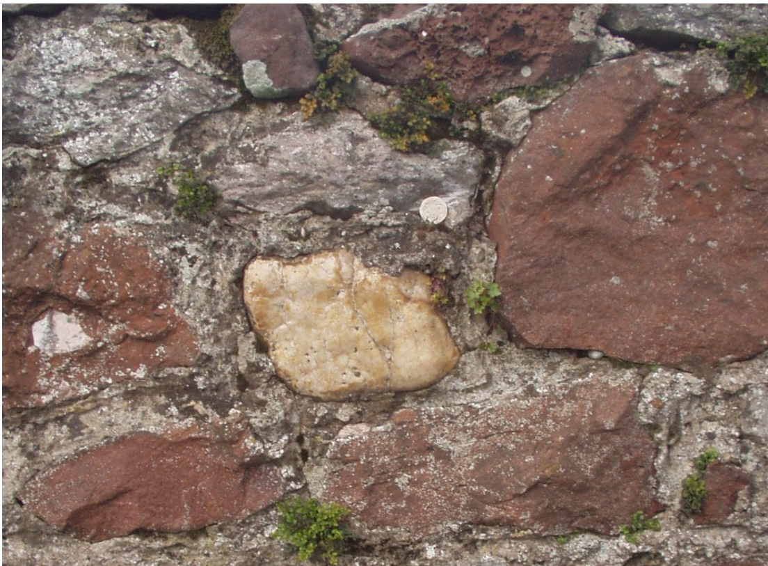
Figure 1. Abraded cobble of white vein quartz in a roadside wall mainly composed of purple porphyry and pale grey limestone, Dawlish Warren.
