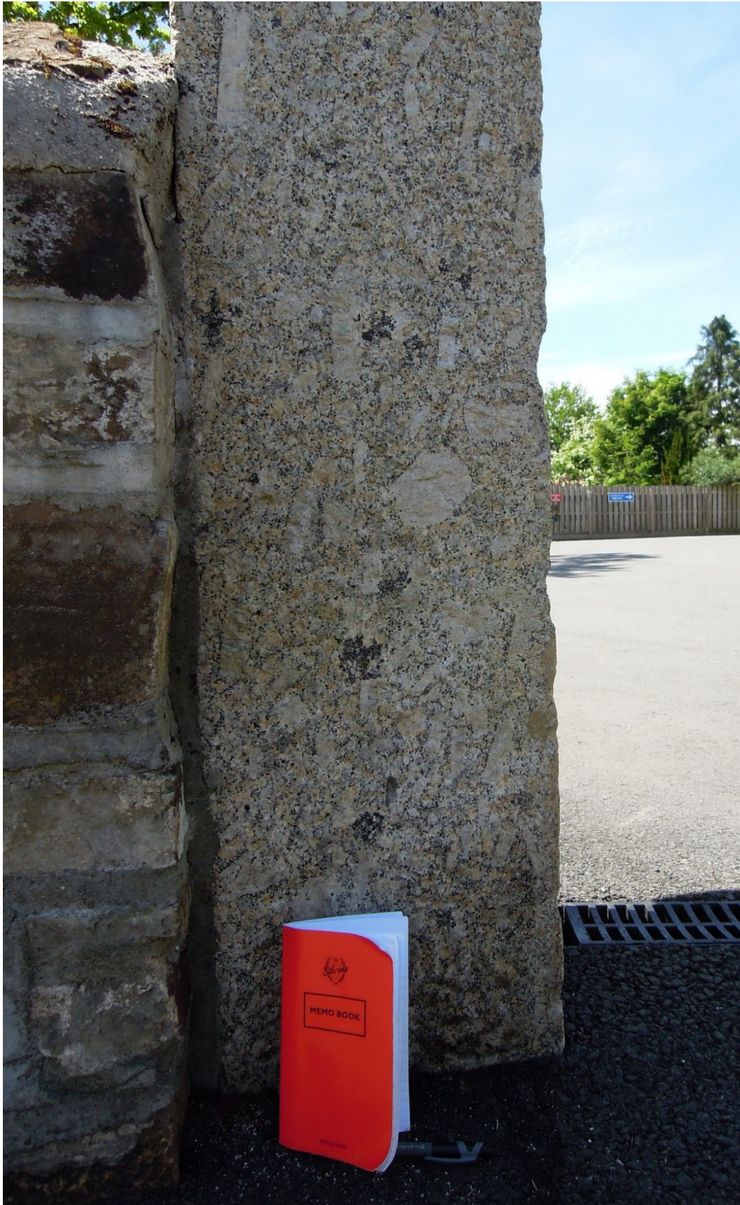
Figure 11. Monolith gatepost, west side of North Road, Holsworthy. The granite has roughly aligned feldspar phenocrysts and dark knots enriched in tourmaline.
