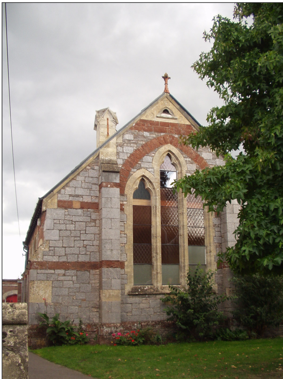
Figure 4. Methodist church, Exminster. The walls are of pale grey limestone from Torbay, with decorative string courses and outer relieving arch of red Heavitree Breccia. The dressings of the window and a few additional strategically placed blocks are of Bath Stone.
