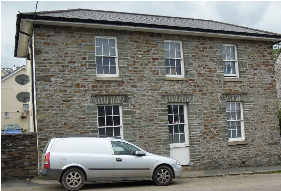
Figure 5. Pale grey-green slate weathered orange with some Hurdwick Stone and granite in the quoins. Callington Road, Tavistock.
