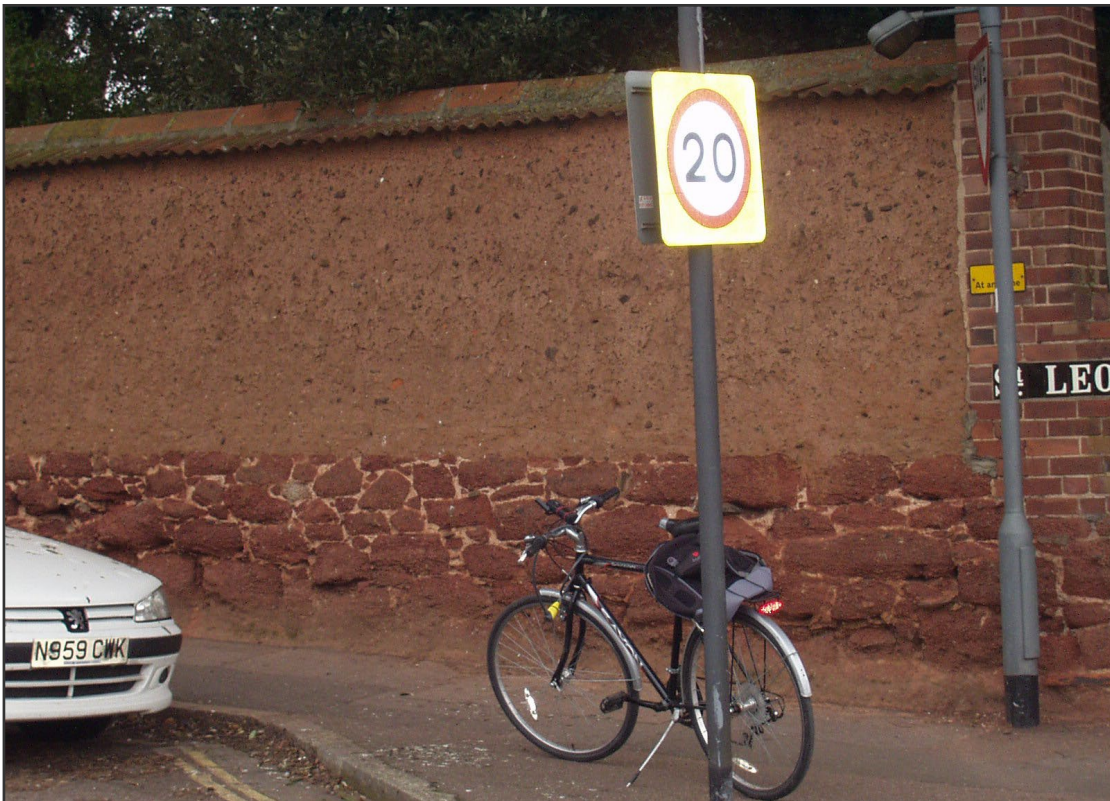
Figure 6. Junction of Topsham Rd. and St. Leonards Rd., Exeter. Cob with tile coping over Heavitree Breccia rubble.
