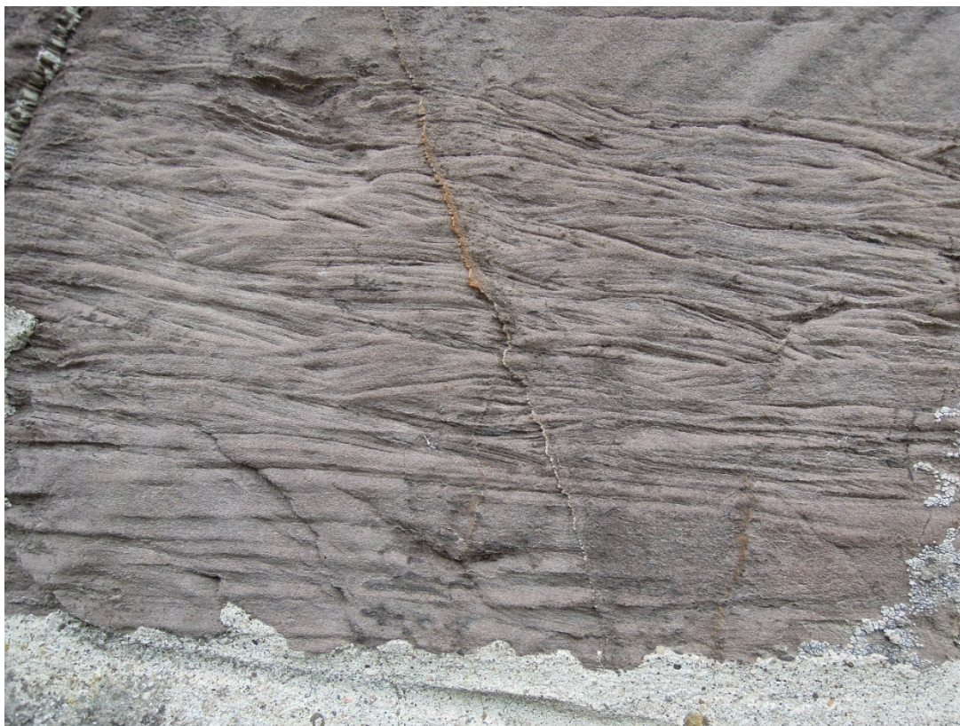
Figure 6. Ripple drift cross-bedded sandstone, chancel of St Hieritha's church, Chittlehampton. The stone has been laid upside-down. Width of view, 30cm.
