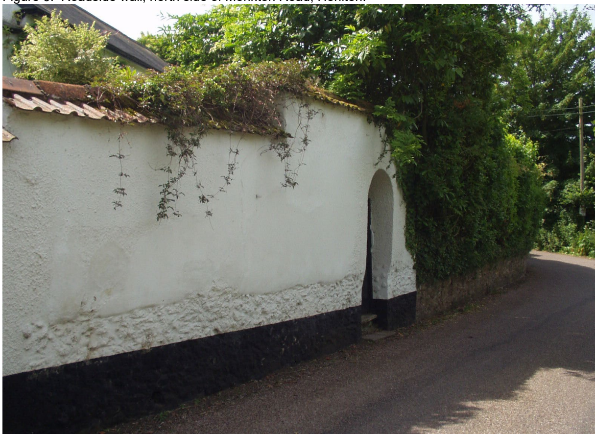
Figure 4. Roadside wall, Ellon House, Harpford. Cob wall on a footing of painted stone rubble and with a coping of tile and corrugated iron.
