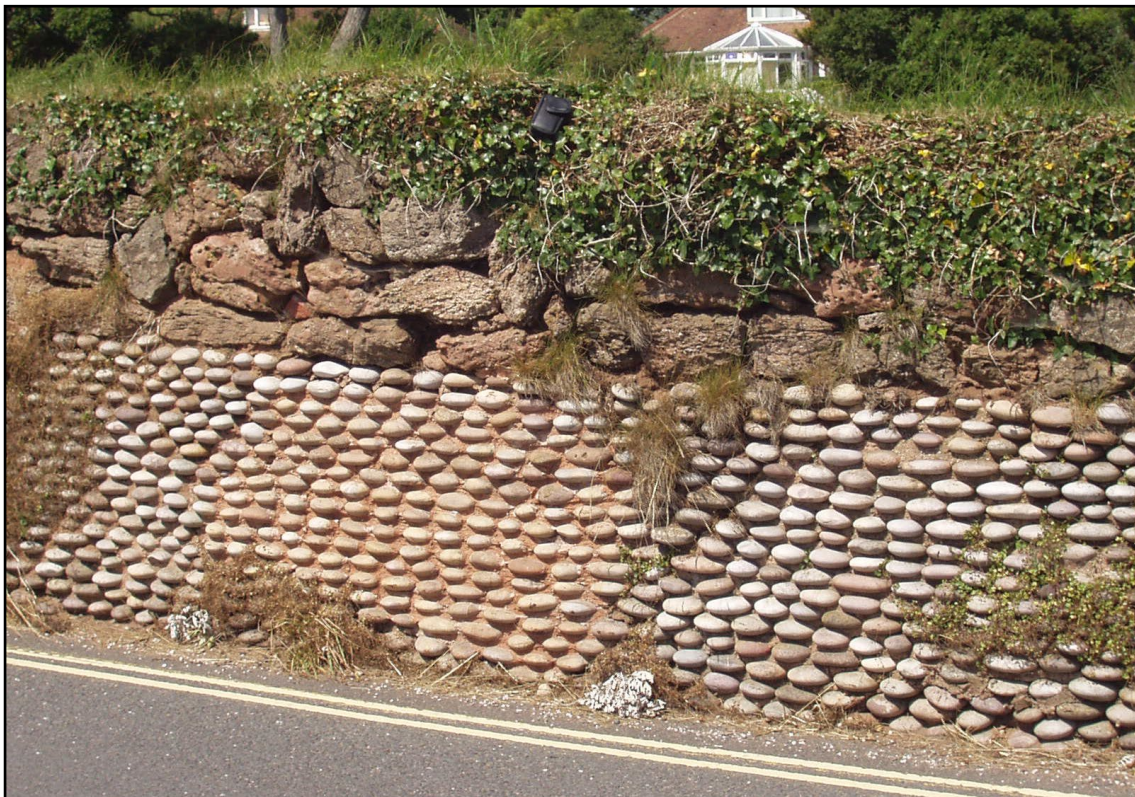
Figure 2. Salting Hill, Budleigh Salterton. The top of the wall is of red pebble conglomerate from the Otter Sandstone. The lower part is finished in carefully matched cobbles from the Budleigh Salterton Pebble Beds.
