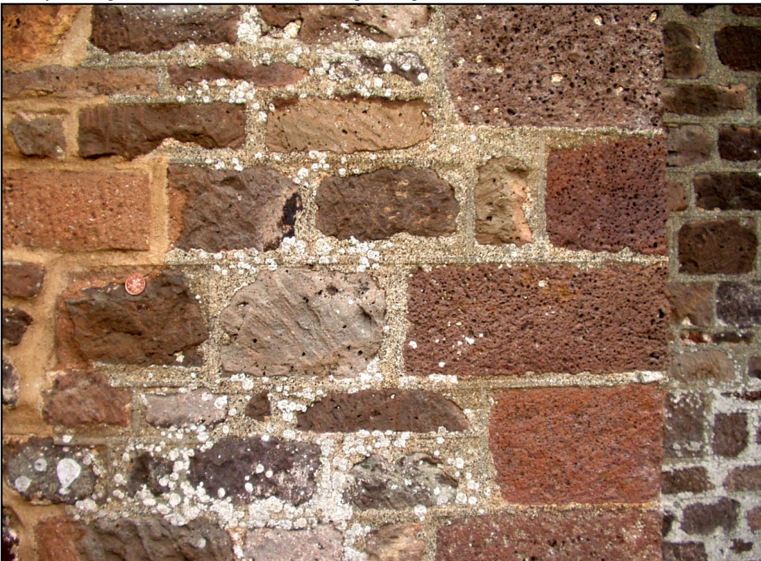
Figure 3. North transept, St Mary's church, Poltimore. Vesicular lava is used for the quoins but lava mainly lacking vesicles is used in the wall. The block above and to the left of the 2p piece is a repair of artificial stone.
