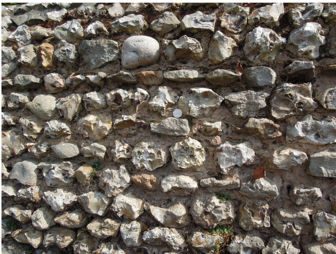
Figure 4. Wall next to Larbi Cote, Station Road, Sidmouth. Mainly of flint with minor chalcedonic sandstone and chert.
