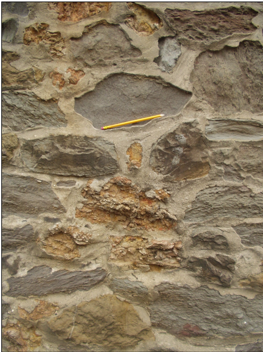
Figure 2. House wall, Sea Town. The ochreous blocks with very irregular surfaces and some pink pigmentation below the pencil, in the lower left and top left corners are of Junction Bed limestone. The rounded grey blocks are fine-grained sandstone probably from the Thorncombe or Down Cliff Sands.
