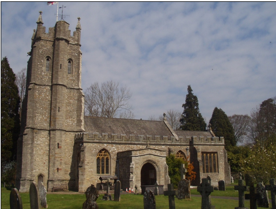
Figure 4. St Giles' church, Bradford-on-Tone. Quoins and dressings are of North Curry Sandstone with some Portland, Ham Hill and Bath Stone while the walls are a mixture of this sandstone and Upper Greensand chert.
