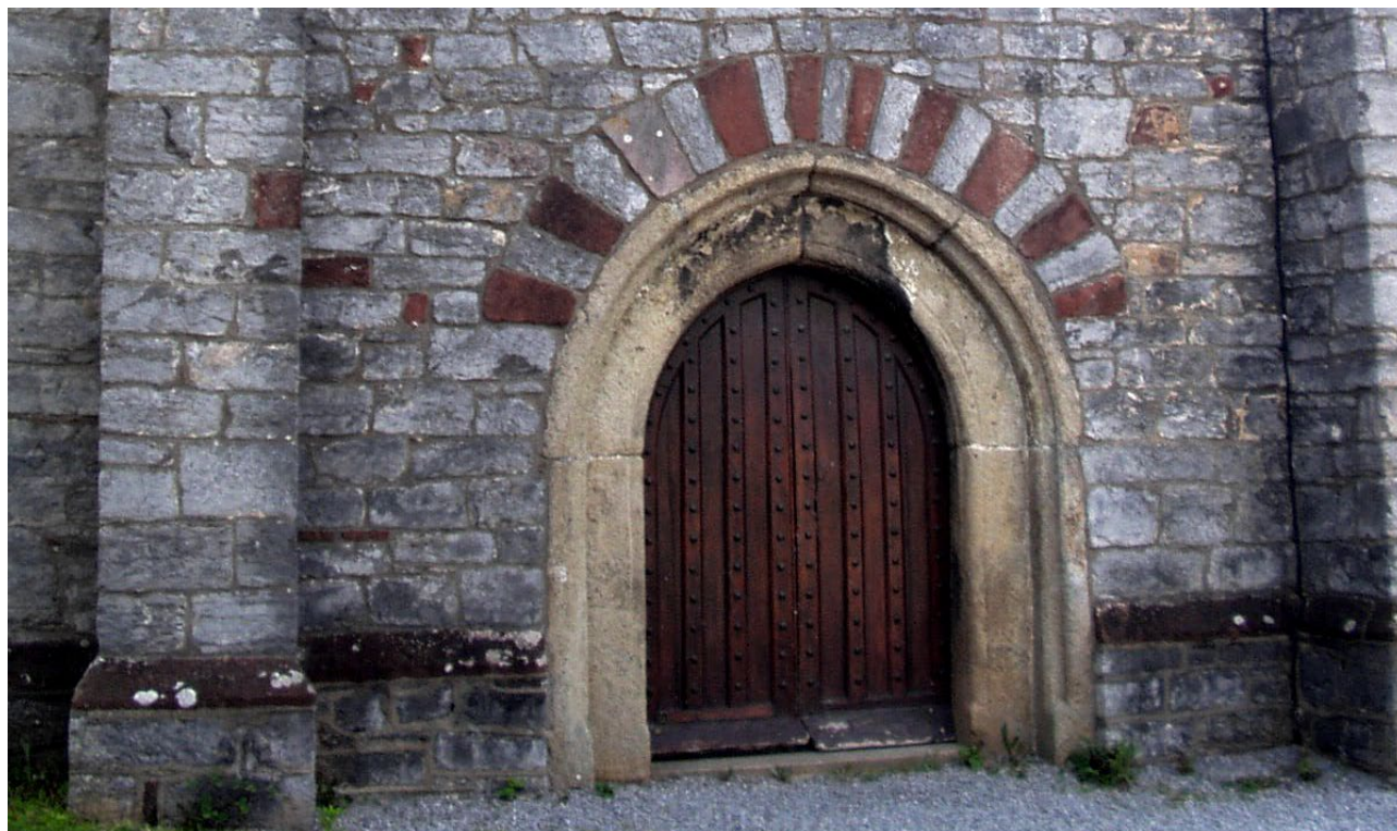
Figure 20. Tower of St Michael's church Kingsteignton. The dressings of the west door and the window above are of Dartmoor granite with very large shaped blocks used for the doorway. The relieving arches are of alternating grey mid-Devonian limestone and red Permian sandstone. The walls are of grey limestone.
