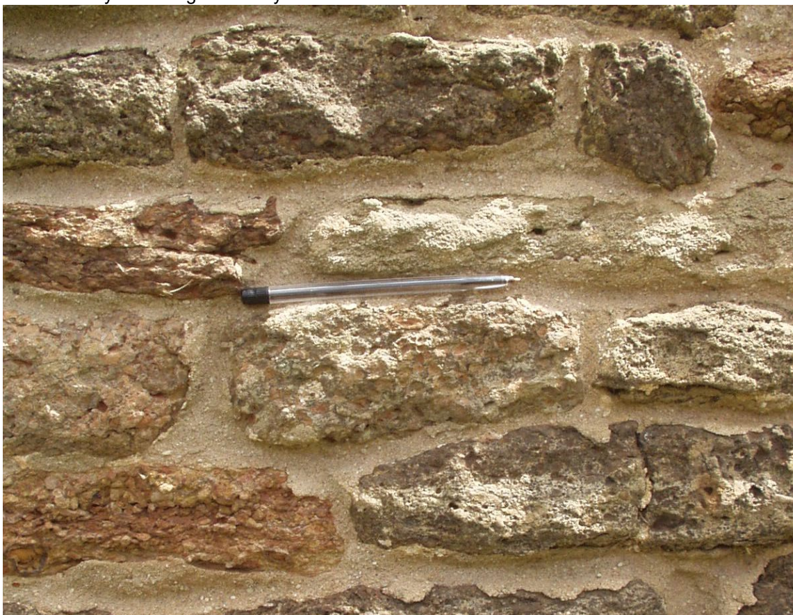
Figure 3. Tower of St Gregory's church, Harpford. The pale sandstone block above the pencil has a pimply texture matched by some of the adjacent blocks of mud-flake conglomerate (Code 82).
