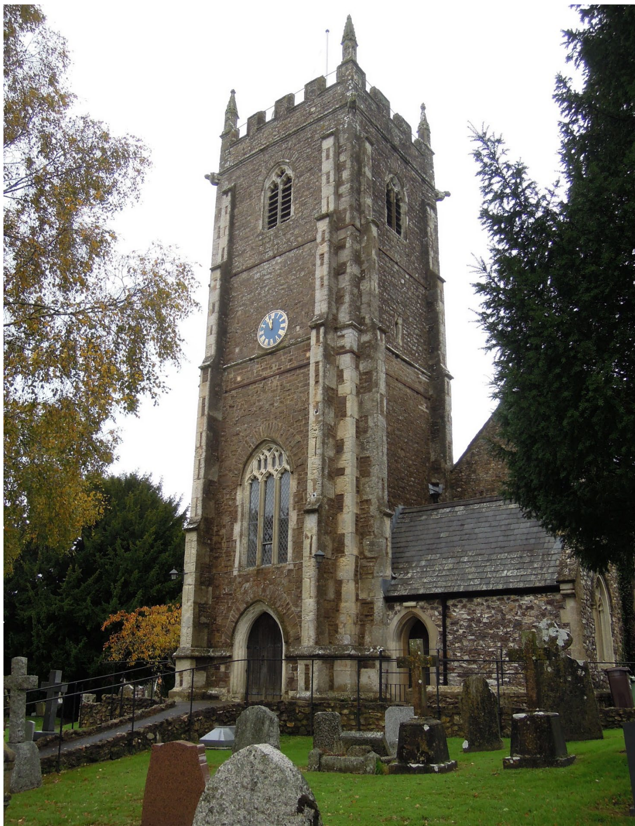
Figure 16. Tower of St Mary's church, Kentisbeare. The quoins and staircase are made of decorative alternating large blocks of Beer Stone and maroon Bude sandstone from the nearby Upton Quarry.
