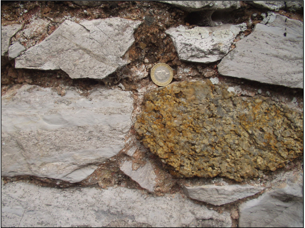
Figure 1. Garden wall of Woodlands, Globefields, Topsham. Mainly composed of pale grey limestone from Torbay but including some blocks of yellowish granite of unknown origin (illustrated) and dark green dolerite.
