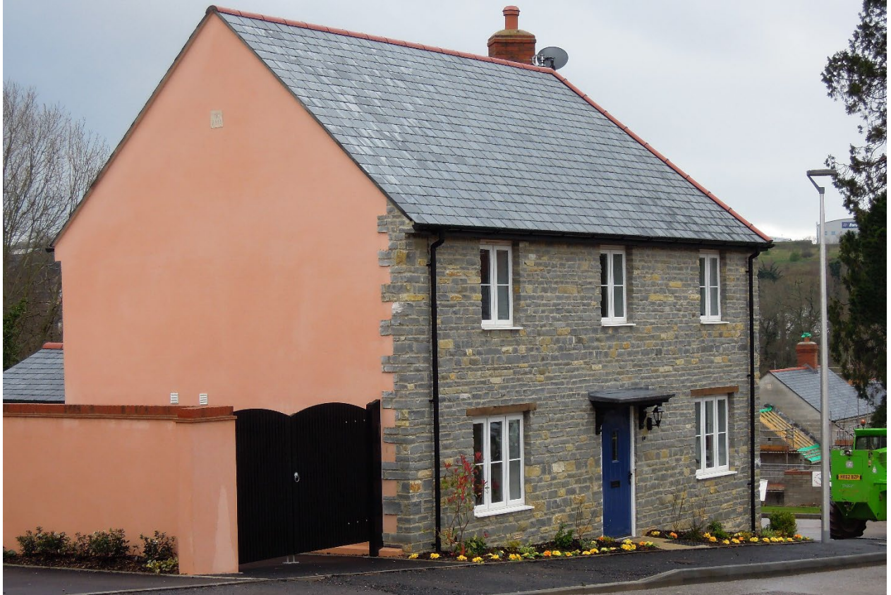
Figure 15. 1 Hillcrest Gardens, Exmouth. Blue Lias limestone finish to the front of the house including some cream and yellow blocks, breaking up the monotonous grey pigmentation.
