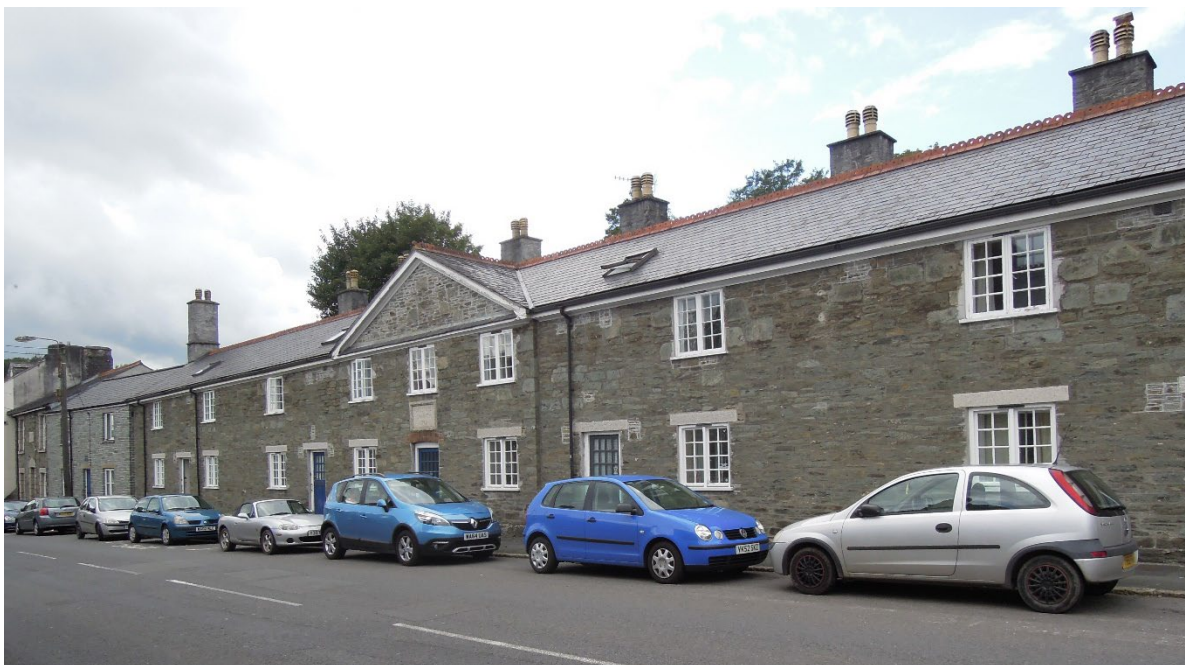
Figure 26. Ford Street Charity, Tavistock, of Hurdwick Stone with granite lintels to the ground floor windows.
