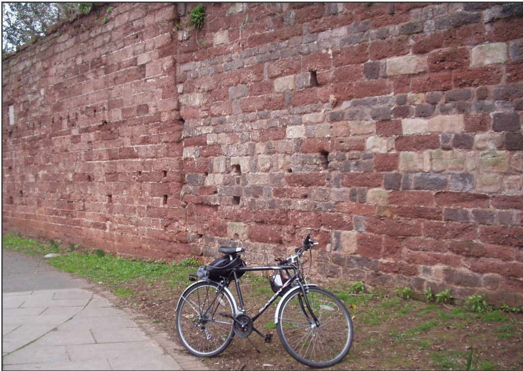
Figure 9. Exeter city wall 175m northeast of the South Gate. The near part is composed of a mixture of Heavitree Breccia (red), Exeter volcanics (violet), probably from Rougemont or Northernhayes and fawn sandstone (Exeter Group, Otter Sandstone or Salcombe Stone). The far part is composed entirely of Heavitree Breccia. It contains a stone dated 1743 just visible on the extreme left of the photograph.
