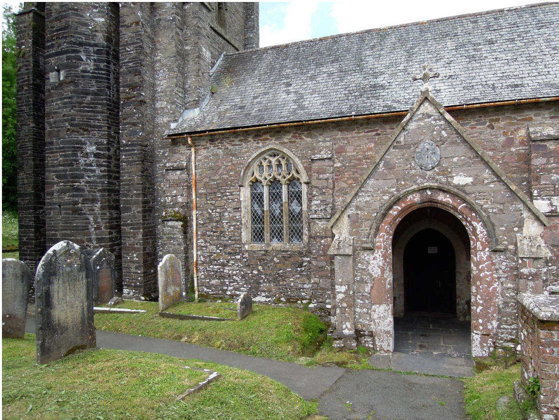
Figure 8. St Leonard's church, Halwell. The tower is made of dark grey slate, the nave and south porch of medium grey slate, both referred to slate of Code 59.
