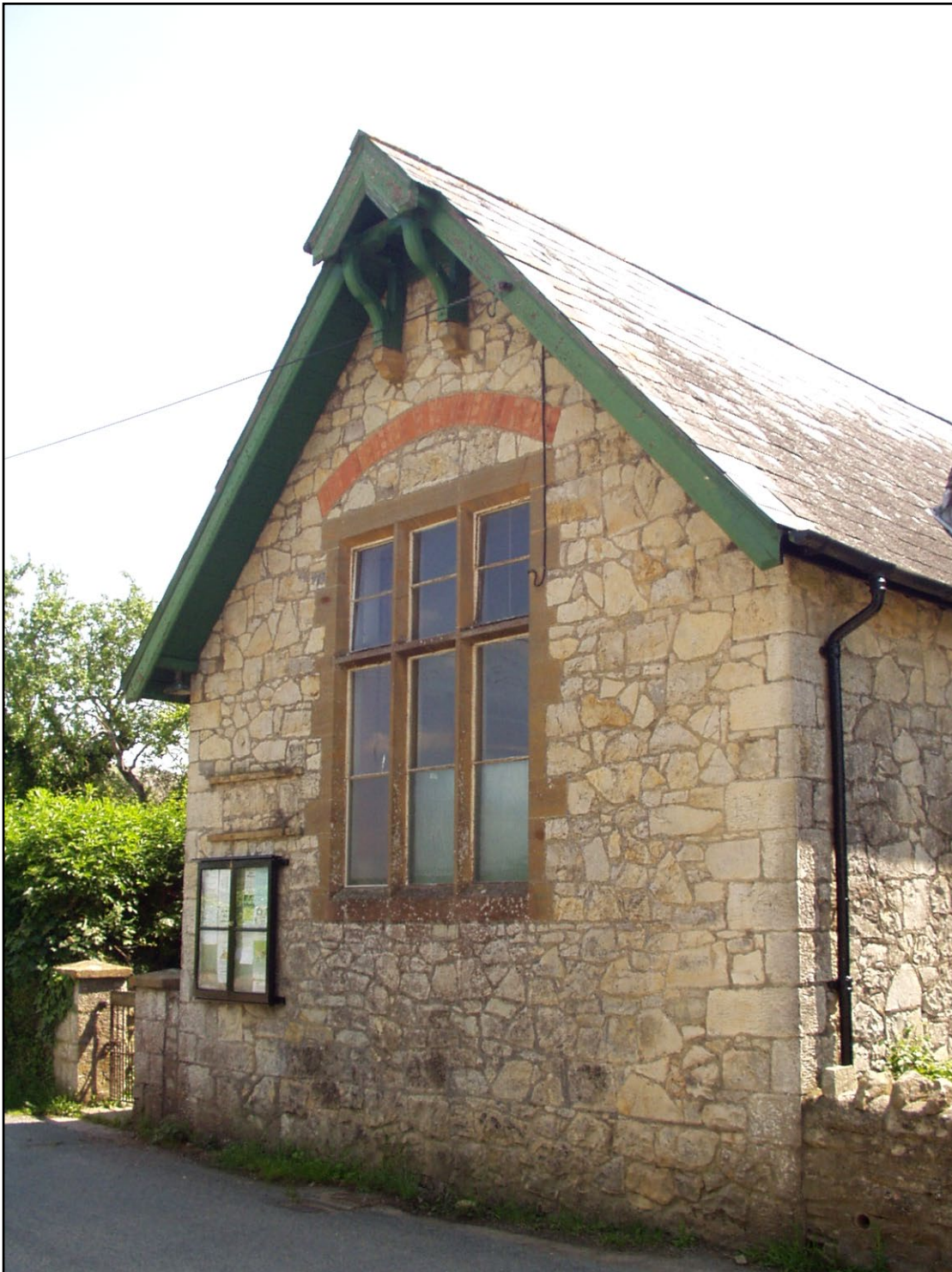
Figure 2. The School House, Isle Abbots. The walls and quoins are of White Lias limestone. The dressings round the window are of Ham Hill Stone with a relieving arch of brick. The wall also contains a few blocks of Blue Lias limestone.
