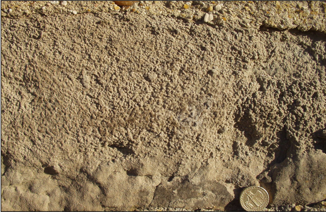
Figure 3. "Droplet" texture believed to be caused by enclosing grains of sparry calcite. St Mary's church, West Buckland.
