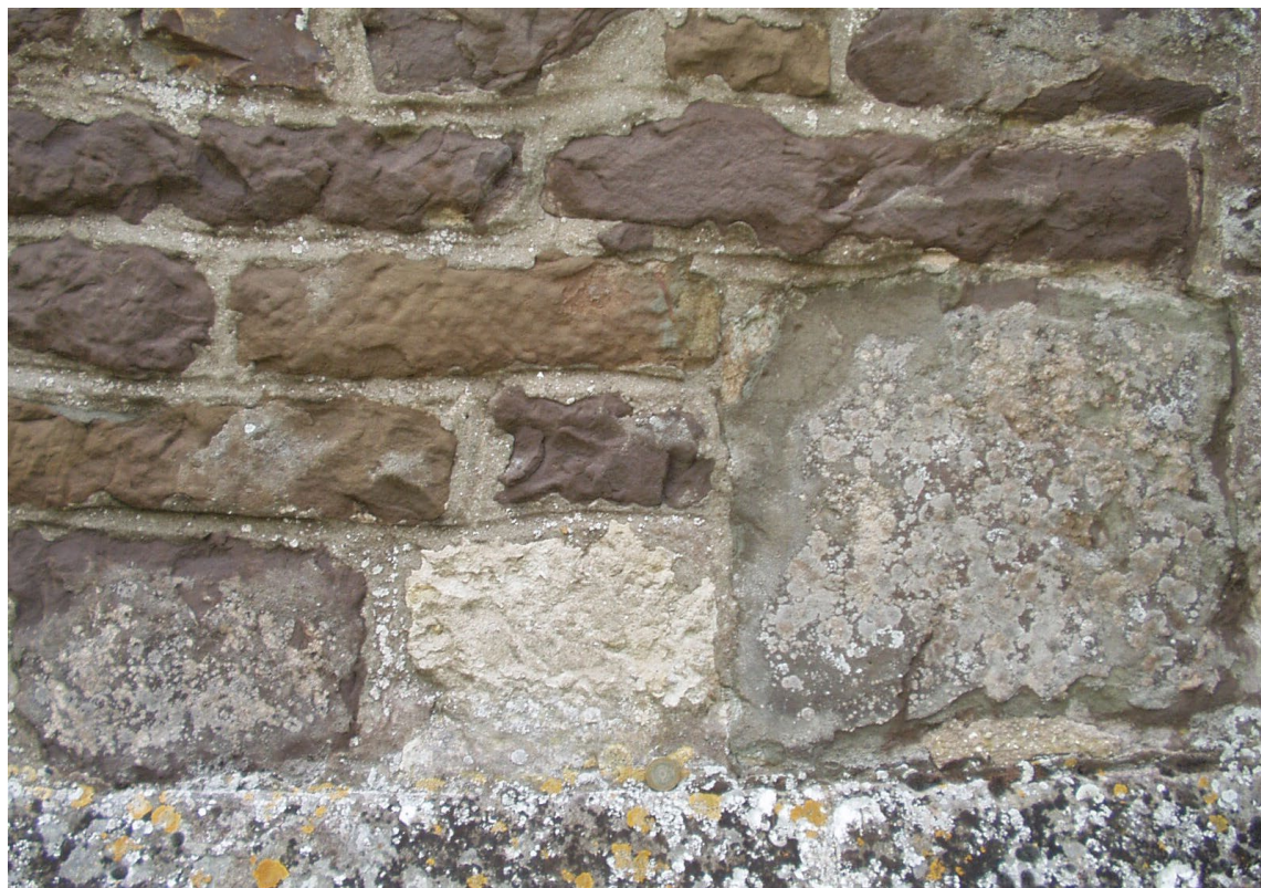
Figure 1. Tower of St John's church, Plymtree. Most of the stone in this picture is maroon sandstone from the Bude Formation but the block in the centre bottom is Beer Stone and the block to its right is pale green-grey sandstone believed to be from the Otter Sandstone.
