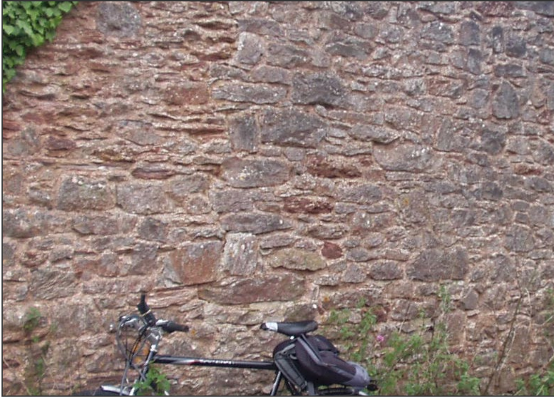
Figure 10. Red stained slate and medium-grey limestone, garden wall, Combe Fishacre, possibly from one of the limestone members of the Nordon Formation.
