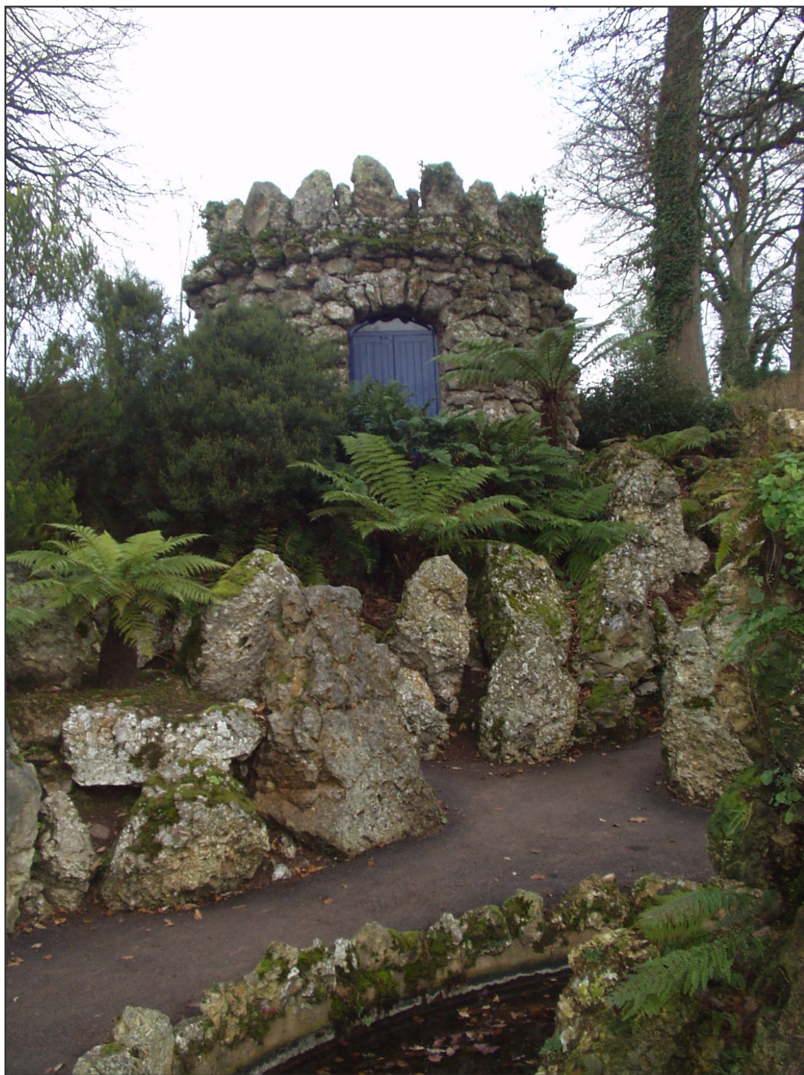
Figure 3. Rockery and wall of the Fish House, Bicton Park, Bicton. A note inside the Fish House records that the chert breccia was hauled from the top of the cliff between Sidmouth and Beer.
