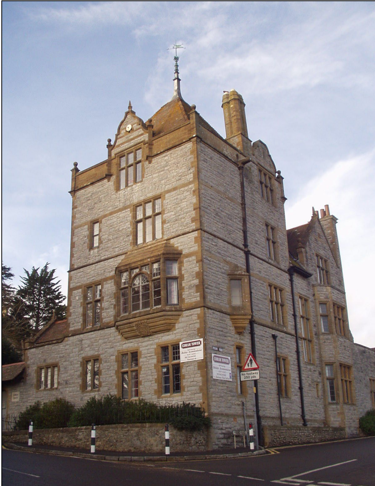
Figure 2. Coram Tower, Lyme Regis. The quoins and dressings are of Ham Hill Stone. The uniformly grey colour of the Blue Lias suggests a source in the sea cliffs or at any rate, beyond the zone of surface weathering.
