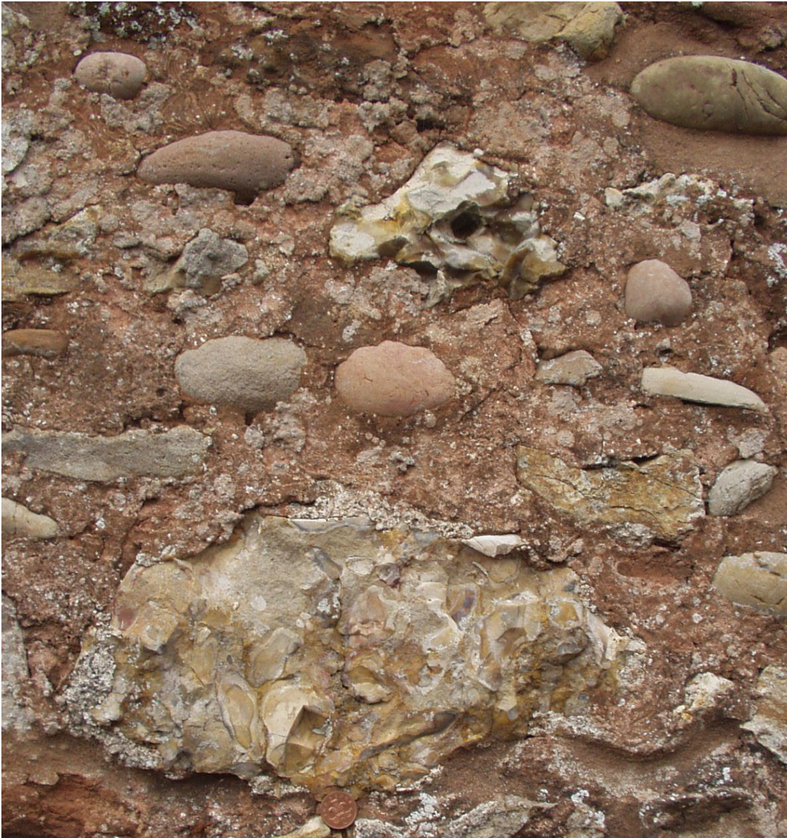
Figure 1. St Luke's Church, Newton Popleford. The photo shows rounded cobbles of quartzite from the Budleigh Salterton Pebble Beds and yellowish chert breccia from the Clay with Flints. However, elsewhere the wall is mainly made of Otter Sandstone and mud-flake conglomerate.
