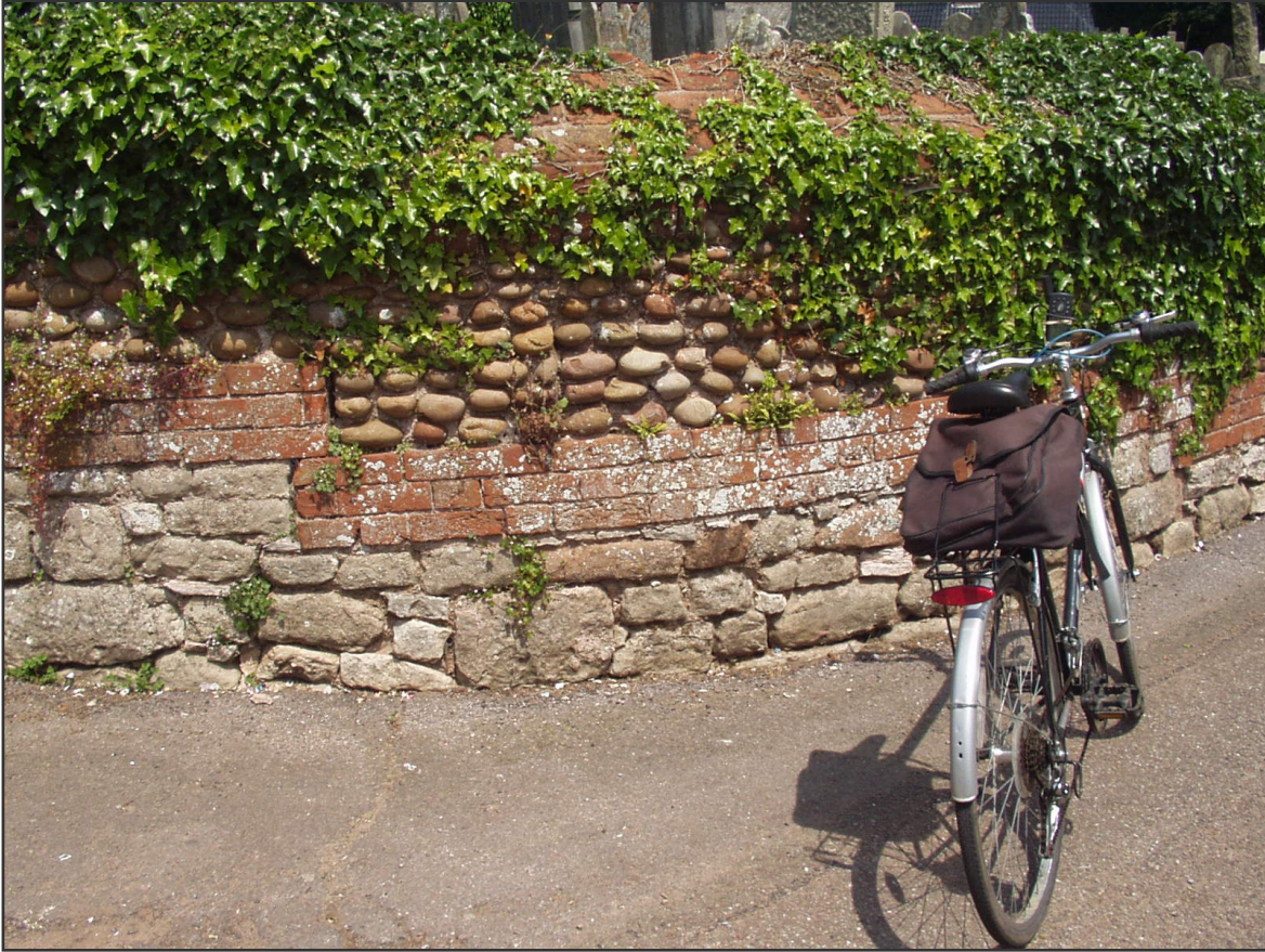
Figure 3. Wall outside the church gate, Woodbury. Stepped construction of fawn sandstone at the base followed by brick, then “Budleigh Buns” with a slate coping (according to the listed building citation but not visible in the photograph).
