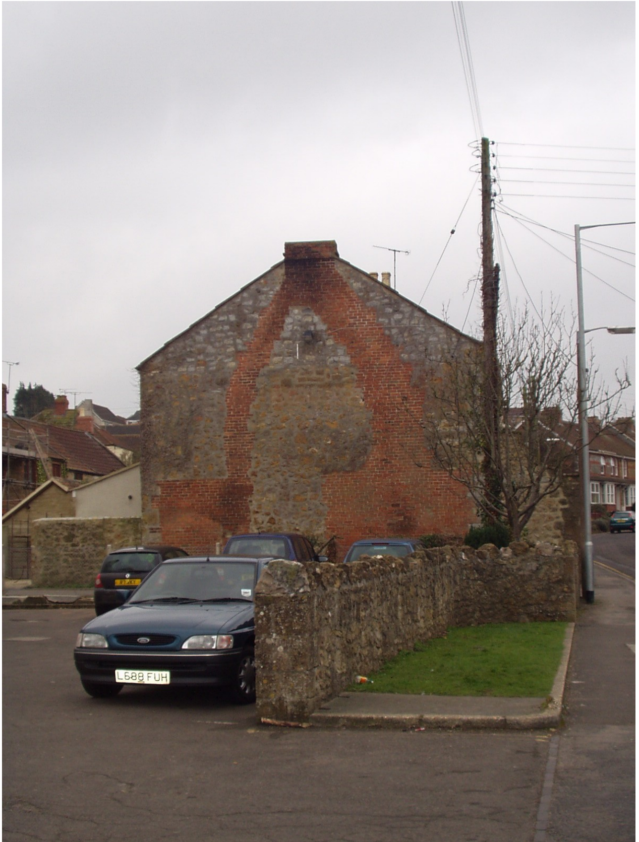
Figure 21. Gable end of 31 Ditton Street, Iminster. The wall is of Moolham Stone below with Blue Lias limestone in the apex of the roof. The fireplaces and flues are of brick.
