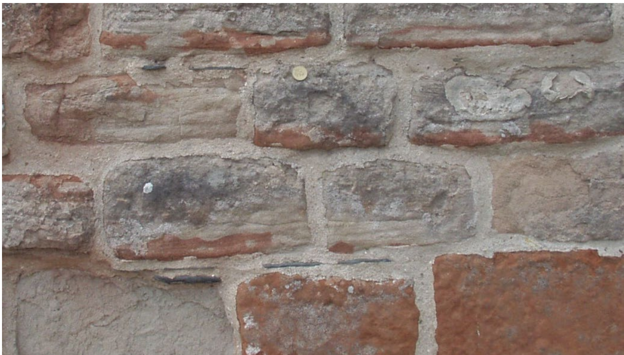
Figure 3. Single slates used fill the gaps between building stones. Vestry of St Swithin's, Woodbury. The red and white stone is sandstone from the Aylesbeare Mudstone Group.
