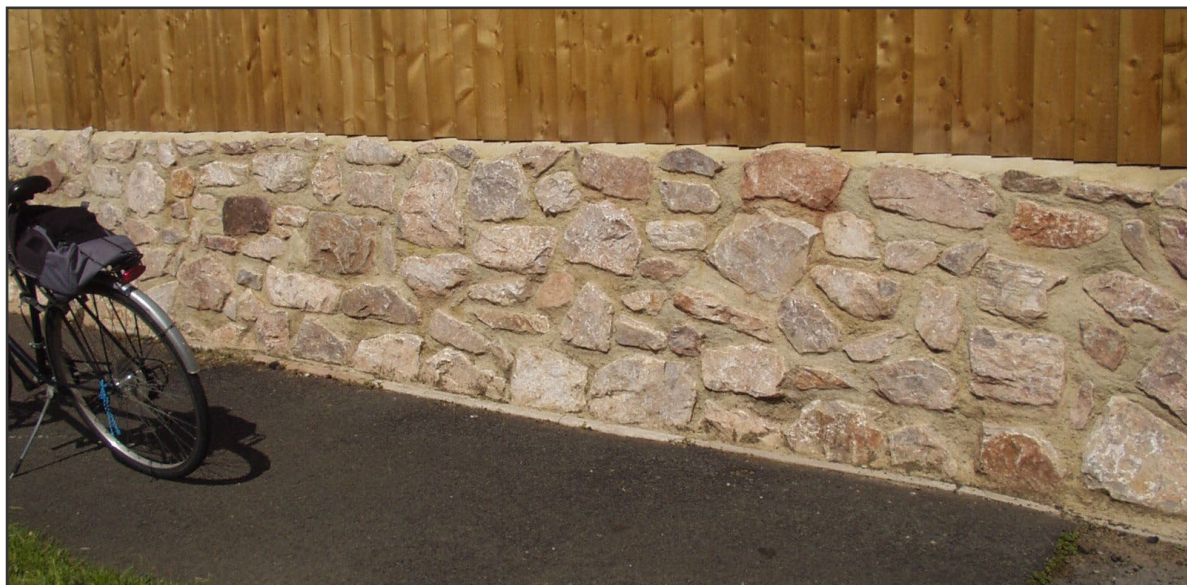
Figure 5. New wall of pale grey limestone with pink cast, probably reused. Rydon Road, Kingsteignton.
