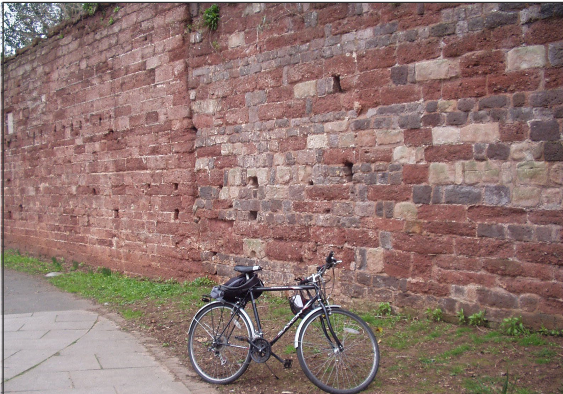
Figure 5. City wall, Exeter. The nearer part is composed of a mixture of Heavitree Breccia (red), Exeter volcanics (purplish grey) and fawn sandstone. In this case, it may be that the sandstone is Salcombe Stone (Code 14) rather than being won from older formations.
