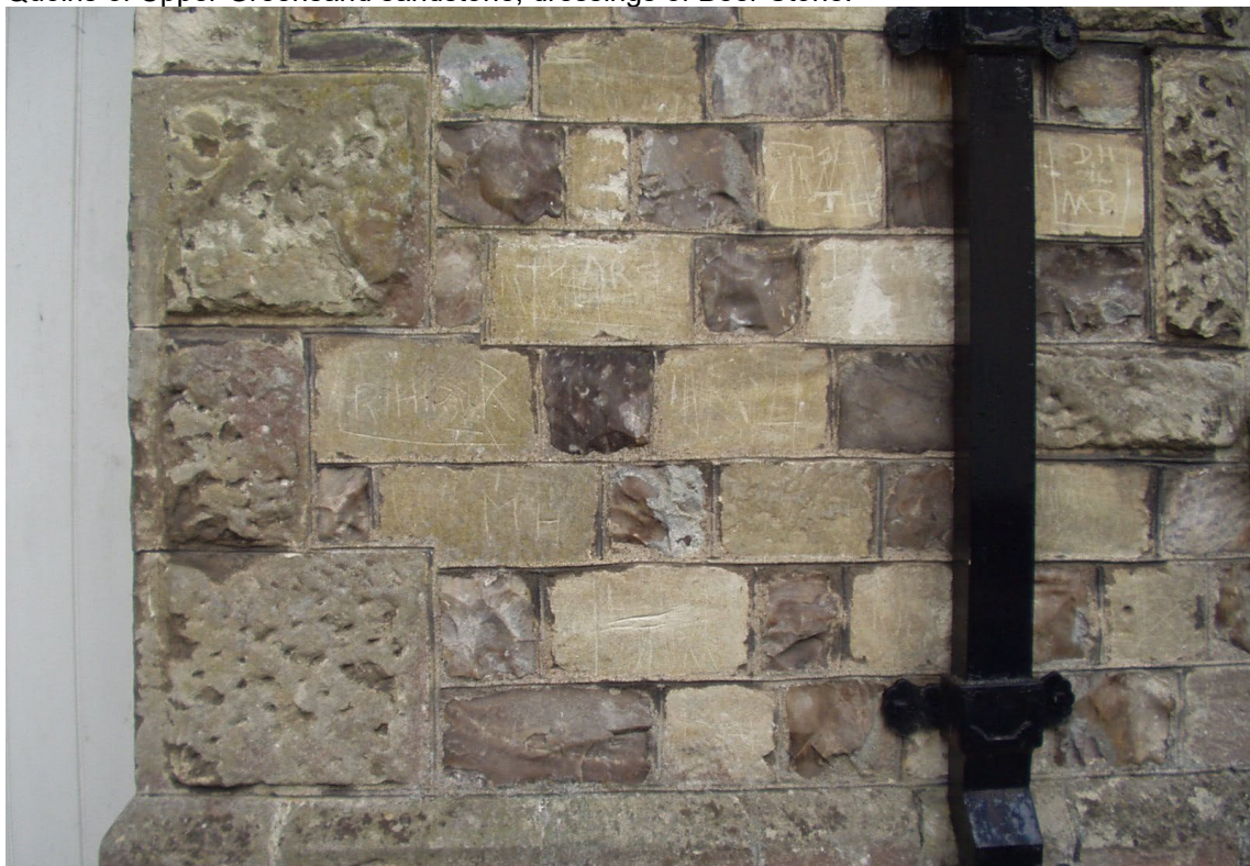
Figure 10. Parish Hall, Church Street, Winsham. The wall is made of alternating blocks of squared chert with hackly finish and yellow Upper Greensand sandstone with smooth finish.
