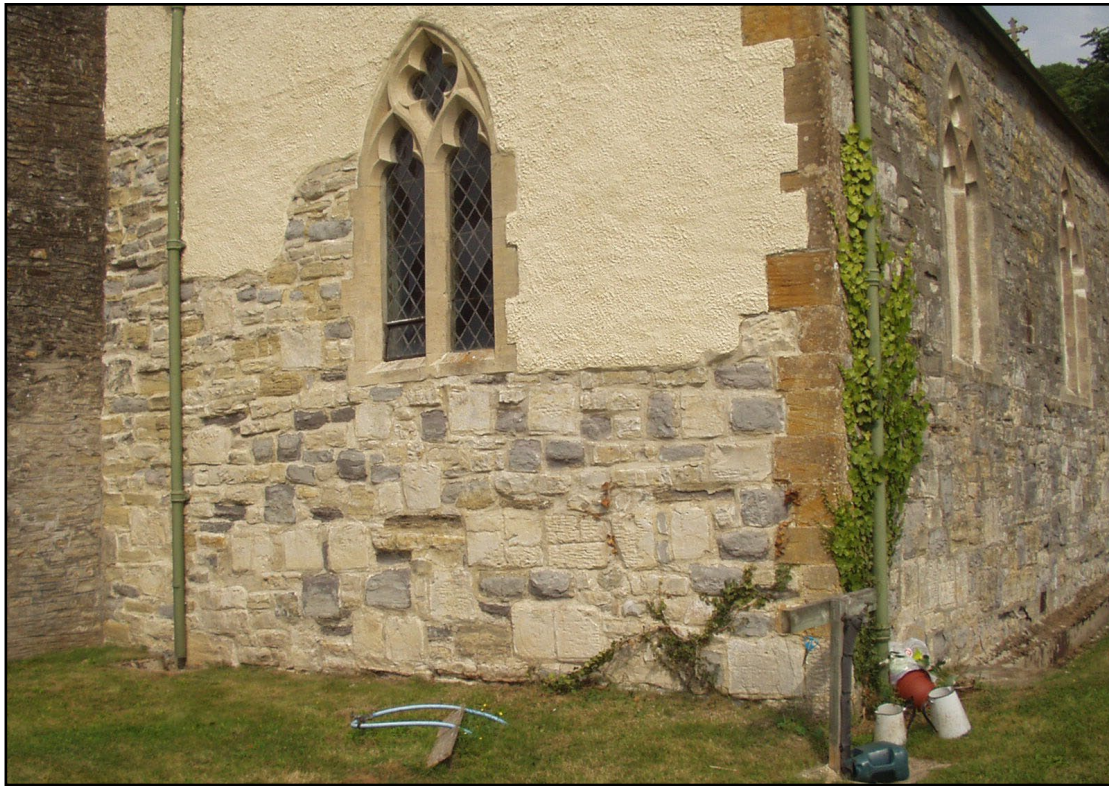
Figure 3. South aisle of St Mary's church, Stoke St Mary. Rubble wall of White and Blue Lias limestone, partly rendered. Note that the White Lias blocks are usually thicker than the Blue Lias ones. The quoin on the right is of Ham Hill Stone and the dressings round the window of Bath Stone.
