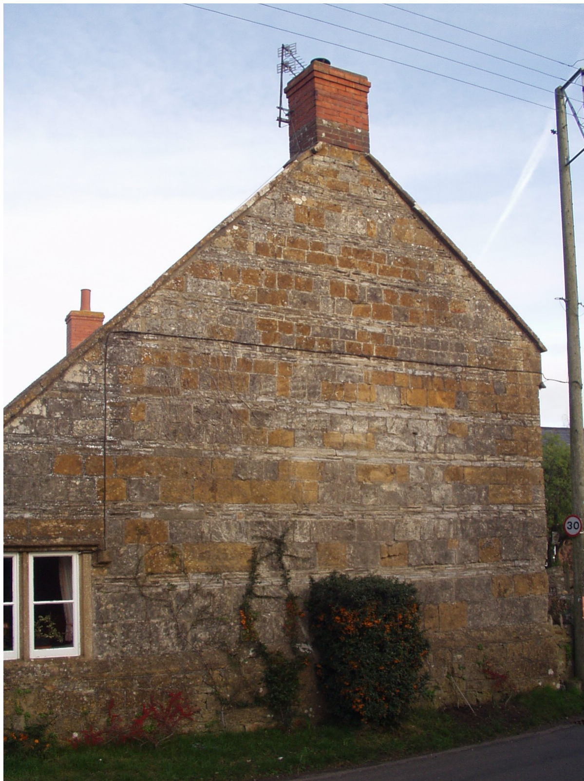
Figure 14. Gable end of Porch House, Broadway Road, Broadway. Two thin courses of Blue Lias limestone alternate with two thicker courses of grey Upper Greensand calcareous grit (Code 13) and yellow Moolham Stone (Code 66).
