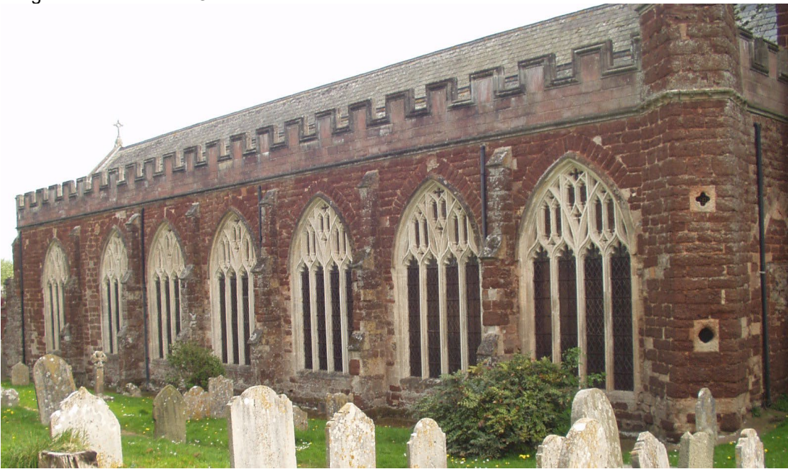
Figure 2. Beer Stone window dressings of the north aisle of All Saints church, Kenton. The wall is of red Heavitree Breccia and fawn sandstone probably from the Otter Sandstone Formation.
