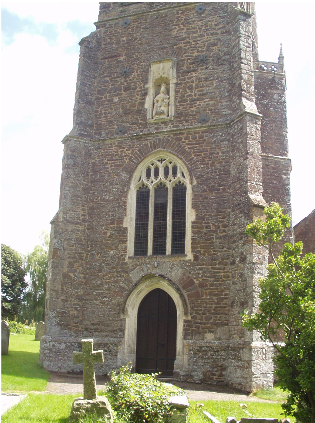
Figure 5. St John's church, Plymtree. The window dressings and the niche for the statue are of Beer Stone. The walling and relieving arches are mainly of maroon Bude Formation sandstone (Code 119) with minor Exeter volcanics.
