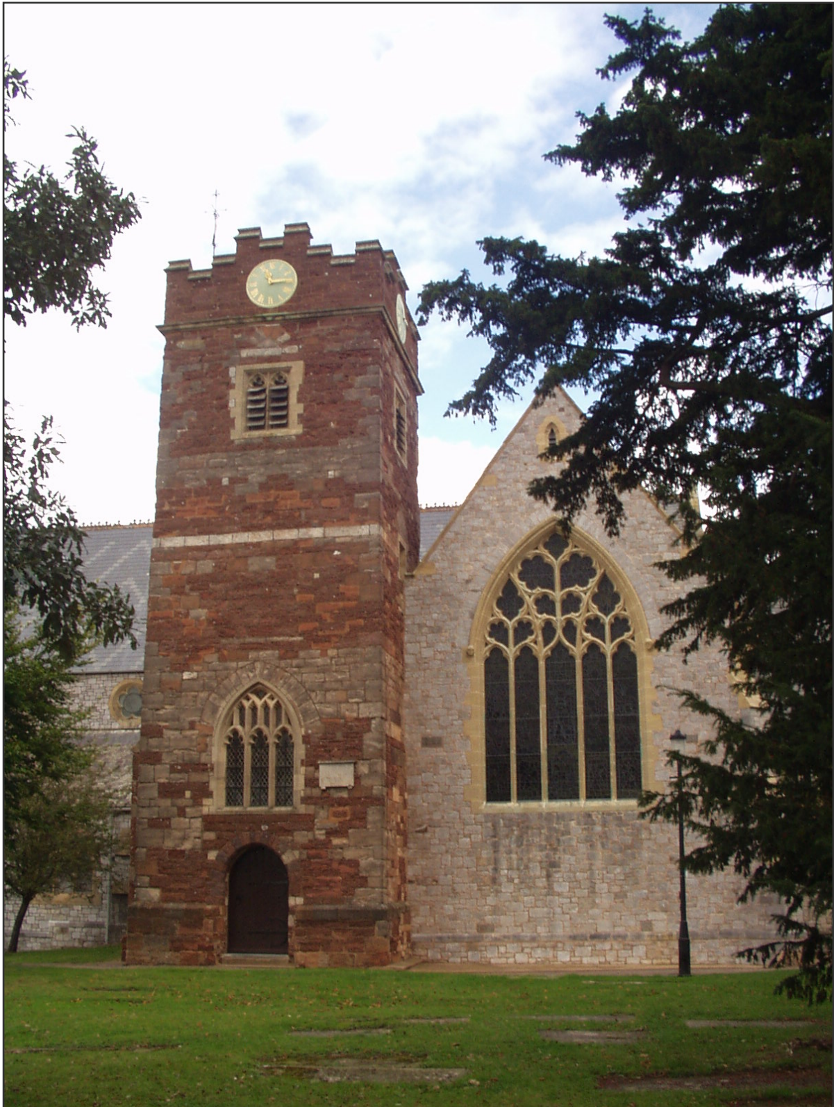
Figure 3. St Margaret's Topsham. The tower is medieval, composed of red breccia from Heavitree or Exminster, mottled sandstone from the Exmouth Sandstone and Mudstone Formation and minor Exeter volcanics.
