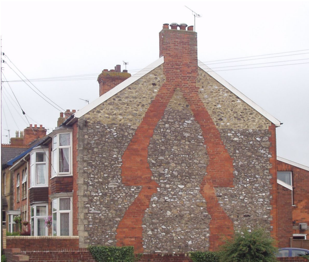
Figure 12. 19 Victoria Avenue, Chard. The gable end is of chert with flues lined with brick.
