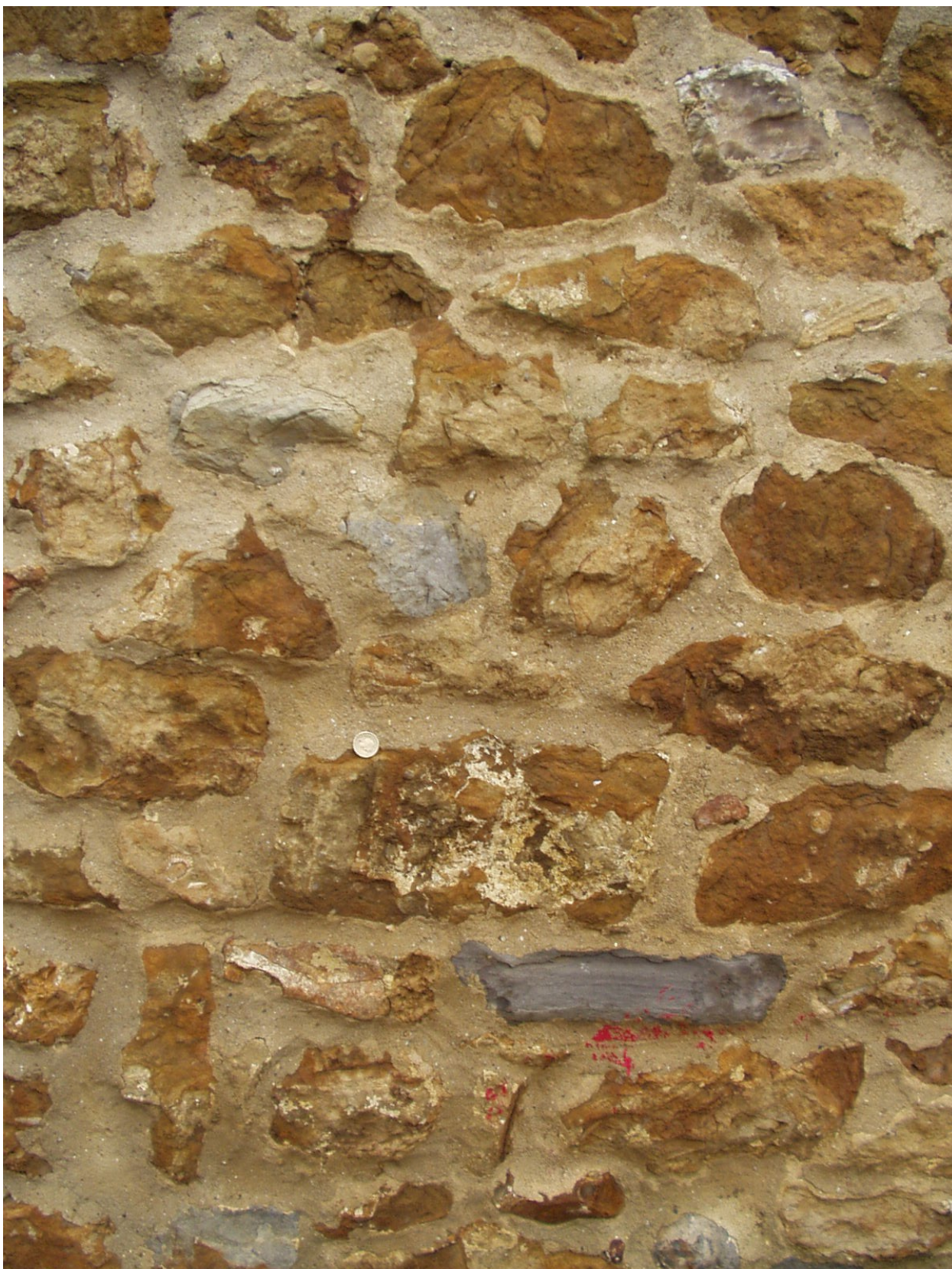
Figure 6. Wall adjacent to PAWS Pet Shop, Ilminster, composed mainly of ochre limestone from the Junction Bed with a few blocks of grey Lias siltstone.
