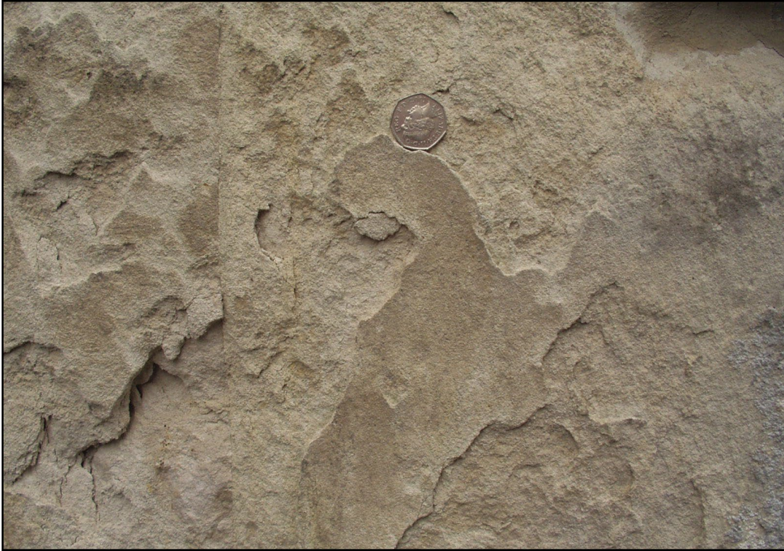
Figure 6. Buttress to the south aisle of St Andrew's church, Colyton. Characteristic surface flaking of Beer Stone.
