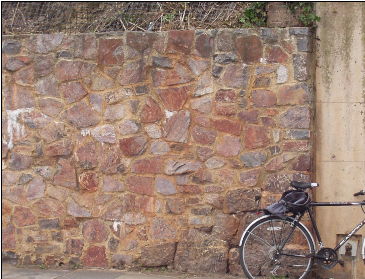
Figure 1. Cowley Bridge Road, Exeter. Blocks are laid with bedding parallel to the surface of the wall.
