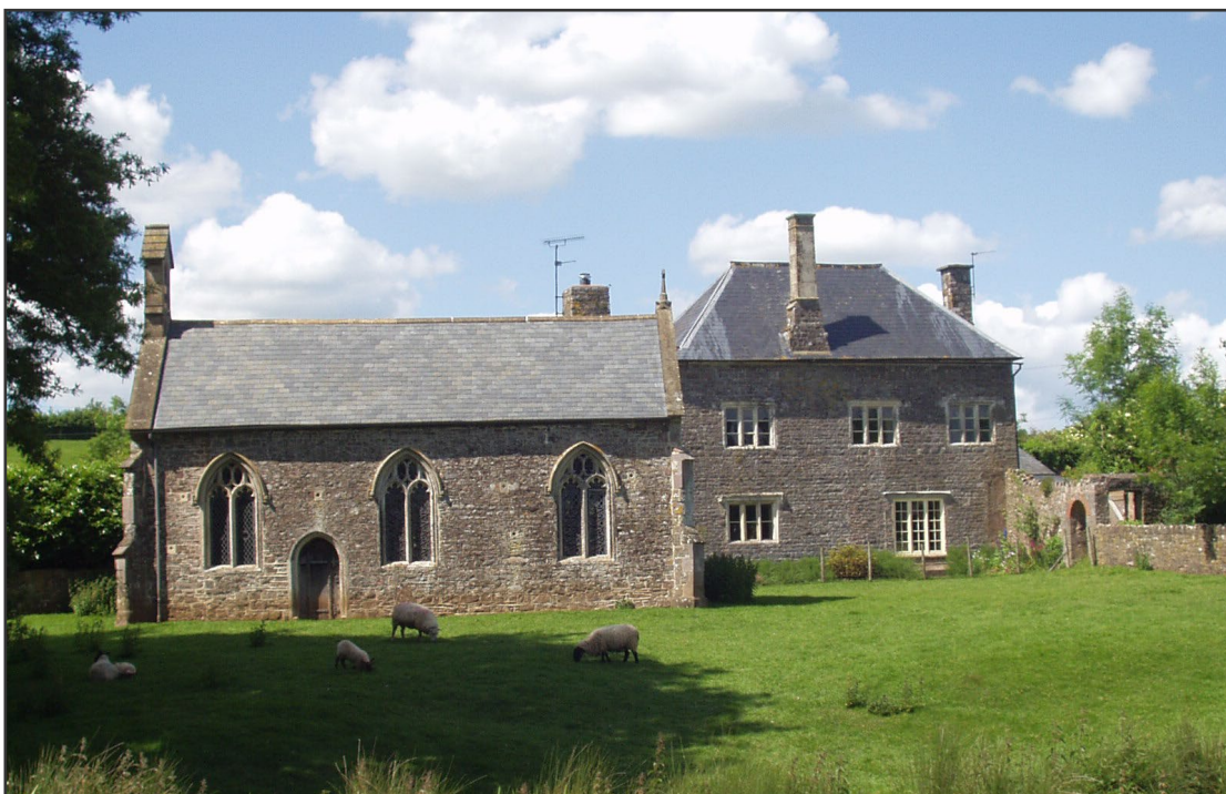
Figure 4. Ayshford Chapel with Ayshford House behind. Mainly Westleigh Limestone with some Exeter volcanics and breccia from Sampford Peverell. Beer Stone dressings around the windows are repaired with Doulling Stone.
