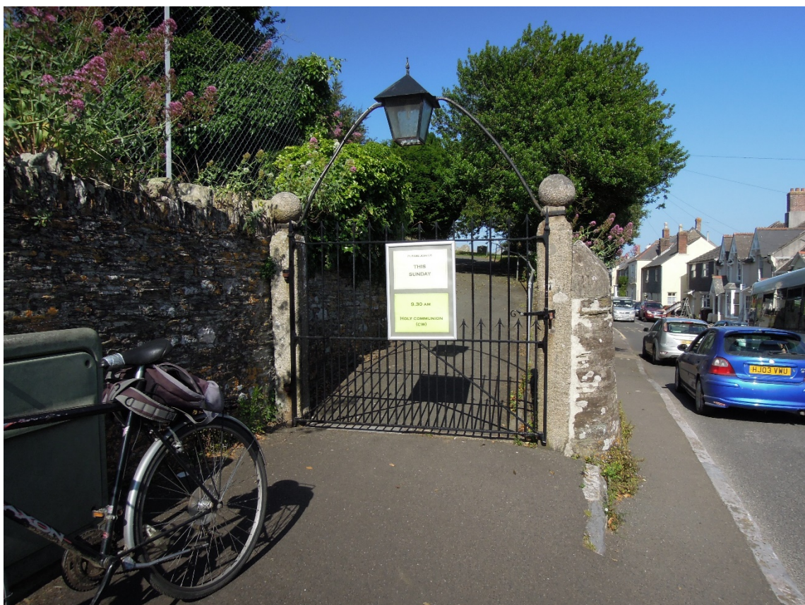
Figure 24. Shaped granite monolith gateposts at entrance to the churchyard, West Alvington.
