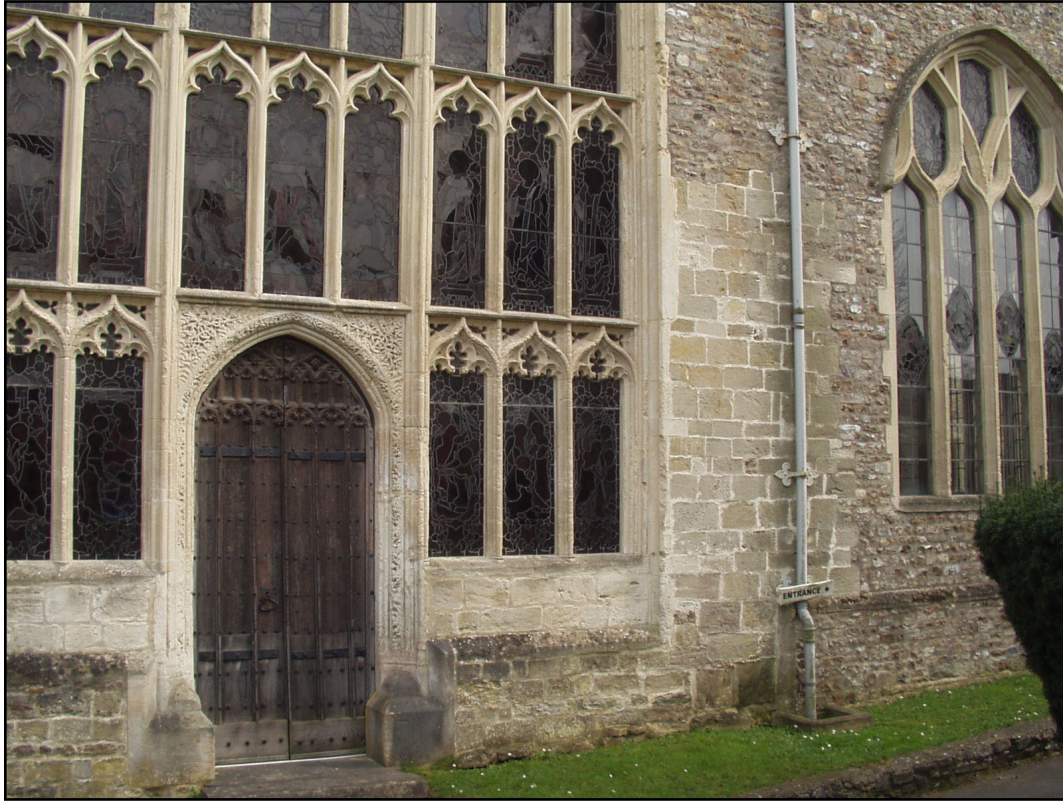
Figure 9. Beer Stone tracery at the west end of the nave of St Andrew's church, Colyton. The slightly darker blocks used for the footing below the window and part of the wall on the right are believed to be from the Upper Greensand (Code 52). The west end of the south aisle on the far right is made of chert rubble.
