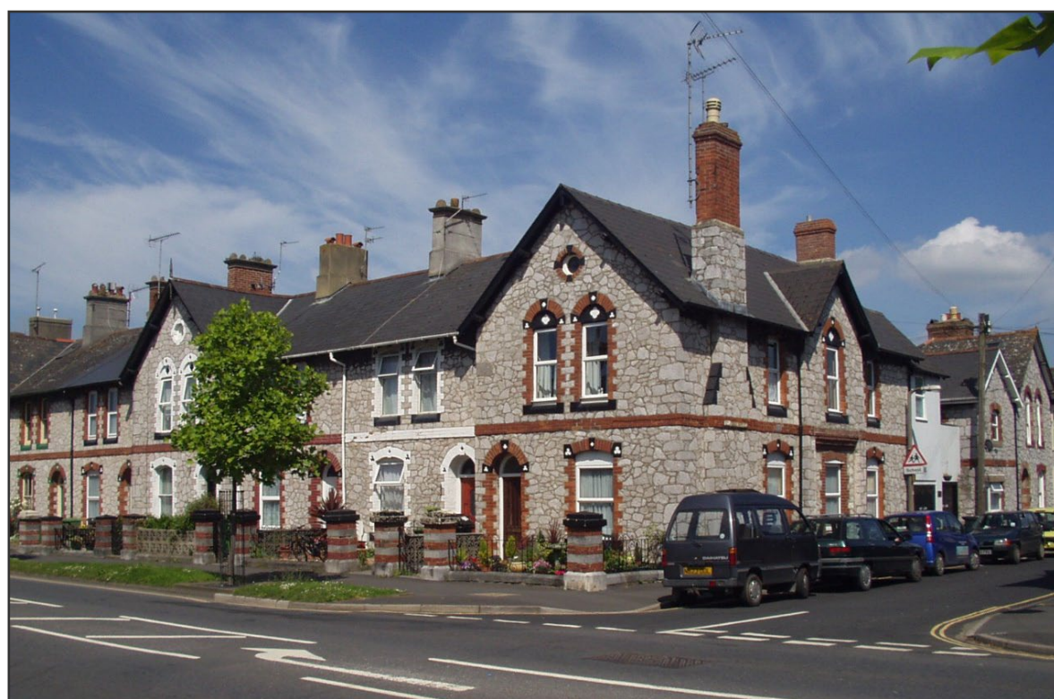
Figure 6. Pale grey limestone rubble with brick dressings, junction of The Avenue and St John's Street, Newton Abbot.
