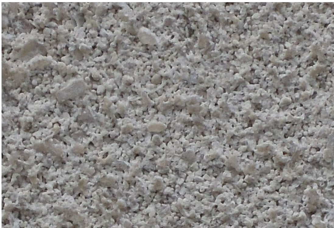
Figure 5. Lloyds Bank, High Street Exeter. The small free-standing ooliths are about 0.5mm across. They are mixed with larger shell fragments.
