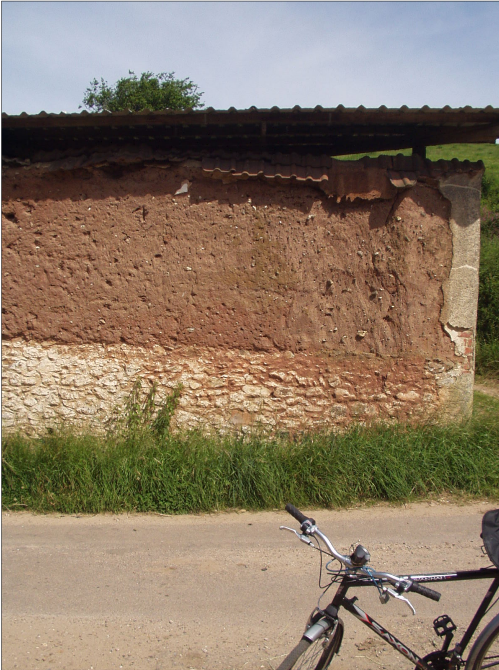
Figure 1. Outbuilding, Tipton St John. Remains of the original tile roof are visible below the new corrugated iron.
