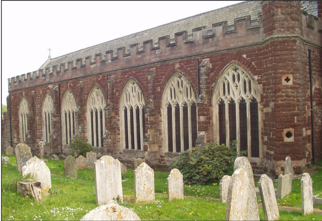
Figure 5. North aisle of All Saints church, Kenton. The wall is of mixed Heavitree Breccia, mottled fawn and red sandstone, probably from the Dawlish Sandstone, and minor calcareous sandstone from the Upper Greensand, probably from Salcombe Regis. The superb window arcade is dressed with Beer Stone.
