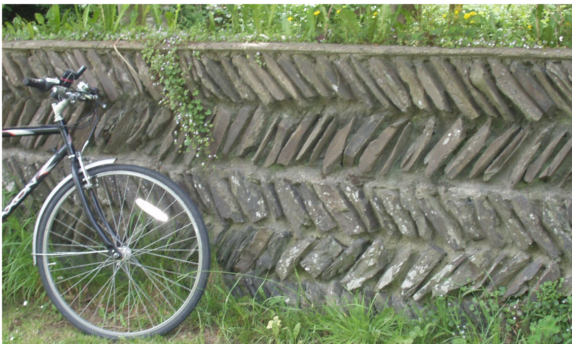
Figure 2. Thin concrete coping to a roadside wall of Pickwell Down sandstone, Foxhunters Inn, West Down.
