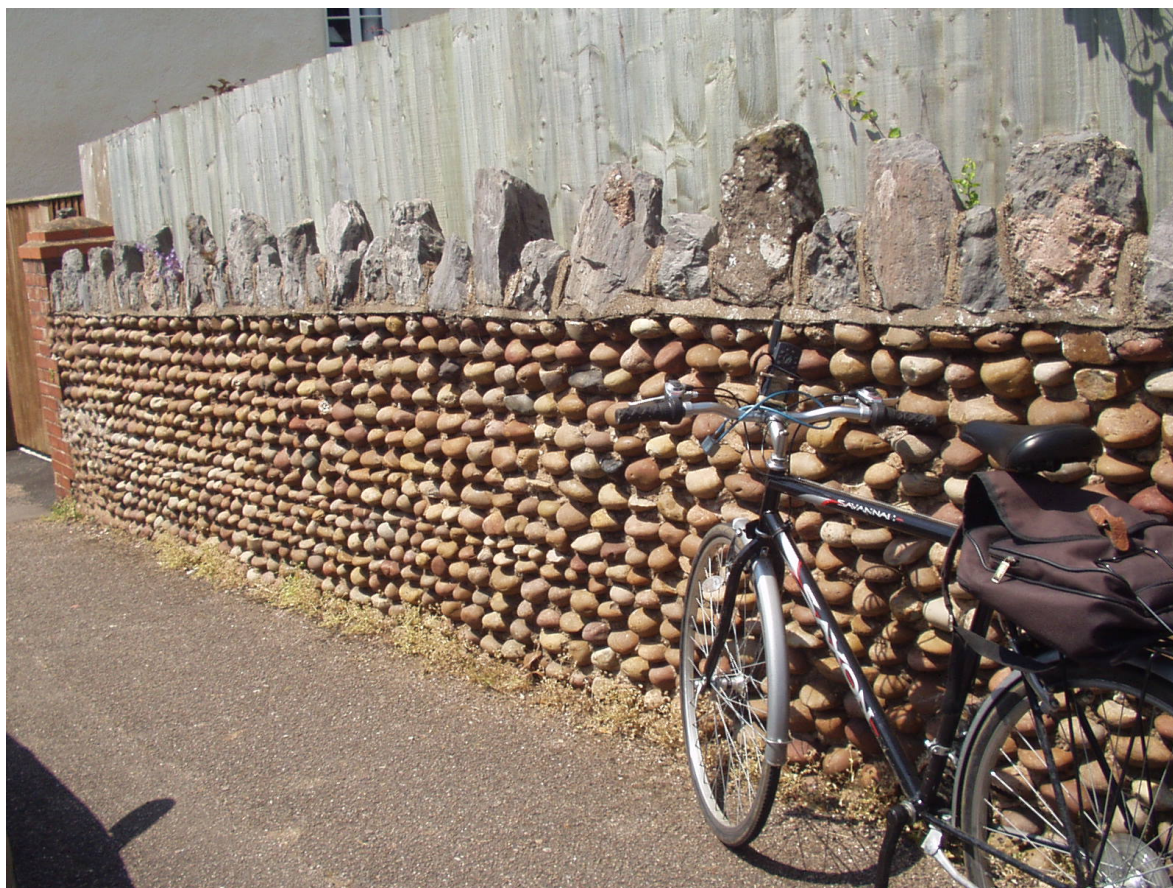
Figure 4. Decorative finish of sized “Budleigh Buns”. North side of Flower Street, Woodbury. The coping is of grey Torbay limestone.
