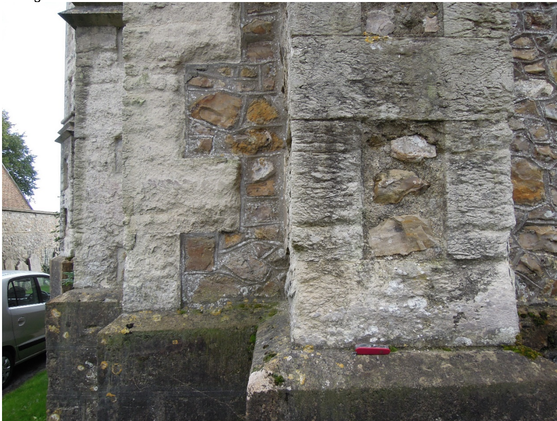
Figure 7. North aisle of St Andrew's church, Charmouth. Badly weathered Beer Stone used for the quoins and buttresses.
