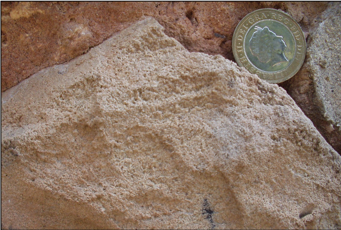
Figure 5. Ruined outbuilding near Kentisbeare. Fawn glauconitic sandstone showing characteristic rough-weathered porous surface texture and flat facets believed to record the original cleaving of the rock when first extracted in a soft state.
