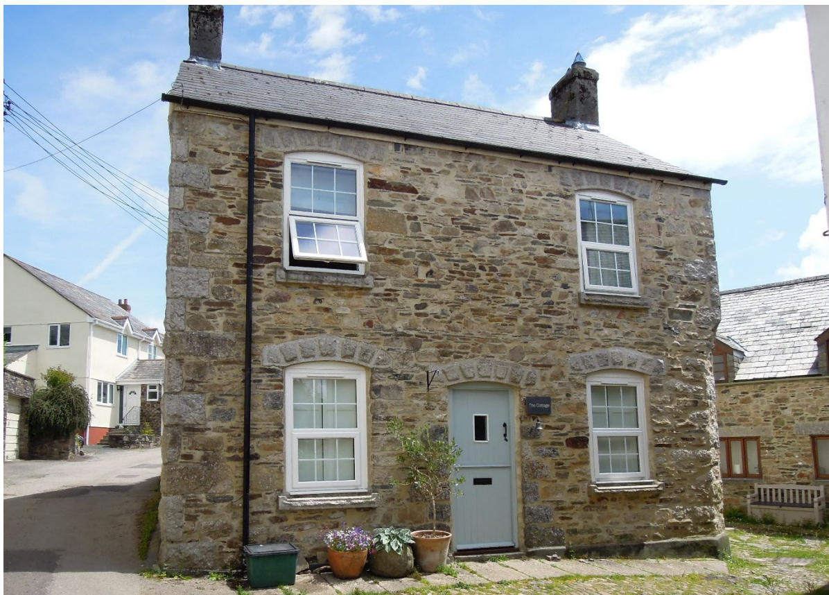
Figure 27. The Cottage, Walkhampton. The walls are of microgranite and spotted slate. The quoins and lintels are of granite. The lintels are each made of a single stone carved to look like relieving arches.
