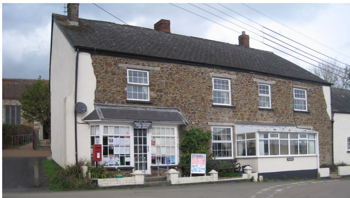
Figure 1. Post Office and stores, Black Torrington. Concrete lintels to ground and first floor windows.
