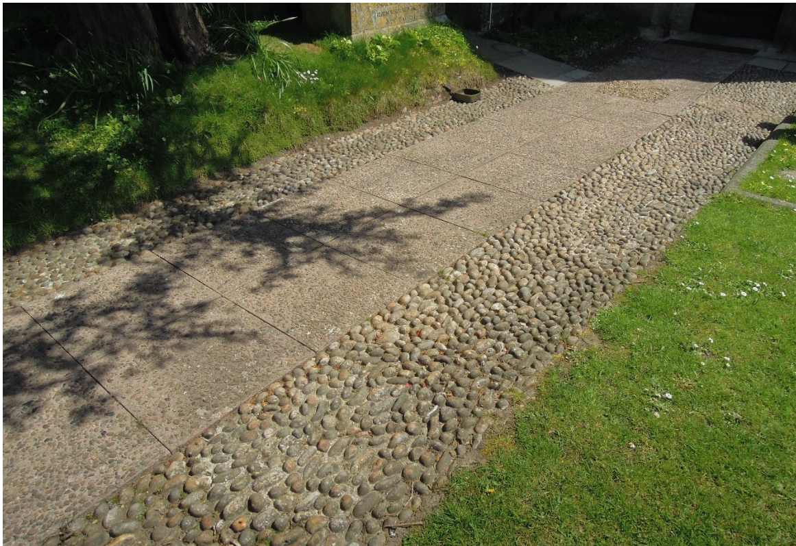
Figure 7. Rounded chert cobbles used as decorative edging to access path, Salcombe Regis church.
