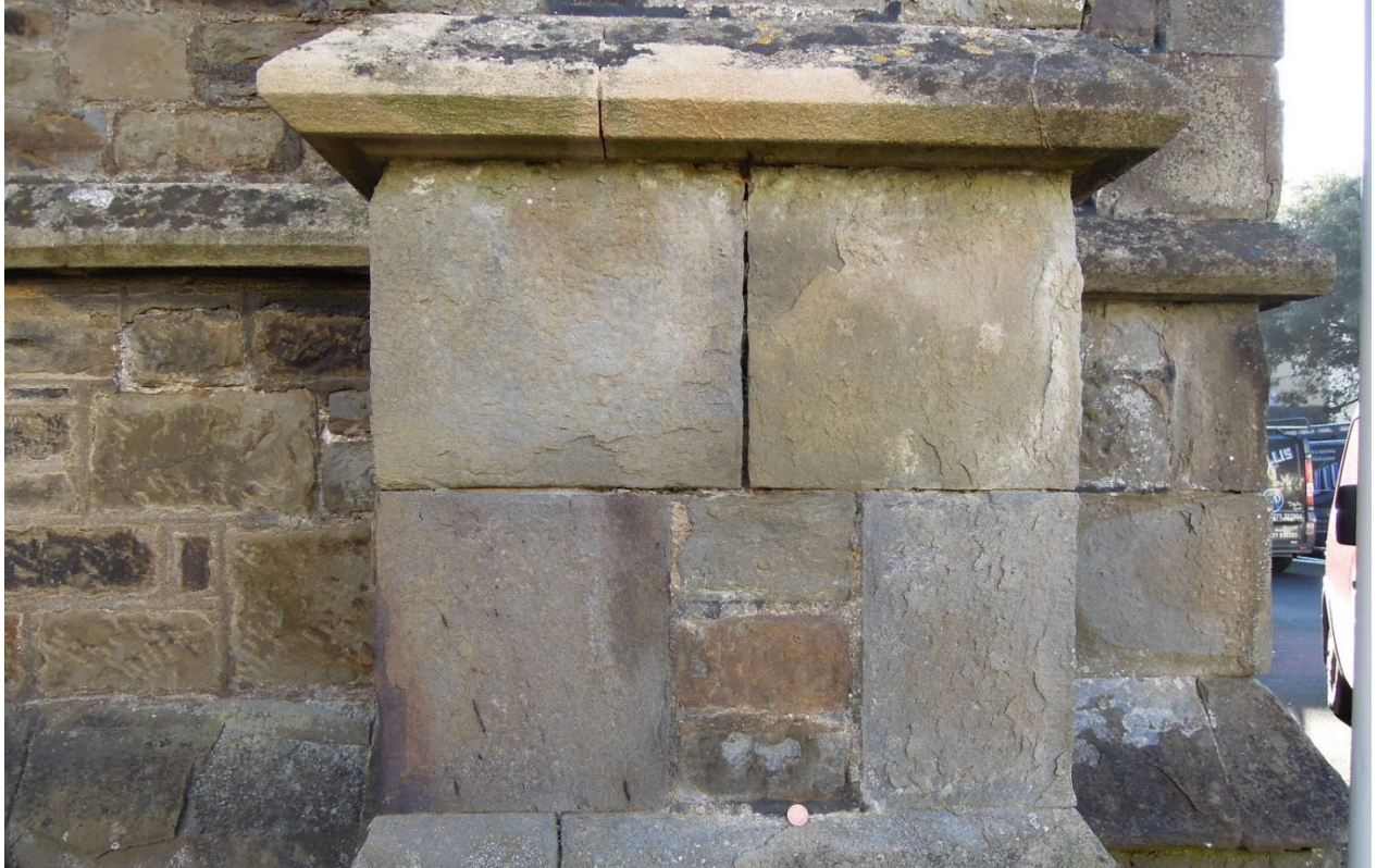
Figure 3. St Phillip and St James' church, Ilfracombe. The buff colour and large size of the sandstone blocks are typical of some stone from the Ilfracombe Formation.
