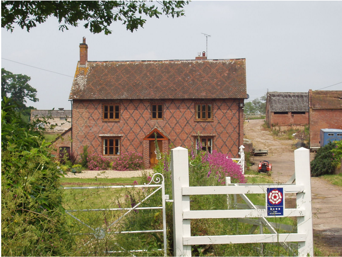
Figure 2. Street Raleigh Farm, Street Raleigh. Lintels and window frames are all made of hardwood.
