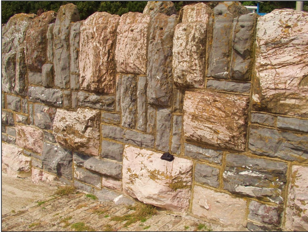
Figure 9. Pale grey limestone with pink cast and medium grey limestone, sea wall, Meadfoot Sea Road, Torquay.
