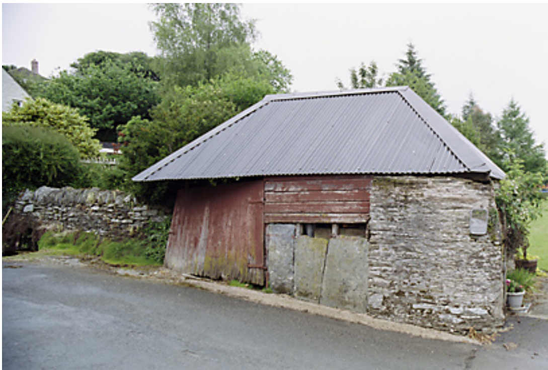
Figure 1. Tumbledown outbuilding, Ledstone Farm near Buckland Tout-Saints with new corrugated iron roof. The walls are made of stone rubble, stone slabs set on end and boards. Photo © Mr Stuart Brighton.
