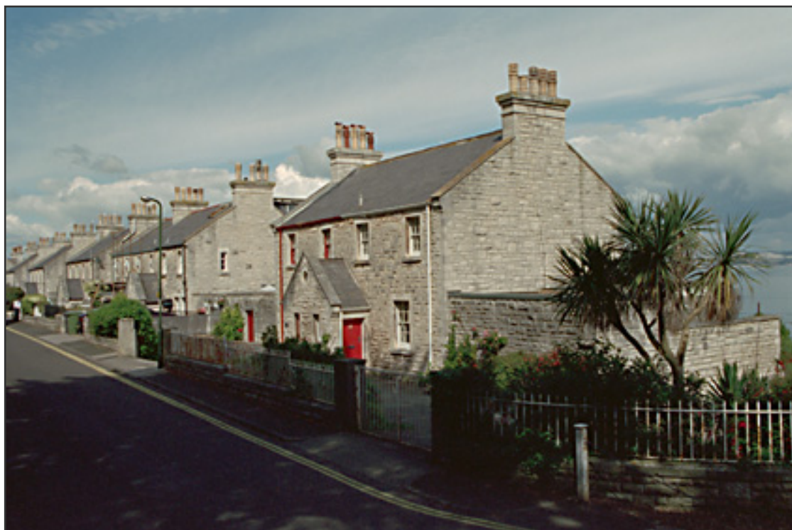
Figure 4. 14-32 Berry Head Road, Brixham. Photo © Mr Dennis Coote CPAGB APAGB. Built originally for the coastguard. The listed building citation says they are of local limestone but in fact they are of Portland Stone.
