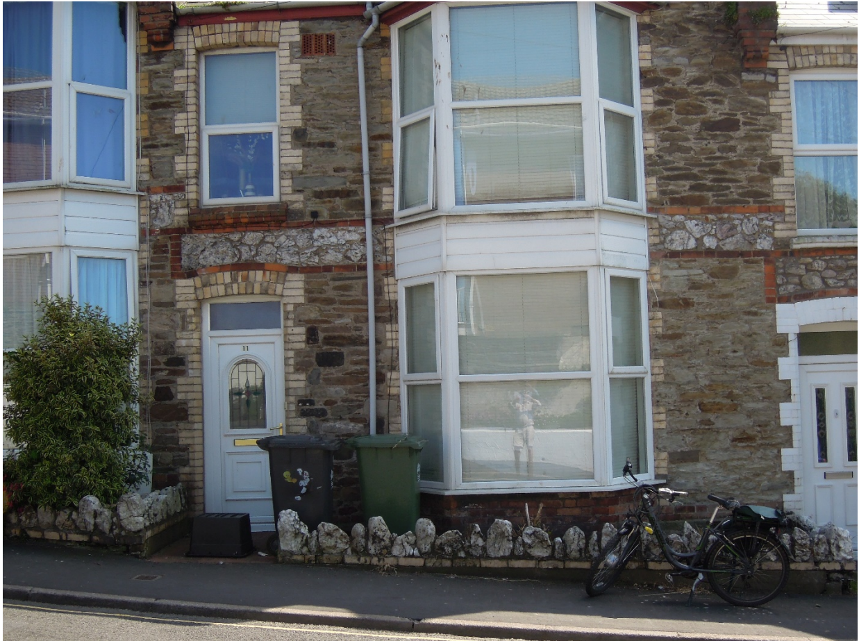
Figure 4. No 11 Malborough Road, Ilfracombe. Vein quartz used as a decorative band above the first floor of the house and as edging to the front border.
