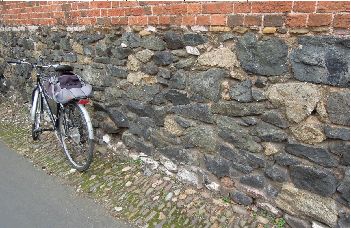
Figure 2. Roadside wall, Monmouth Hill, Topsham. Hornblende gabbro (dark blue) with subordinate biotite gneiss (pale grey).
