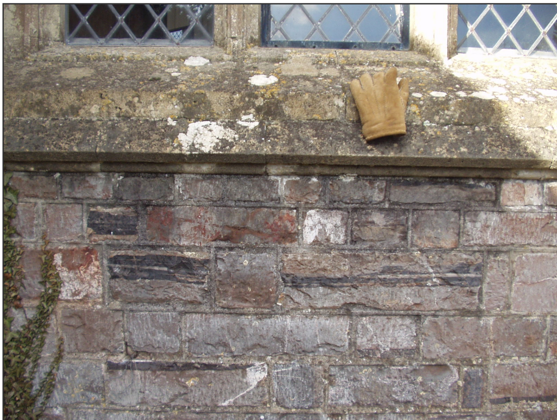
Figure 1. St Mary's, Uffculme. Dark grey limestone with black chert bands.
