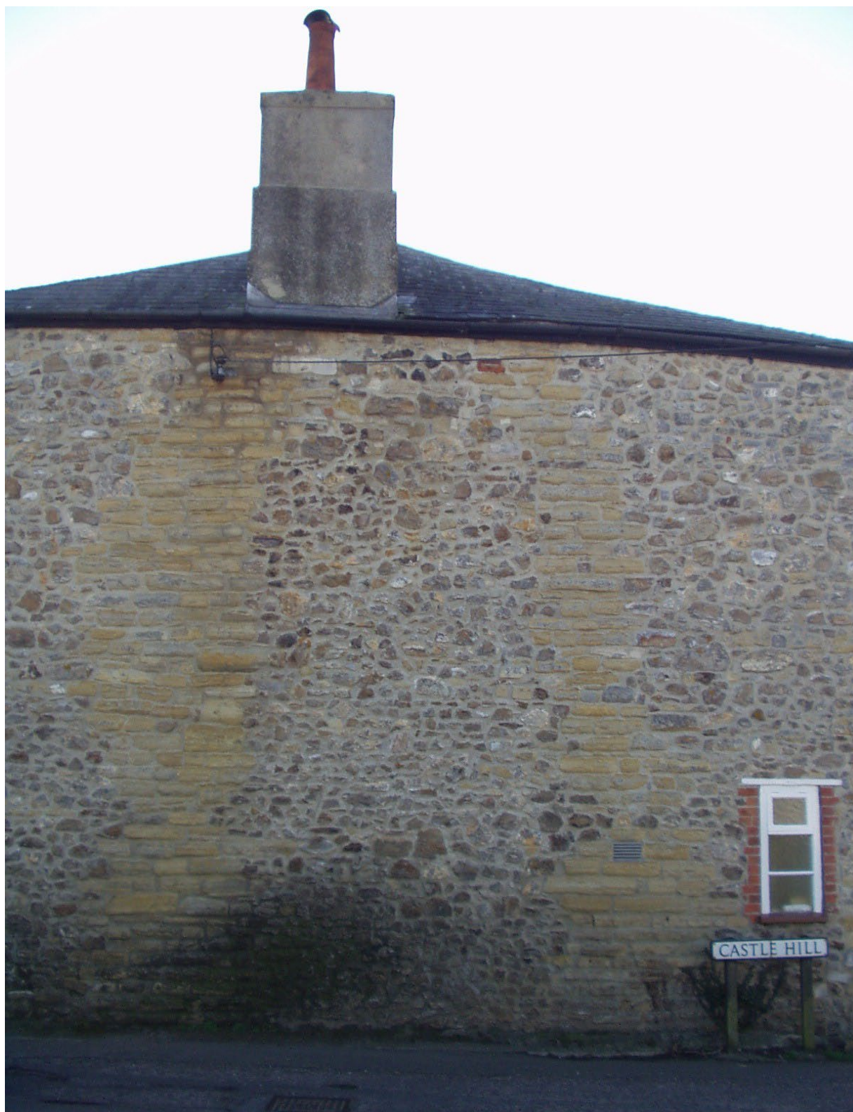
Figure 20. The Old Farmhouse, Castle Hill, Axminster. The gable end is mainly of chert but the flues are lined with yellow Blue Lias limestone. There is only one chimney pot so one or perhaps both chimneys may be blocked up.
