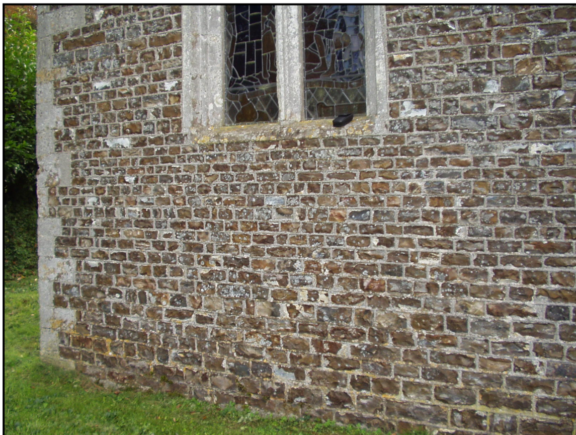
Figure 9. Church of St Peter and St Paul, Churchstanton. Coursed rubble of shaped chert blocks. Quoins of Upper Greensand sandstone, dressings of Beer Stone.
