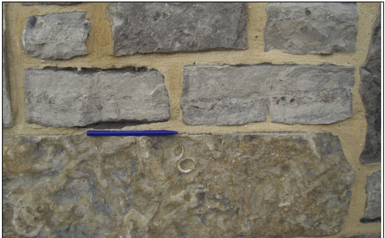
Figure 4. Wall of Lifeboat Station, Lyme Regis. The block below the pen shows bivalve shells and worm tracks. The stone is from Tout Quarry, South Somerset.
