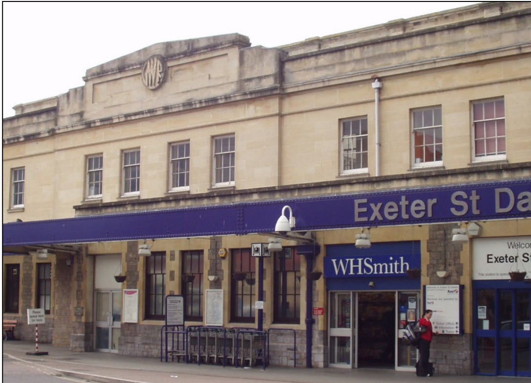
Figure 4. St David's railway station, Exeter. The lower storey is of Westleigh Limestone; the upper storey, and most quoins and dressings are of Bath Stone.
