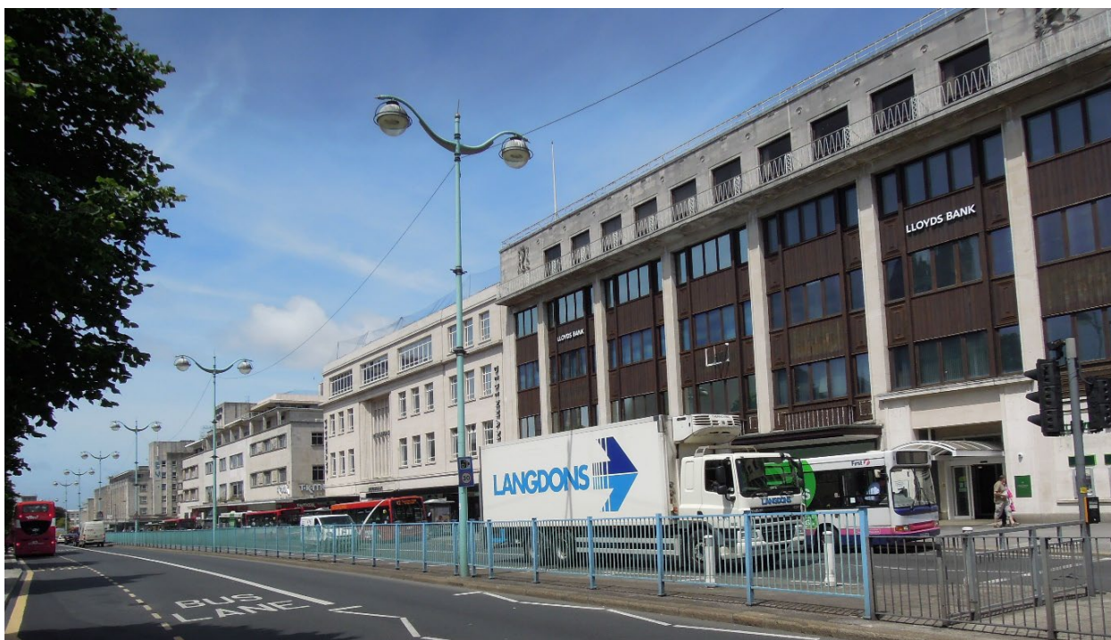
Figure 4. Lloyds Bank, Plymouth. The façade is made of Portland Stone with stained wooden panels.
