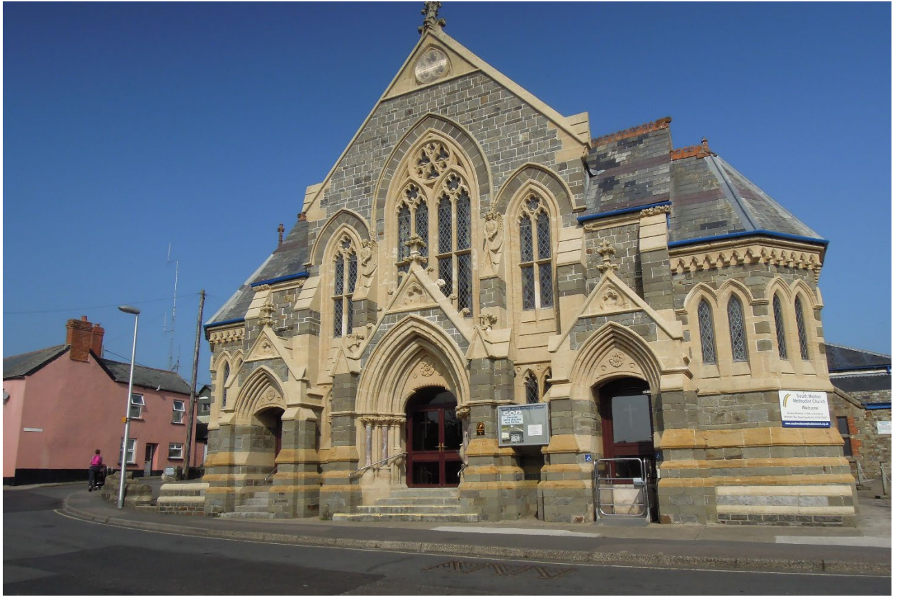
Figure 6. Methodist church, South Molton. The pale yellow dressings are of Doultong Stone. The darker yellow string courses towards the bottom of the façade are of Ham Hill Stone. The little pillars each side of the main doorway are of Devon Marble. The rest of the wall is of grey middle-Devonian limestone.
