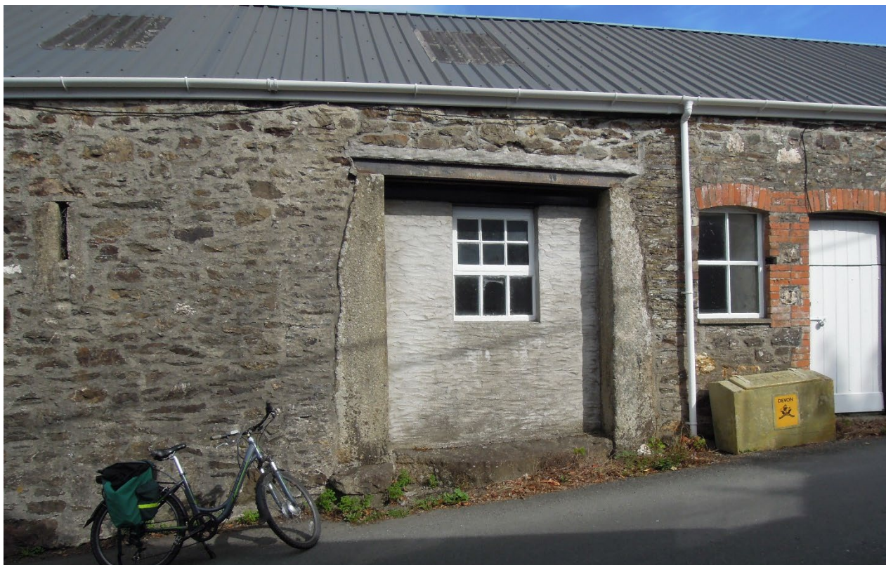
Figure 19. Jambs of former double doors made of single prisms of granite. Outbuilding, 100m west of St Andrew's church, Tavistock.
