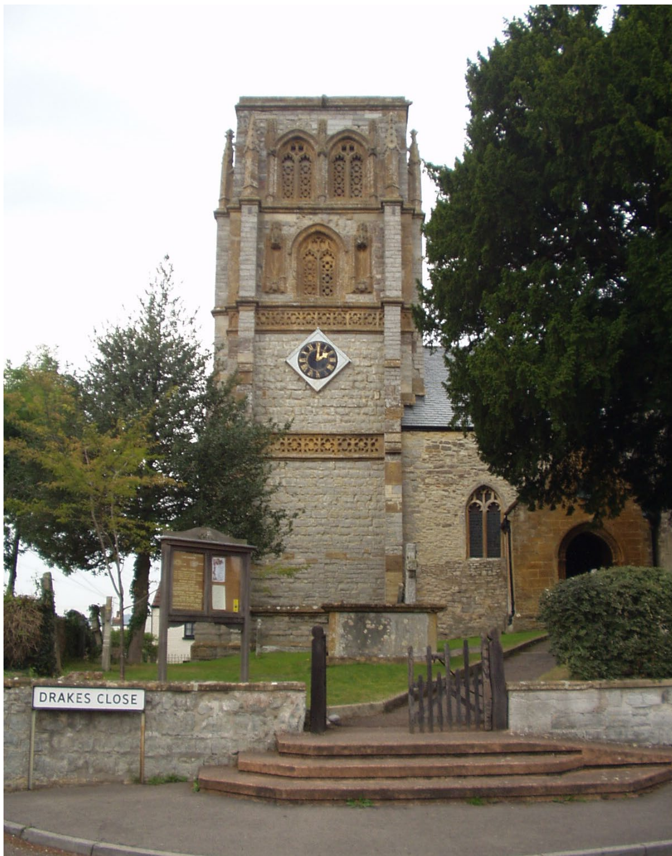
Figure 17. Tower of St George's church, Ruishton, of Blue Lias limestone with dressings of Ham Hill Stone.
