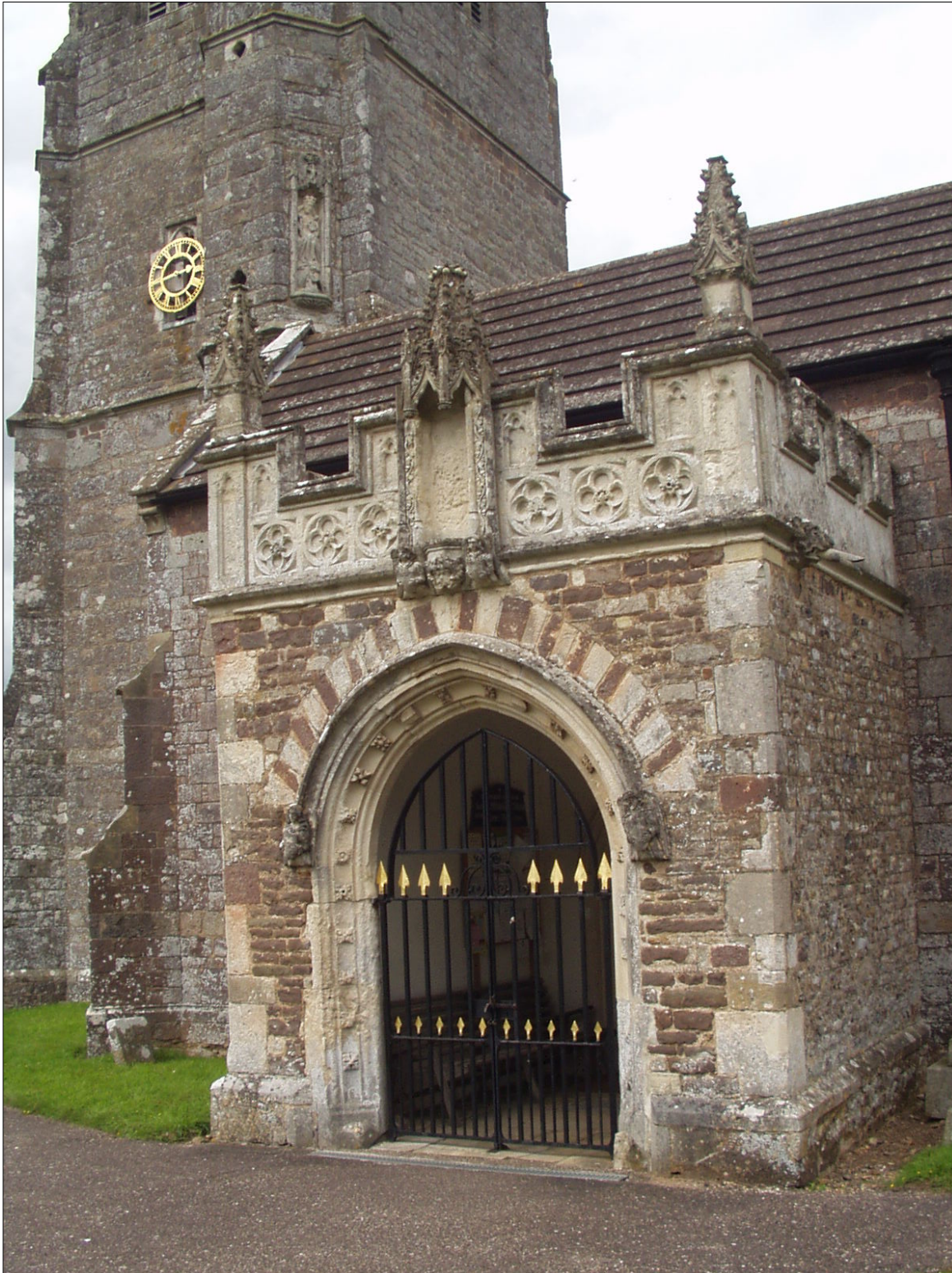
Figure 11. Porch of St James the Great, Talaton. Beer Stone is used for the carved dressings round the door, the parapet and, alternating with purple lava, for the relieving arch over the door. The quoins are mainly of calcareous sandstone from the Upper Greensand and the wall material is mainly maroon sandstone of the Bude Formation.
