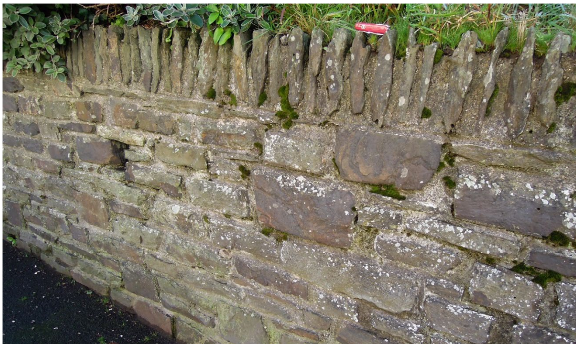
Figure 1. Grey sandstone (Code 96) probably from the Ilfracombe Formation. The coping is of slate, likely from the same source. South side of Portland Street, Ilfracombe.
