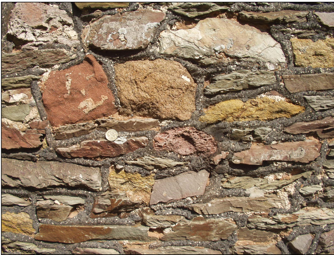
Figure 3. St Mary's, Cheddon Fitzpaine. The red and yellow building blocks are of Otter Sandstone and Ham Hill Stone respectively. The balance are of Morte slate, some laid with cleavage parallel to the plane of the wall.
