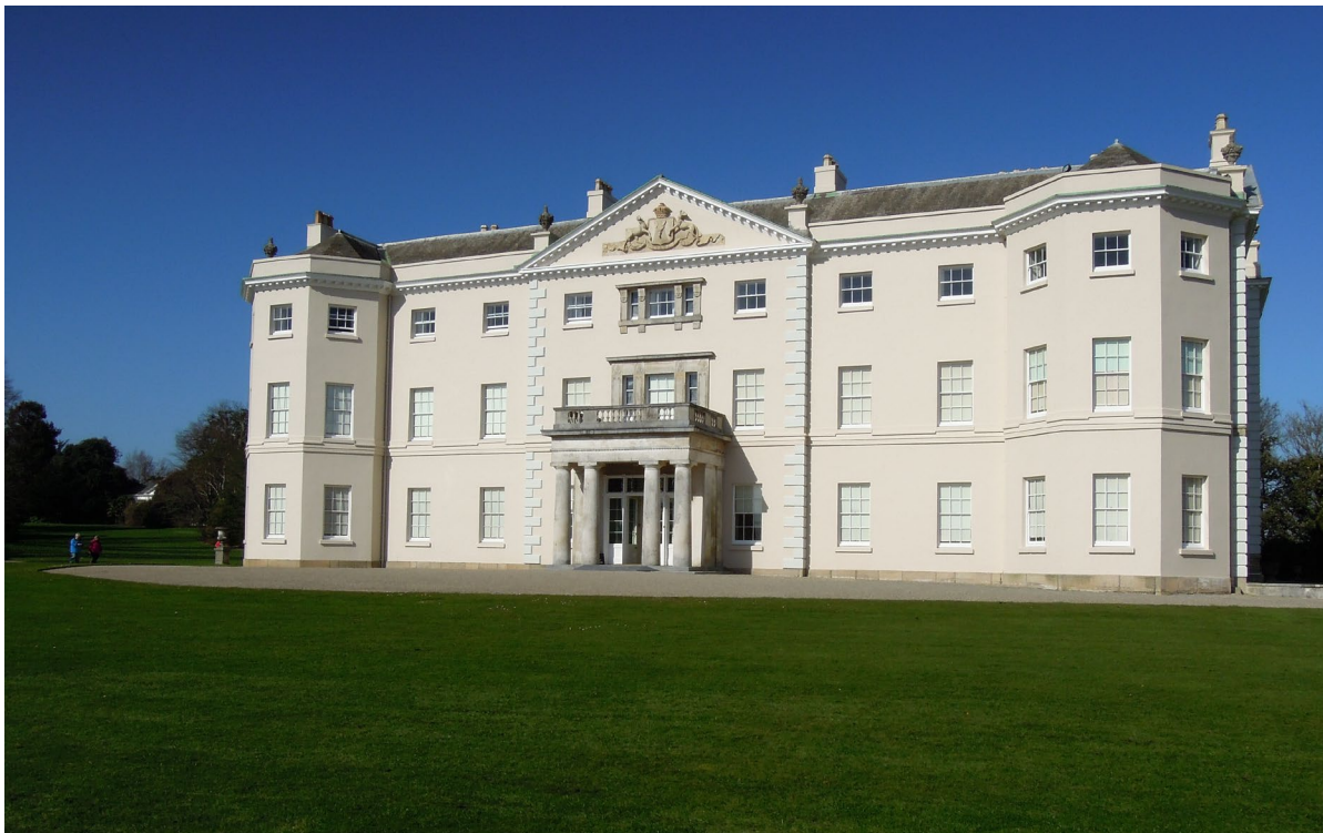
Figure 9. Saltram House, Plymouth. The south façade is finished in stucco on a footing of granite. The dressings of the portico are of Portland Stone.
