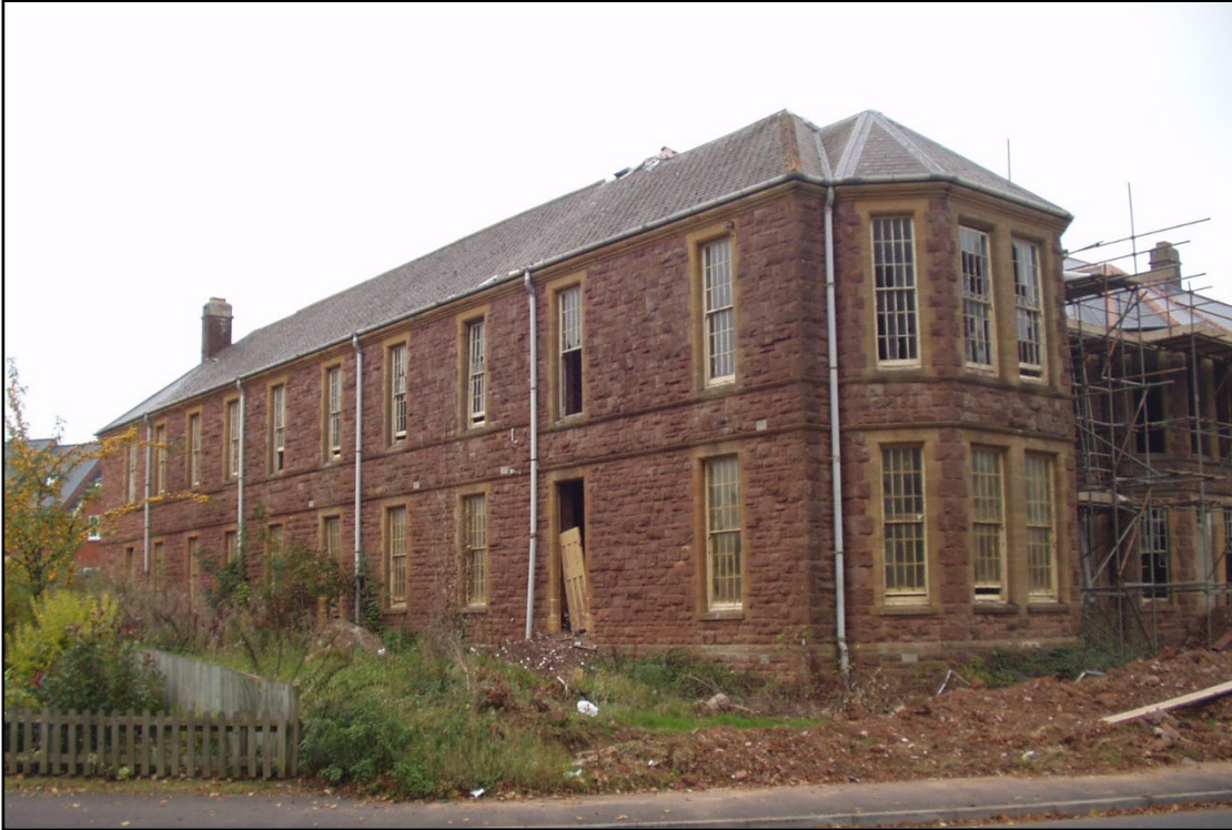
Figure 4. Former hospital block in course of renovation, Cotford St Luke. Red Otter Sandstone from Bishop's Lydeard quarry. Dressings of Ham Hill Stone.
