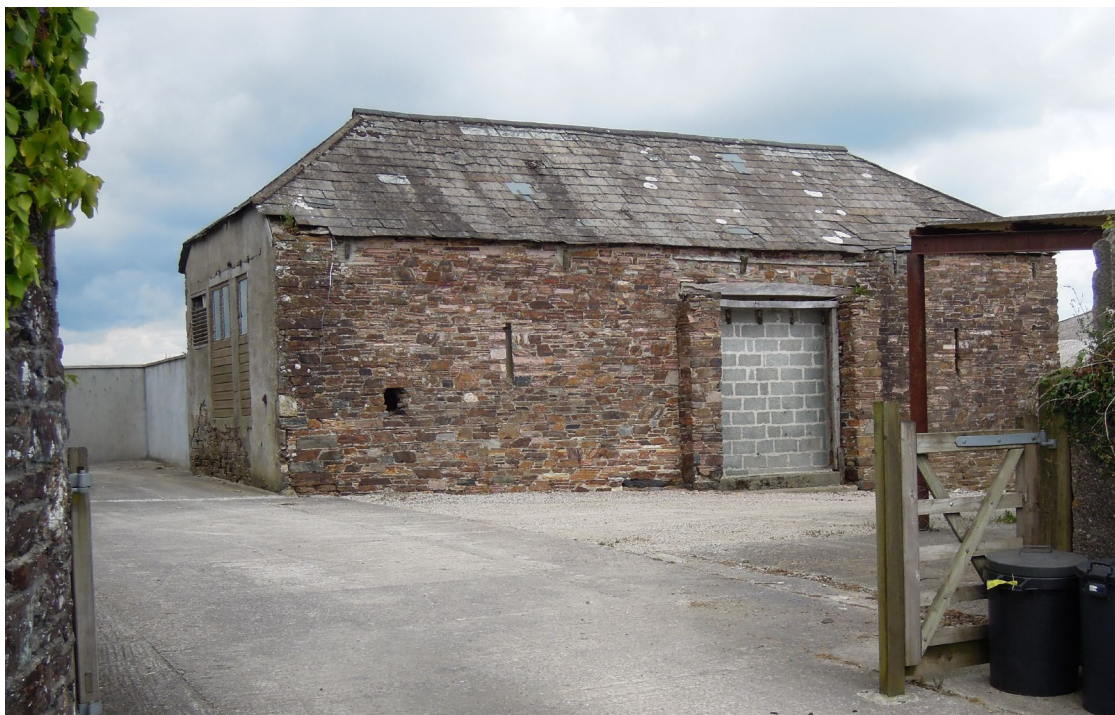
Figure 4. Outbuilding of Router Farm between Lifton and Chillaton, of Codden Hill Chert with doorway filled by concrete blocks.
