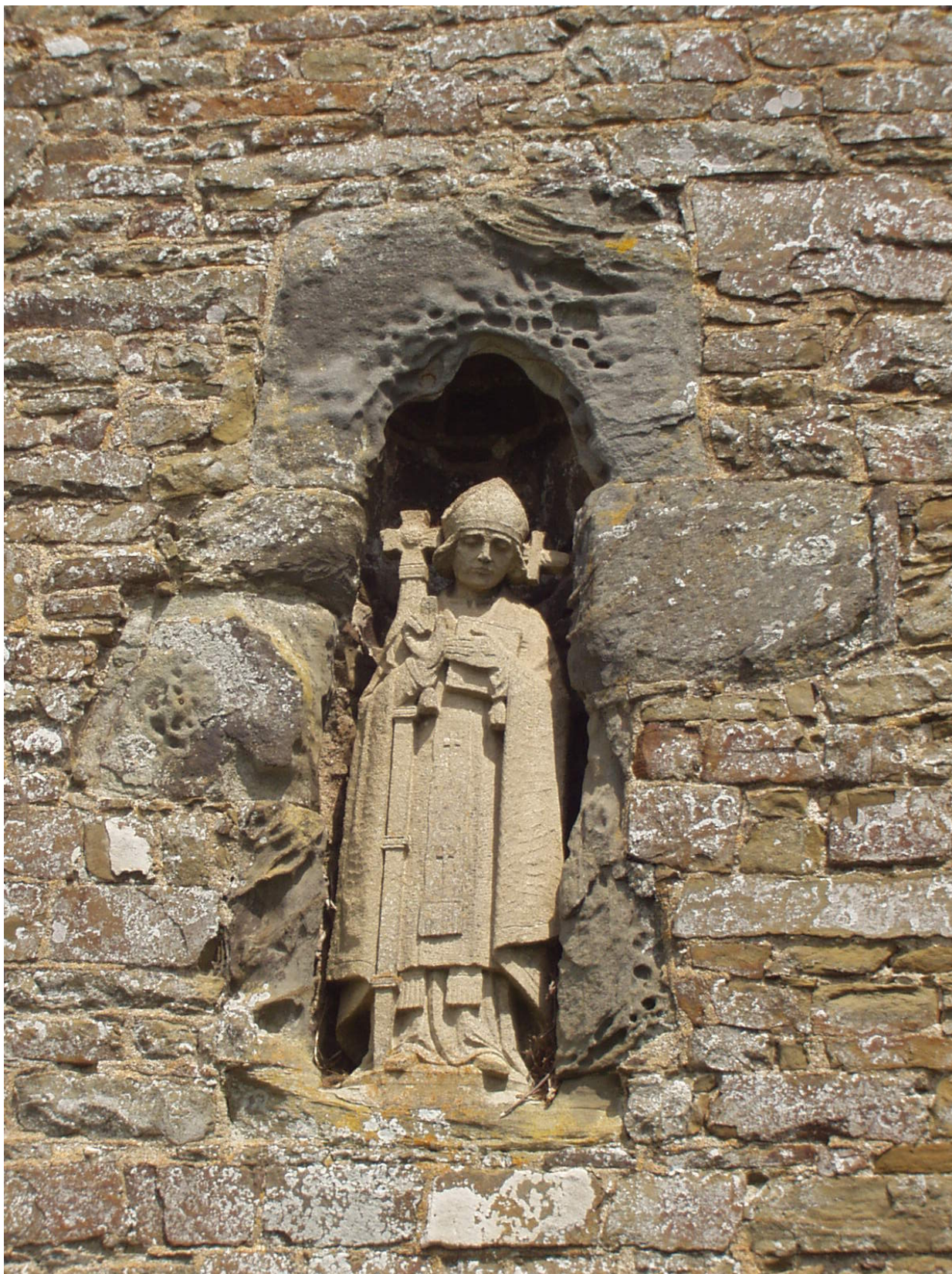
Figure 9. Large blocks of Pickwell Down sandstone lining the niche for a statue, Tower of St Thomas of Canterbury's church, Lapford. The rest of the wall is made of sandstone from the Bude Formation.
