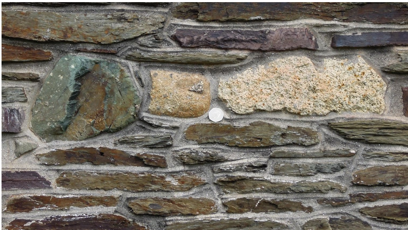
Figure 6. Green-blue block of amphibolite with visible white plagioclase phenocrysts (centre left), pale yellow quartz porphyry and dark hued slate, south transept of St Peter and St Paul's church, Ermington.
