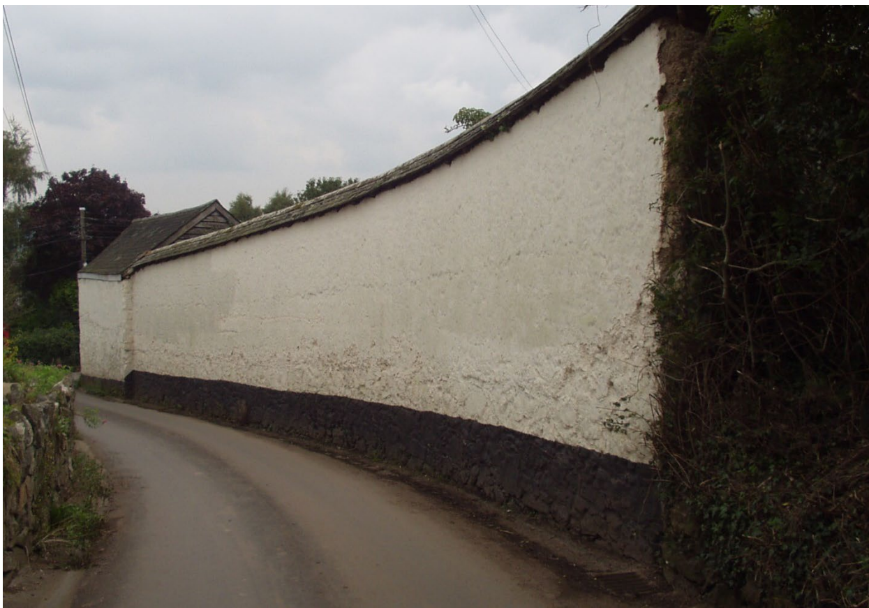
Figure 2. Painted cob on painted stone rubble footing with slate coping. Bottom of Commons Hill, close to junction with Dry Lane, Christow.
