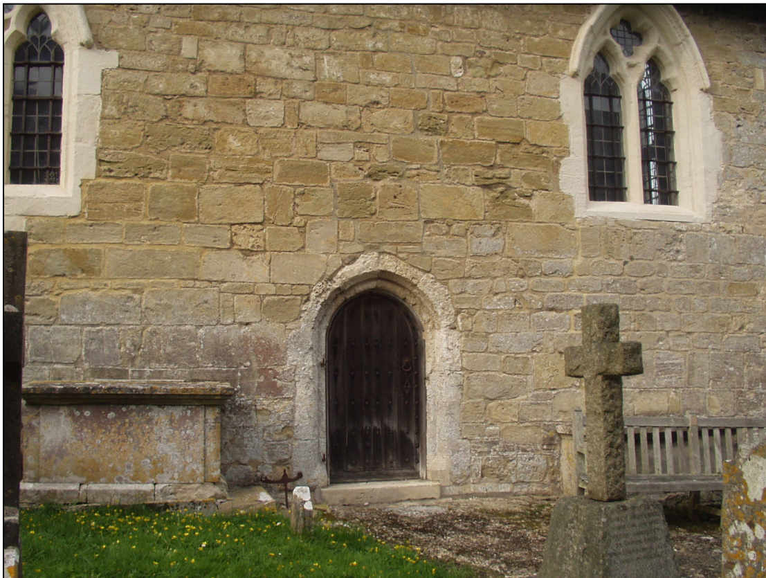
Figure 1. St Winifred's, Branscombe, south wall of chancel. Brown Salcombe stone weathered grey with red algae towards the base. Dressings are of Beer Stone, partly preserved with white paint.
