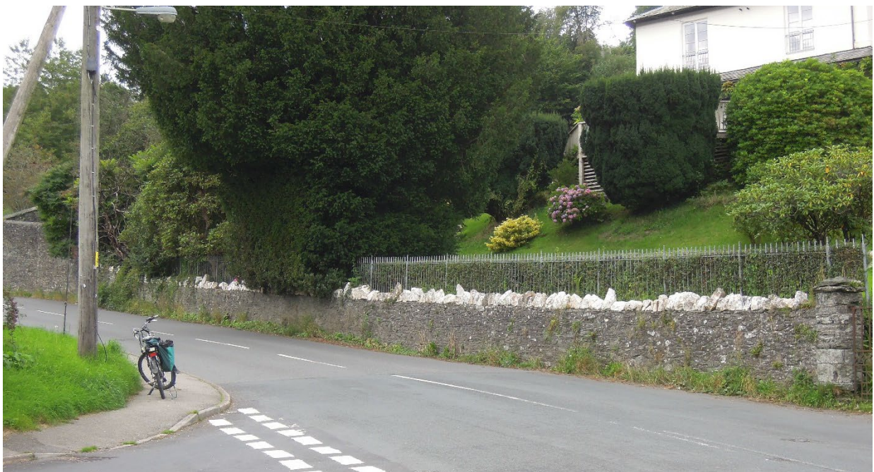
Figure 5. Vein quartz coping of the wall in front of Rosebank, Bannawell Street, Tavistock.
