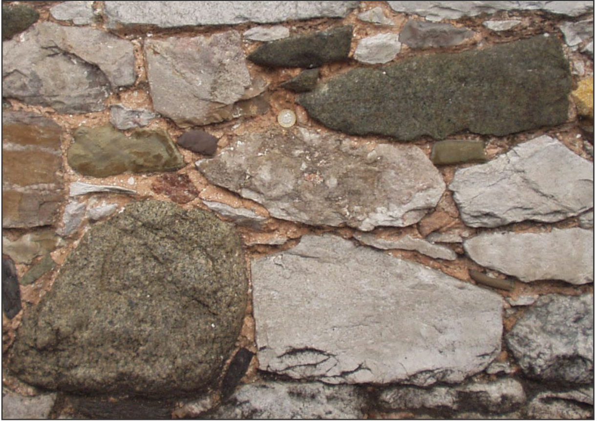
Figure 1. Garden wall, Woodlands, Globefields, Topsham. Grey and dark green-grey blocks of basic igneous rock in a wall mainly of pale grey limestone imported from Torbay.
