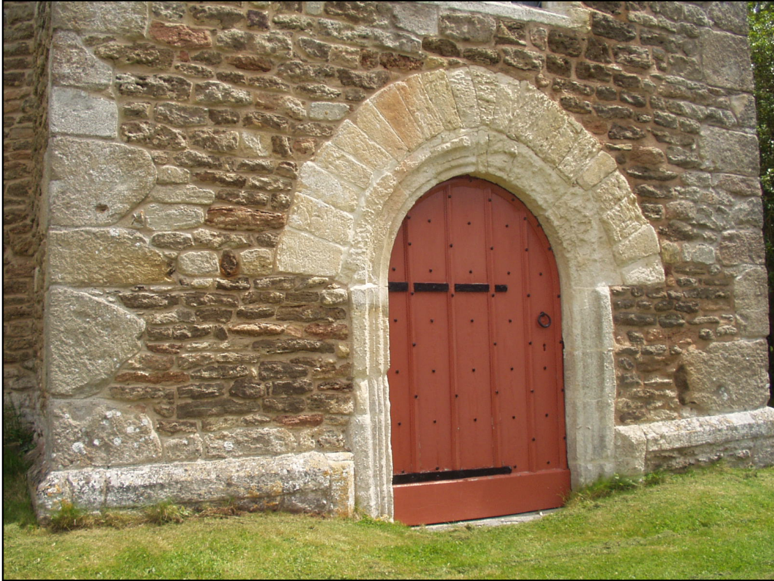
Figure 1. Tower of St Gregory's church, Harpford. Beer Stone dressings round the west door; mainly Upper Greensand sandstone with some Beer stone used for the quoins and mud pebble conglomerate from the Otter Sandstone used for the walls.
