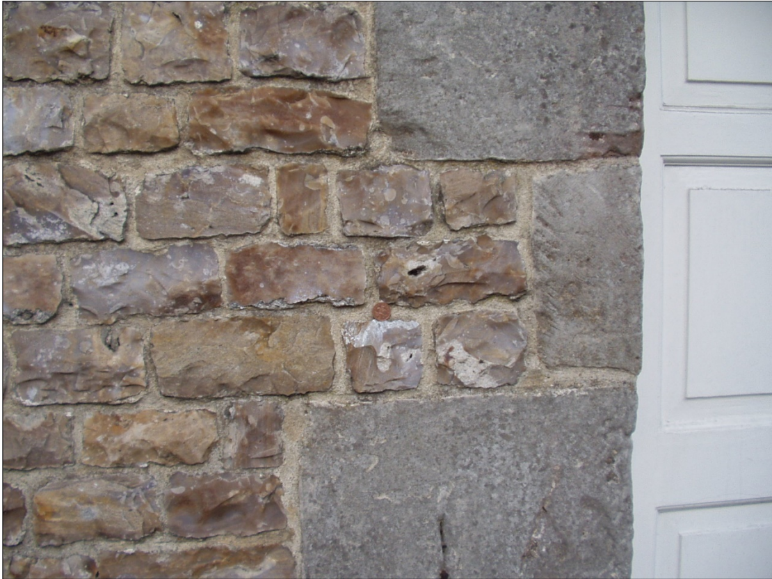
Figure 3. Chard Museum. Wall of dressed chert laid in courses with quoins of grey calcareous sandstone.
