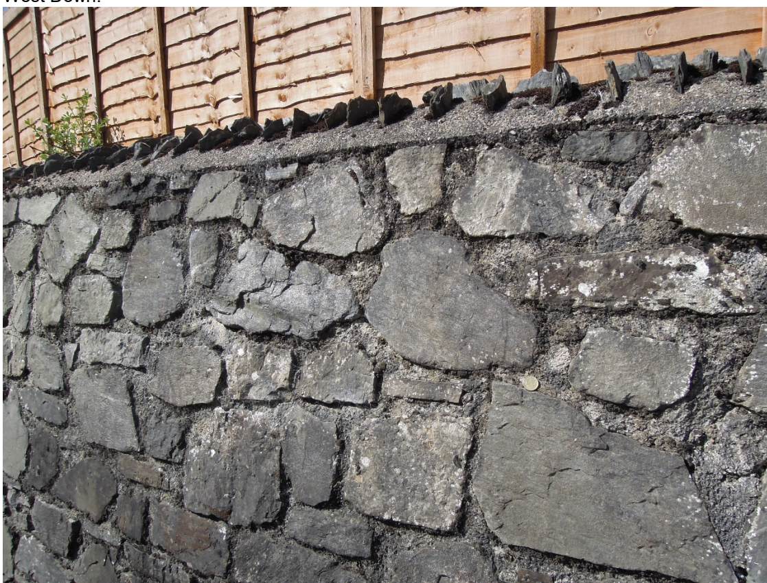
Figure 3. Rounded concrete capping with sharp slate inserts on top of a wall of Pilton Formation sandstone, George Nympton Road near junction with South Street, South Molton.
