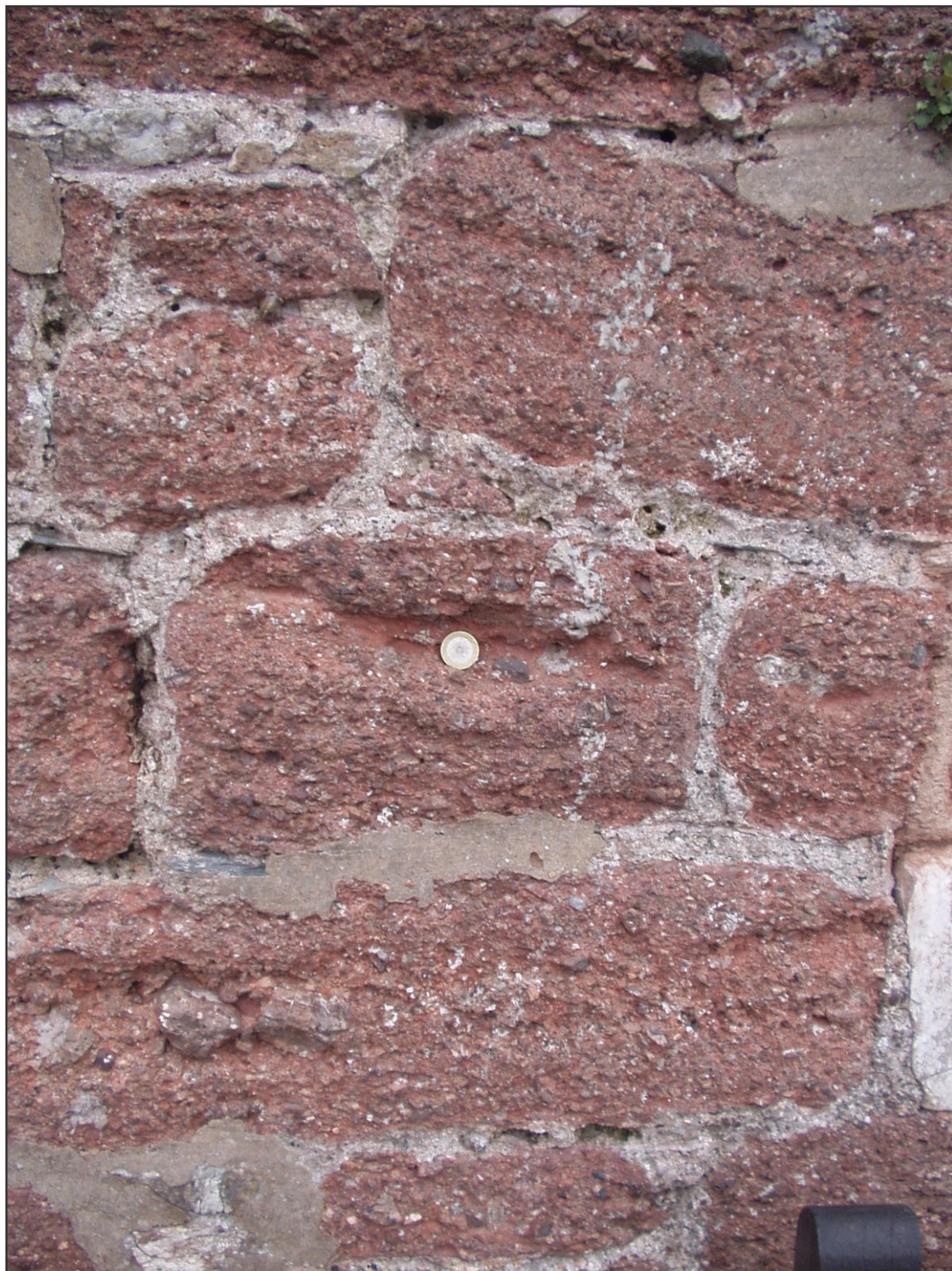
Figure 10. Embankment, Ferry Road, Topsham. Note two large fragments of purple volcanic rock in the breccia towards the lower left corner of the photo.
