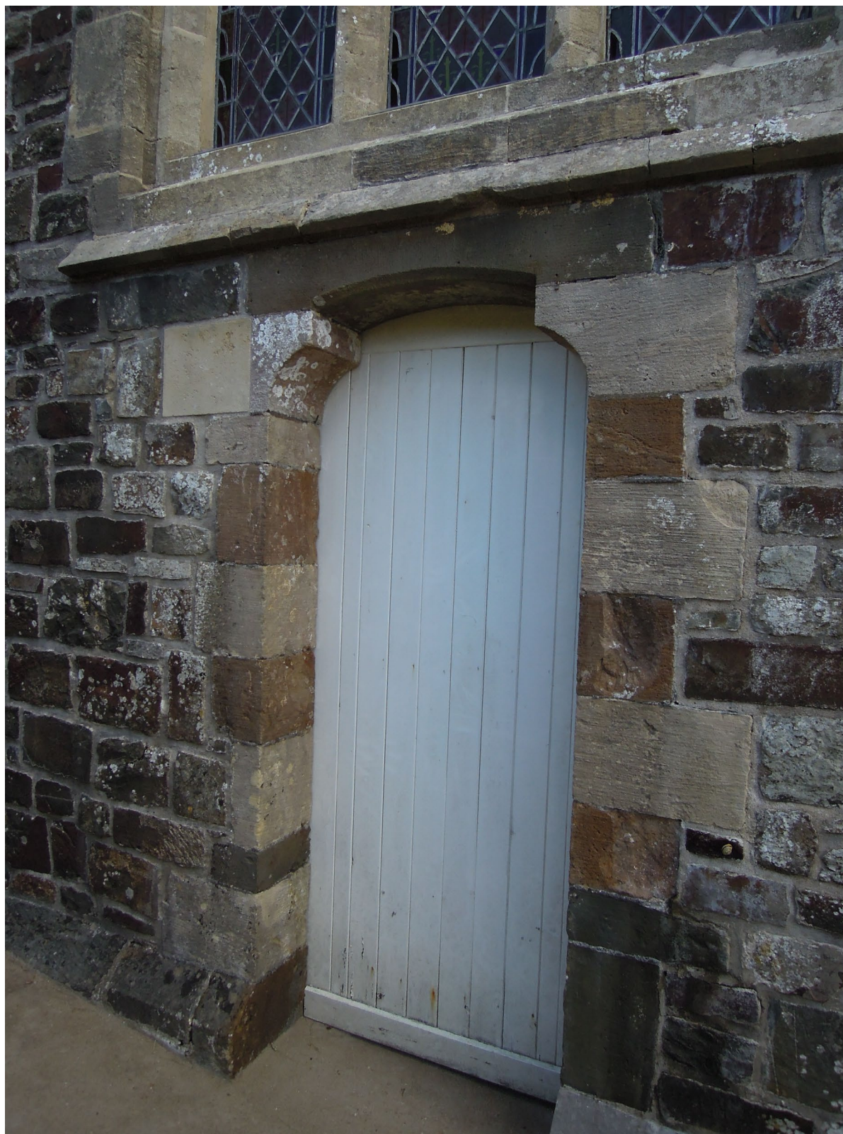
Figure 8. West door, parish church, Langtree. The doorway dressings are of alternating Douling Stone (pale) and Hatherleigh Stone (dark brown). The wall is otherwise made of very dark-stained sandstone believed to be from the Bude Formation.
