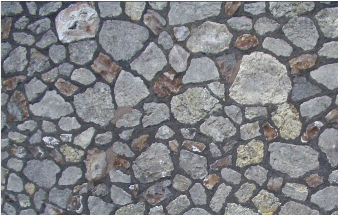
Figure 2. Detail of 22 Boden Street, Chard. Rubble of pale grey calcareous sandstone and some brown chert. Width of view about 60cms.
