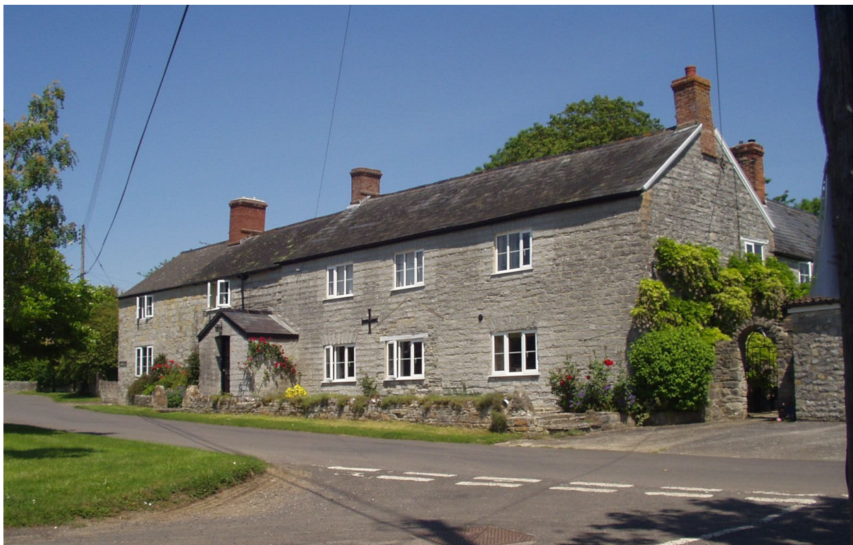
Figure 5. Allens, Beercrocombe. The walls, quoins and dressings are all of Blue Lias limestone with some concrete sills.
