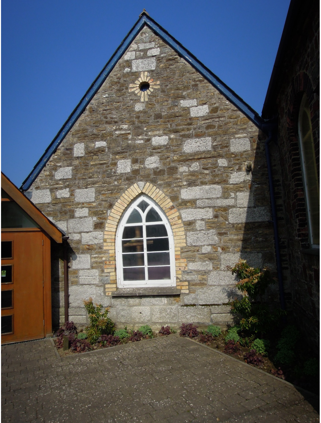
Figure 5. Back of the Methodist chapel, Old School Lane, Fremington. The wall is of pale grey granite without phenocrysts probably from Lundy, and Codden Hill Chert.
