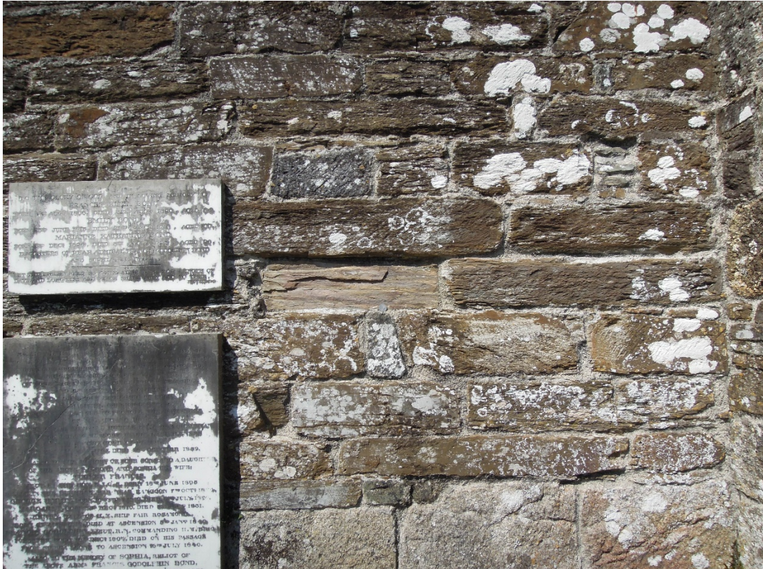
Figure 4. Good quality brown slate as regular blocks. Tower of St Peter's church, Lewdon.
