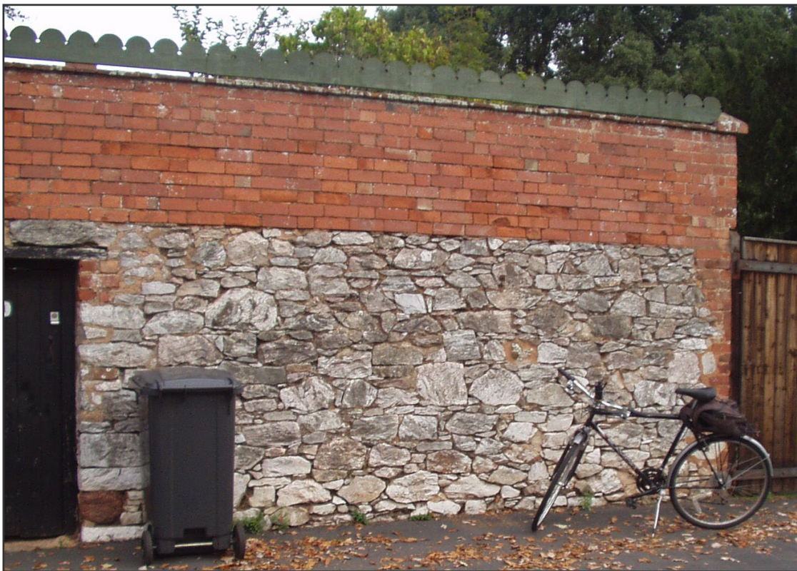
Figure 2. Woodlands, Globefields, Topsham. Pale grey limestone with some blocks of granite and dolerite below and brick above. This is the typical appearance of pale grey mid-Devonian limestone from Torbay and Plymouth.
