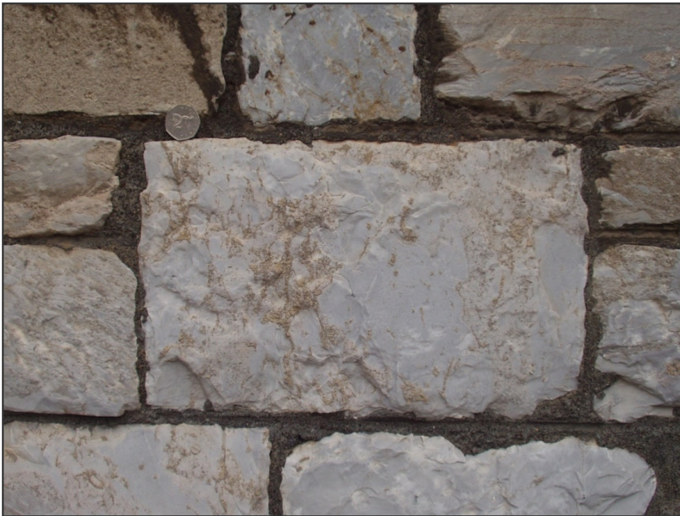
Figure 4. Emanuel parish church, Okehampton Road, Exeter. Fine-grained pale-grey limestone composed of calcite with streaks of fawn dolomite.
