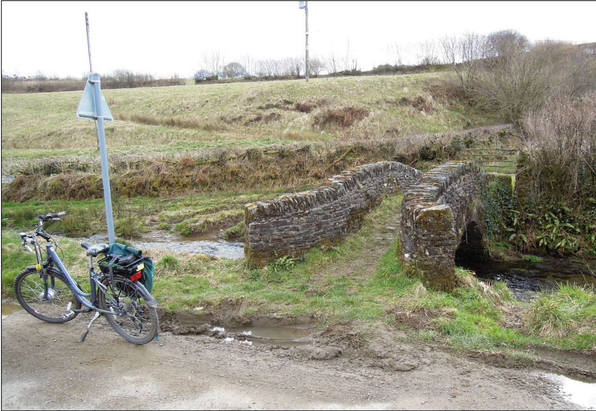
Figure 5. Packhorse bridge, Challacombe. The parapet is made of poorly cleaved slate weathered dark grey.
