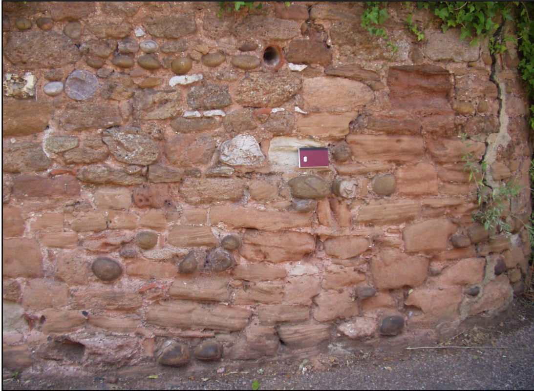
Figure 2. Wall on the west side of Little Knowle, Budleigh Salterton. Quartzite cobbles are mixed with Otter sandstone and mud flake conglomerate.
