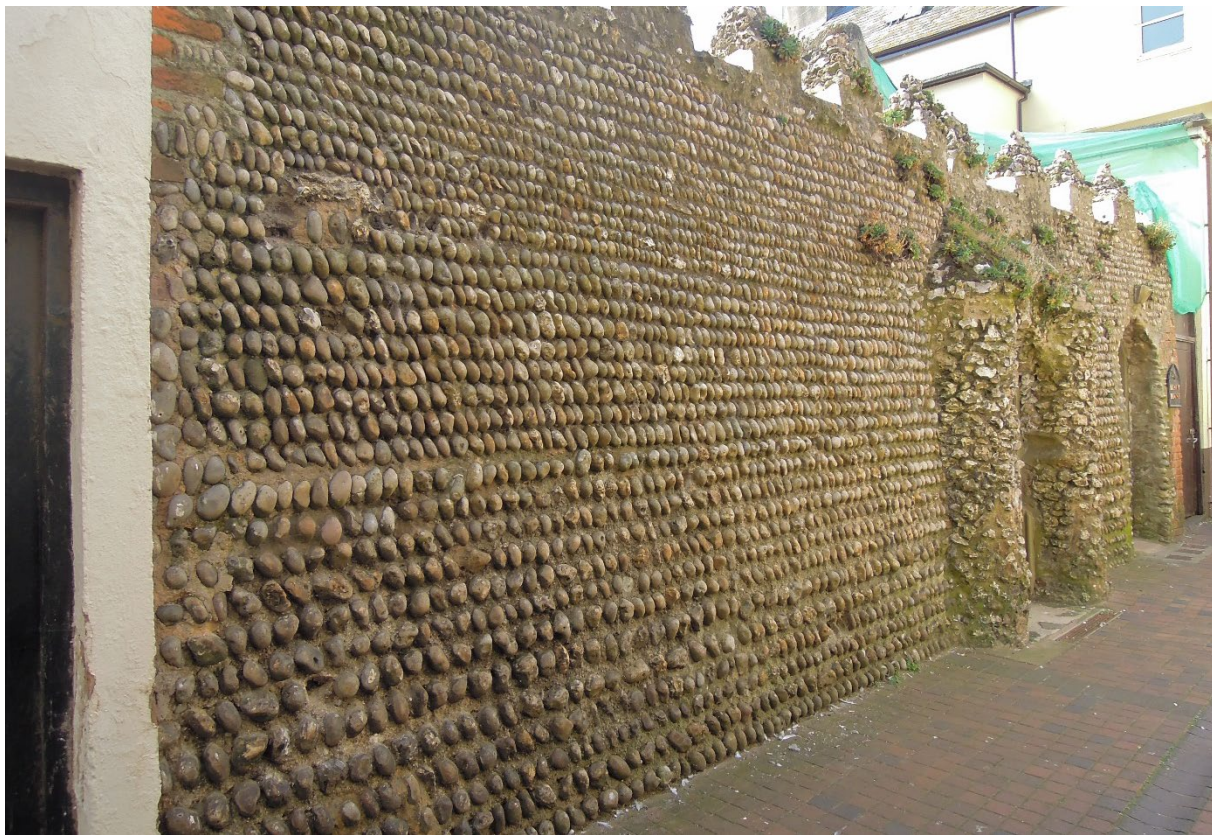
Figure 5. Wall of Beach House, Kings Lane, Sidmouth, of well-rounded chert cobbles collected from the beach with some “Buddleigh Buns” (Buddleigh Salterton Pebble Beds Formation, Code 36, qv).
