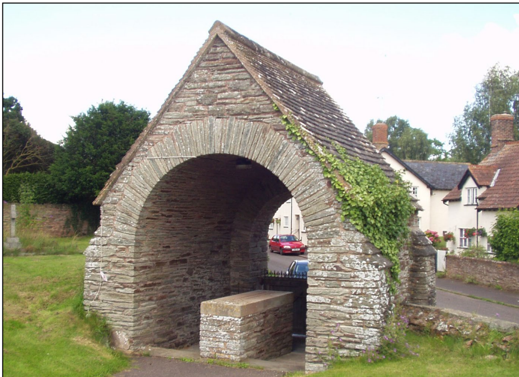
Figure 2. Lych gate and coffin rest of St Mary's, Cheddon Fitzpaine. The roof covering is of thin bedded Ham Hill Stone.
