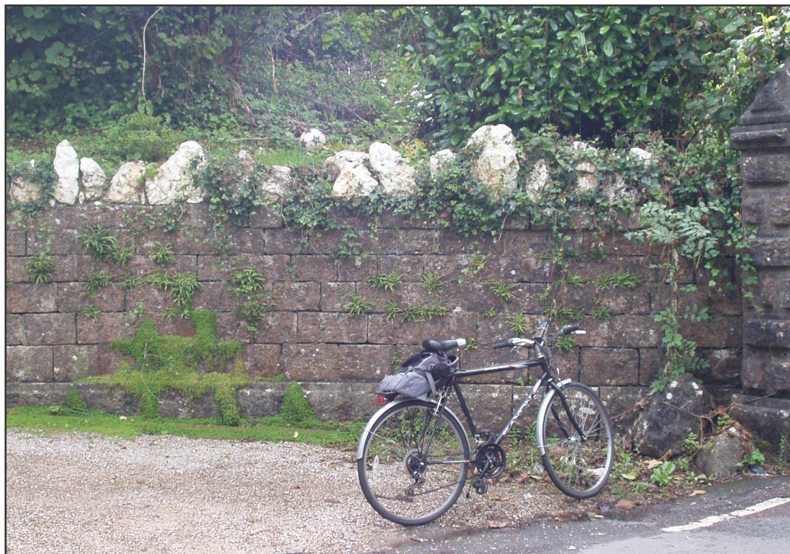
Figure 2. Boundary wall, the Old House, Compton. The wall is of medium-grey limestone. The coping is of vein quartz.
