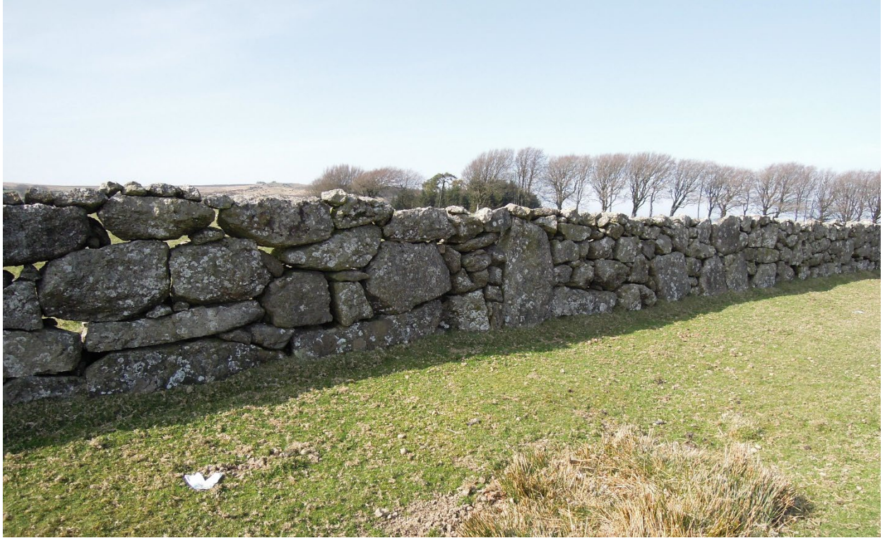
Figure 14. Drystone wall made of huge granite moorstones, approach to Fernworthy Reservoir.
