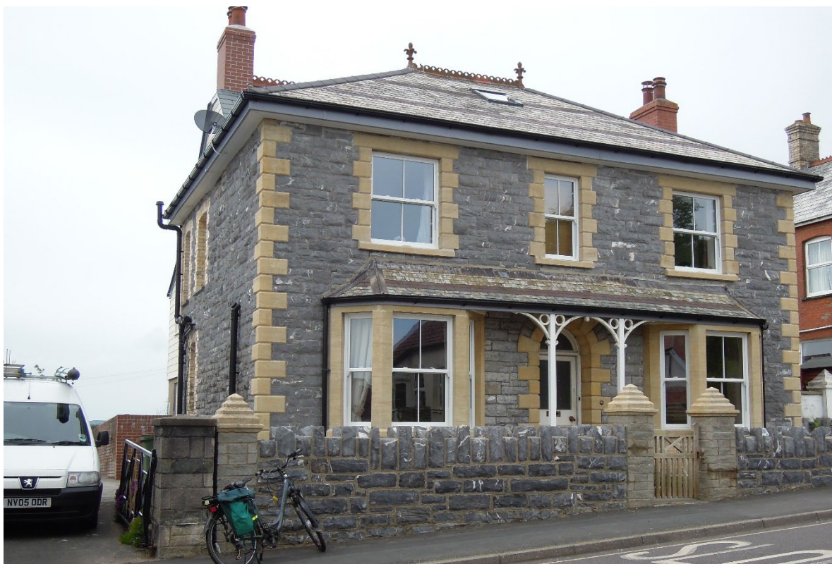
Figure 9. Bodmin Street, Holsworthy. Handsome C19 villa of dark grey limestone with Bath Stone quoins and dressings.
