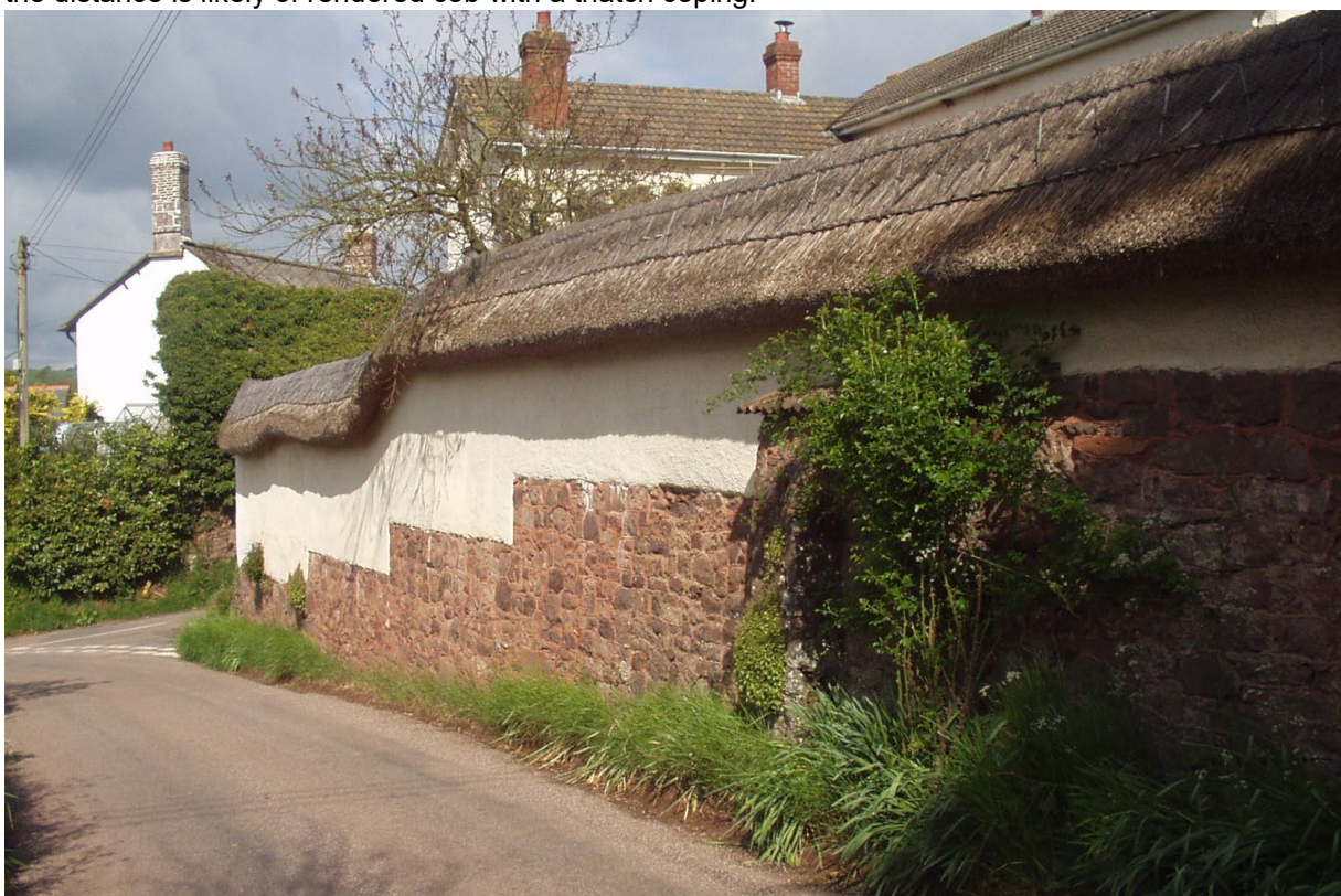
Figure 3. Boundary wall of Pollards, Yeoford. Rendered cob on a tall footing of Exeter volcanics.
