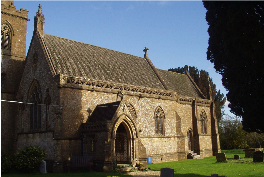
Figure 7. Church of St Mary Magdalene, Cricket Malherbie. The quoins and dressings are of Ham Hill Stone and the walling of Moolham Stone but these are indistinguishable from a distance.
