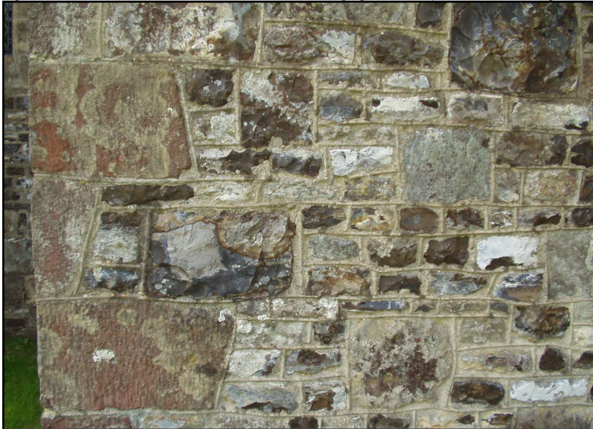
Figure 8. Church of St. Nicholas, Dunkeswell. Chert and cherty sandstone rubble with quoin of Upper Greensand sandstone on left.
