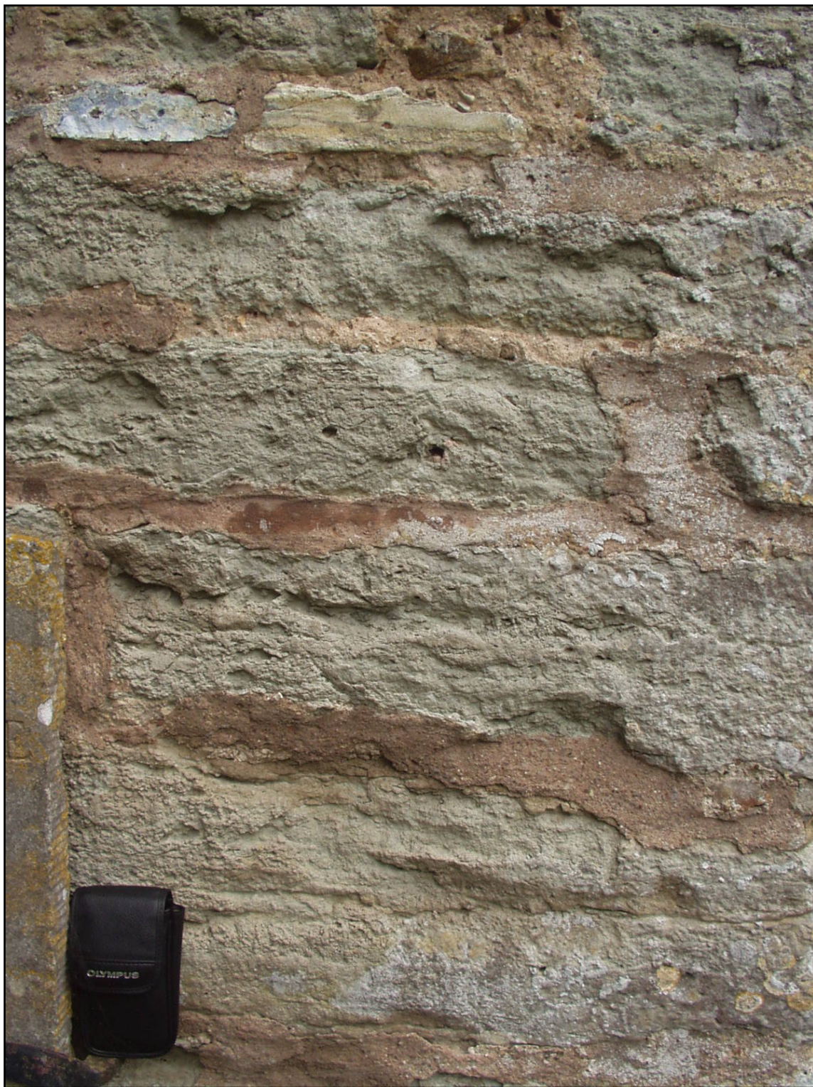
Figure 1. Tower of St Andrew's church, Feniton. Large slabs of grey-green sandstone with a greasy texture but lacking obvious dark minerals. It has a crude but quite well-defined bedding fabric.
