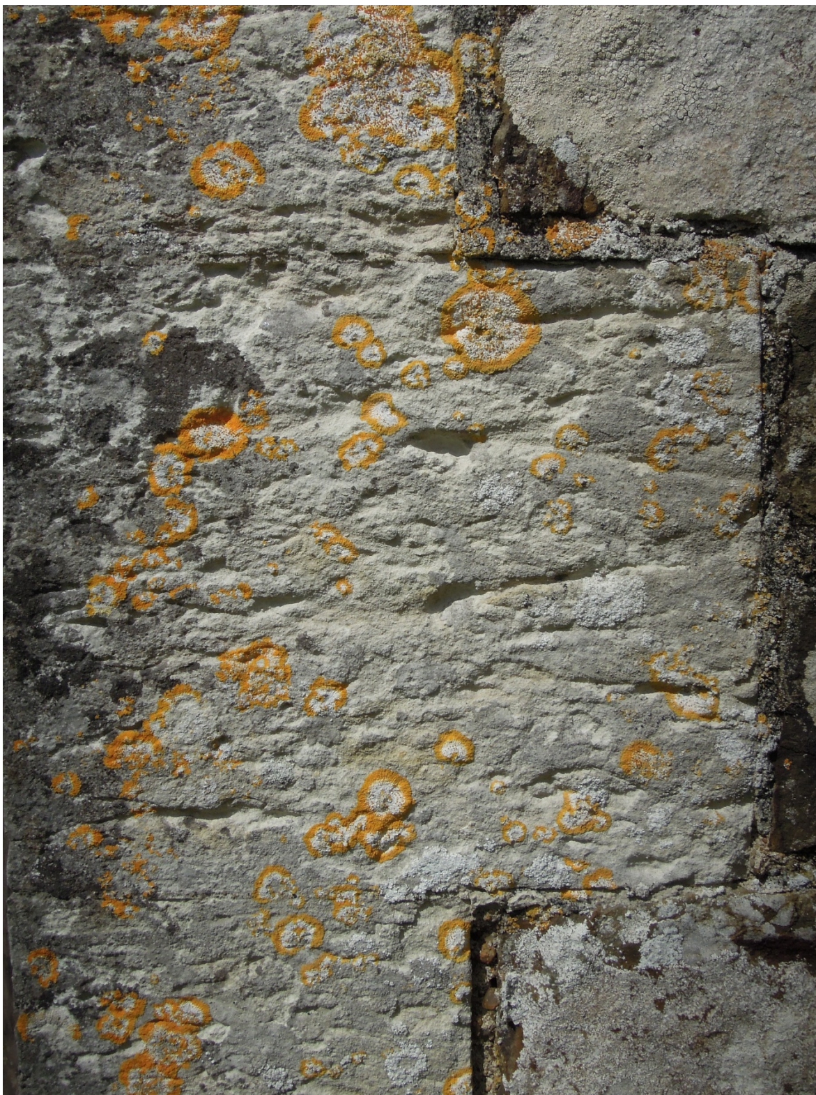
Figure 12. Quoin of the chancel of St George's church, George Nympton. The Beer Stone shows sub-parallel fractures roughly following to the bedding.
