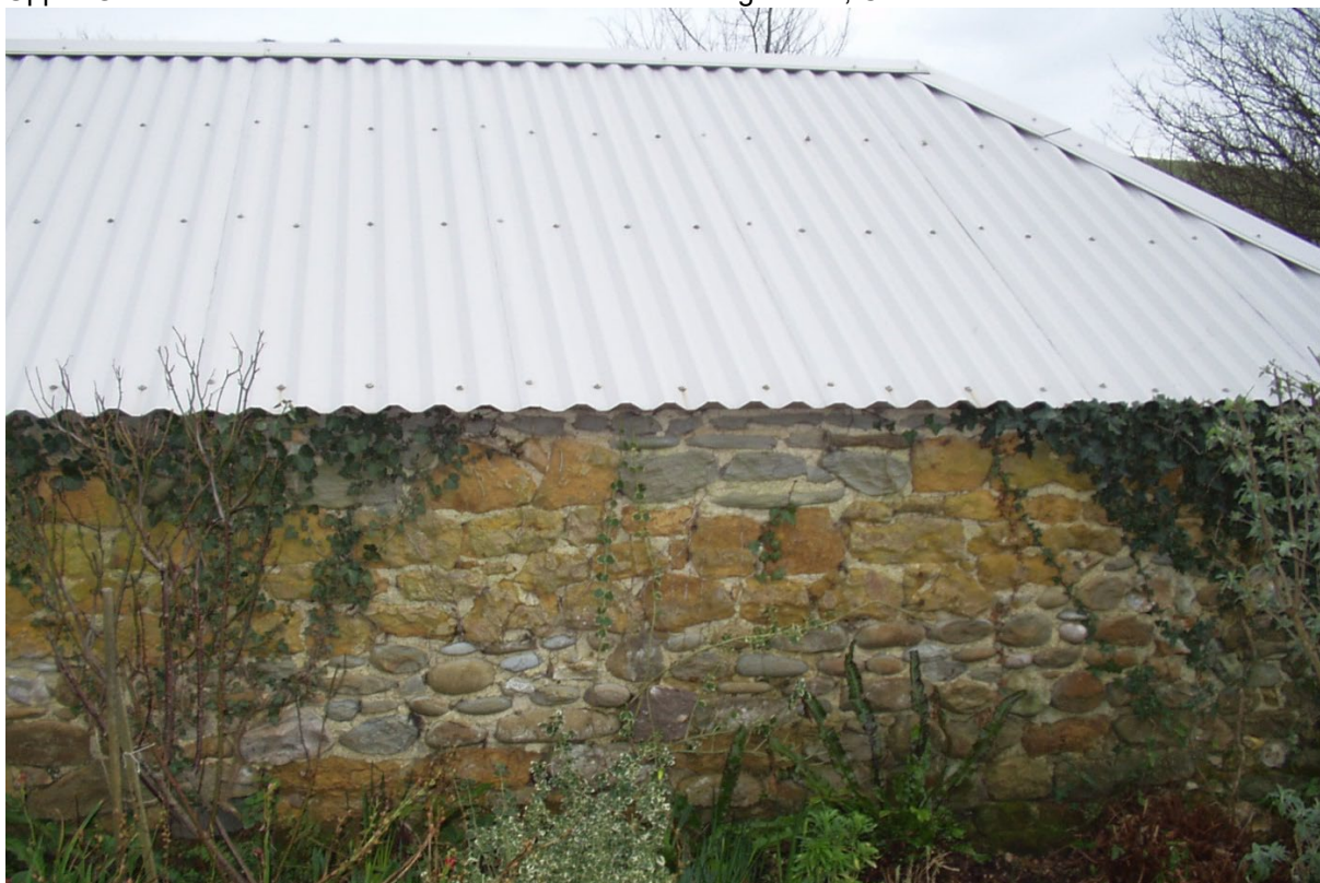
Figure 2. Rounded boulders of grey siltstone associated with yellow Inferior Oolite limestone. Outbuilding adjacent to Mill House, Sea Town.
