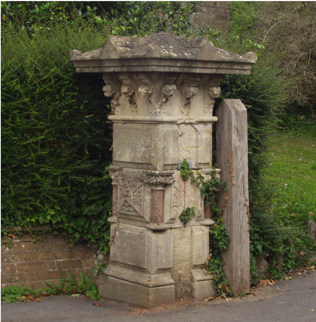
Figure 1. Decorative gatepost, east side of South Road, Taunton. Made of Bath Stone with short pillars of red sandstone.
