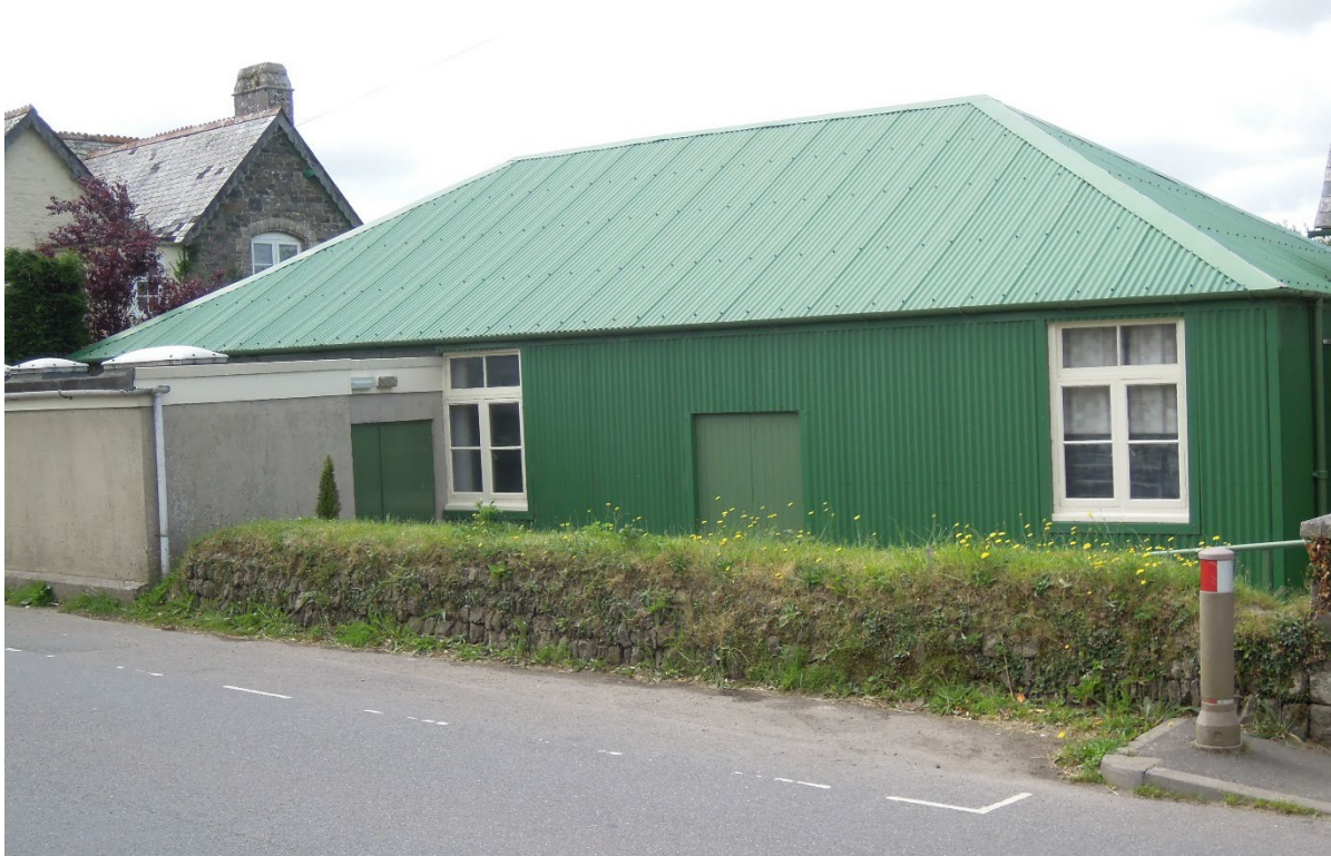
Figure 8. Village Hall, Milton Abbott. The hall was recently refurbished. The planning authority insisted that the hall should retain the corrugated iron finish.
