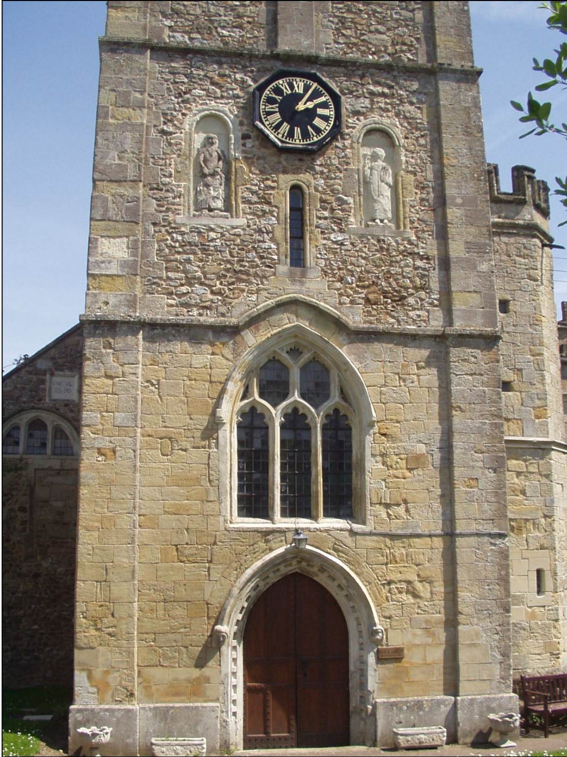
Figure 2. St Giles' church, Sidbury. Lower part of the tower is of Salcombe Stone ashlar with Beer Stone Inserts; upper part is of chert rubble with Salcombe Stone quoins. Dressings are mainly of Beer Stone including the bas reliefs which came from elsewhere in the church. Repairs to the stone of the tower are in finer-grained Salcombe Stone, possibly from Dunscombe.
