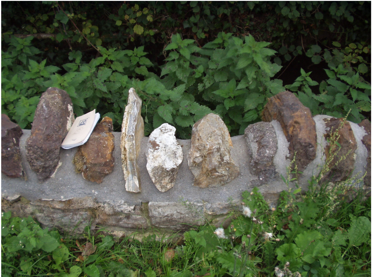
Figure 1. Roadside wall at Fulwood, Somerset. The stones of the coping at the right and left of the photograph are of dark red gossanous sandstone.
