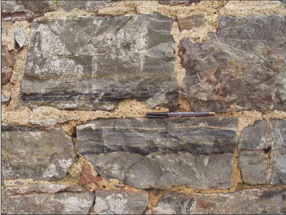
Figure 5. Electricity substation, Ferry Road, Topsham, at junction with Follet Road. Note the black chert bands and the “muddy” colour of the stone which contrasts with the colour of limestone from Torbay and Plymouth.
