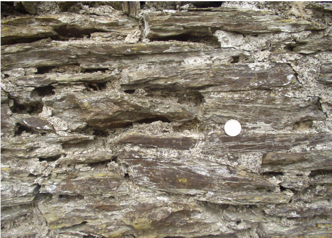
Figure 11. Grey indifferently cleaved slate, wall north side of Roborough Lane, Ashburton.
