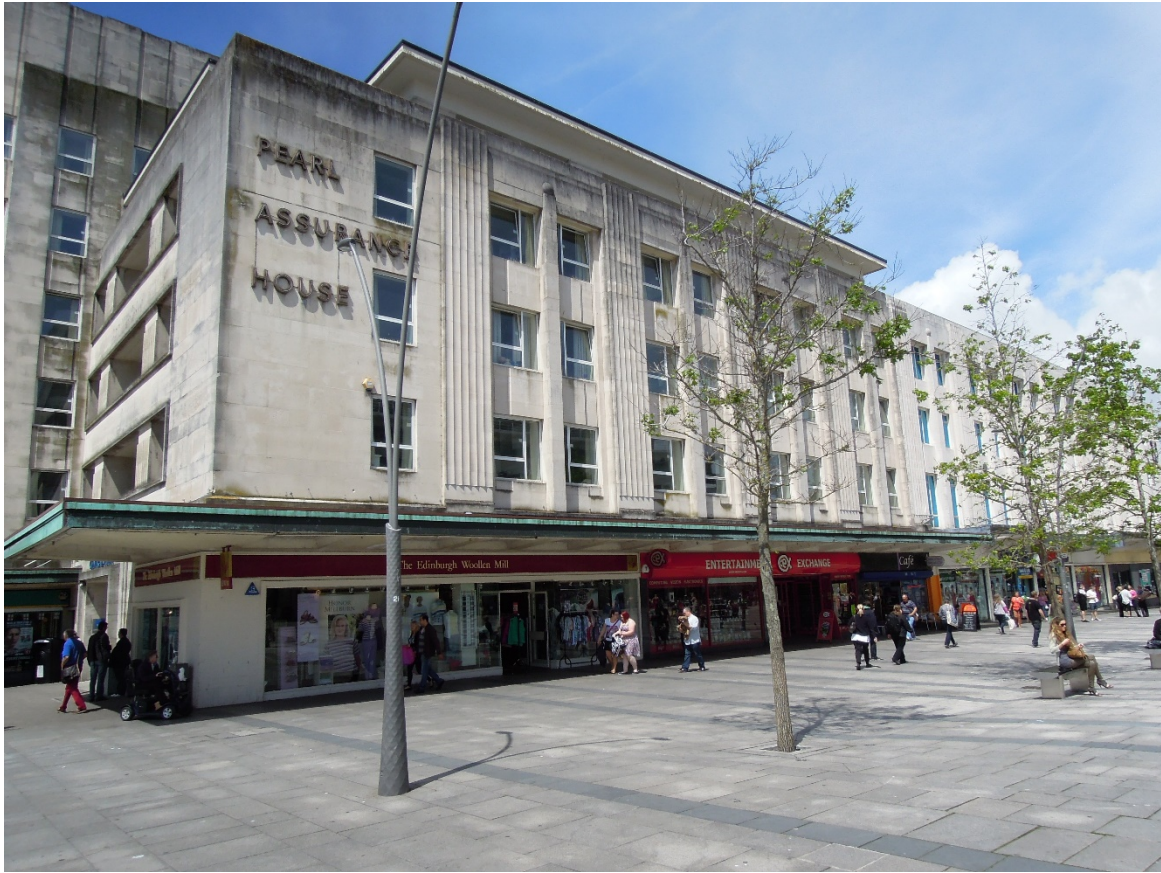
Figure 8. Pearl Assurance House, New George Street, Plymouth. Portland Stone cladding.
