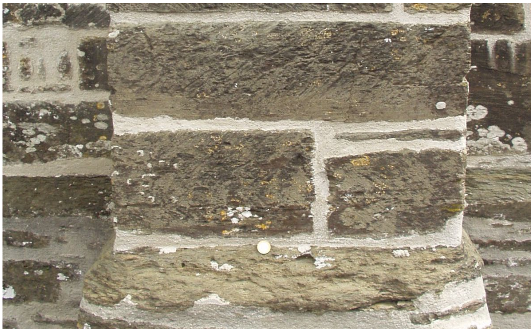
Figure 6. Black-stained slate with red sandstone dressings round door, west end of St Peter's, Cornworthy. Detail of the right buttress below shows the characteristic buff weathering.
