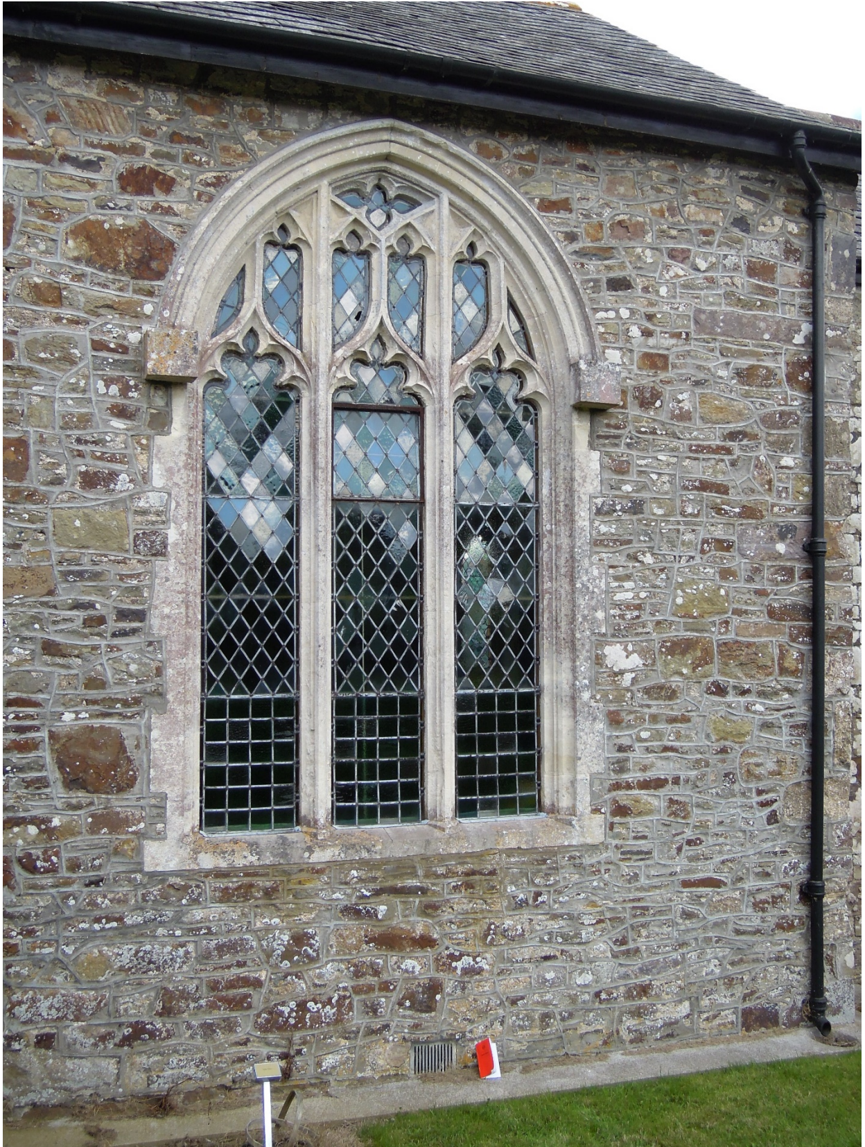
Figure 4. Beer Stone window dressings, south side of nave, St George's church, George Nympton. The wall is made of Bude sandstone rubble.
