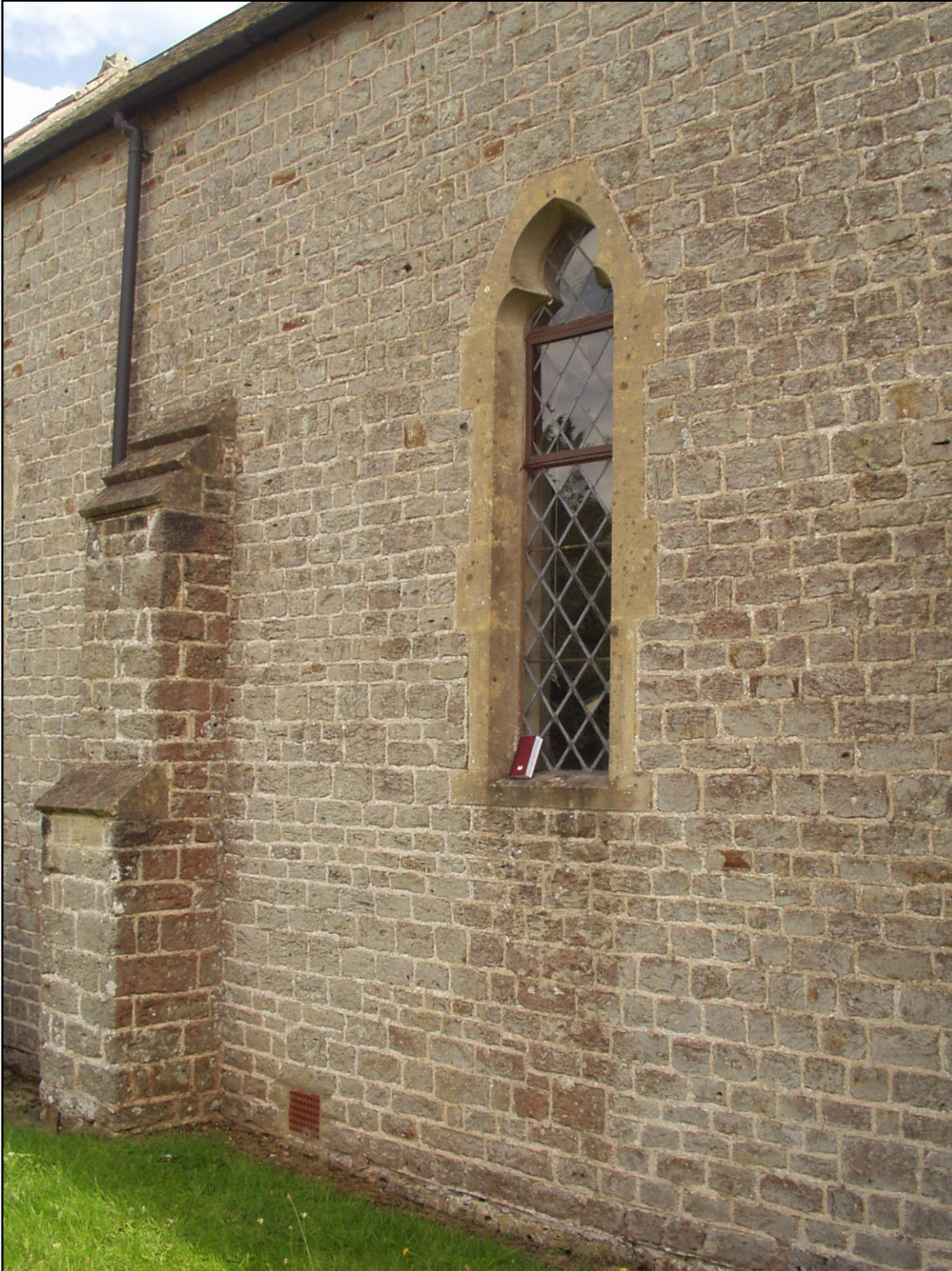
Figure 3. United Reformed Church, Plymtree. Grey-green glauconitic sandstone as regular small blocks laid as coursed rubble. The dressings round the window are of Bath Stone.
