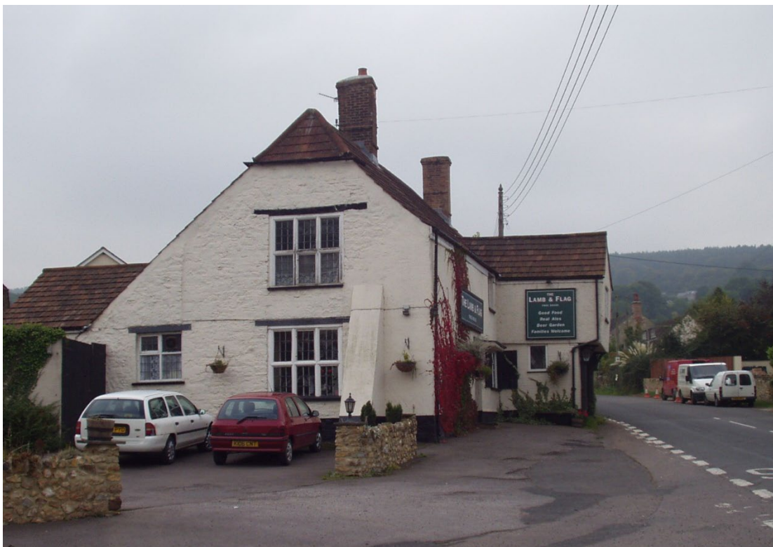
Figure 4. Lamb and Flag public house, Blagdon Hill. The porch is jettied and supported on timber posts.
