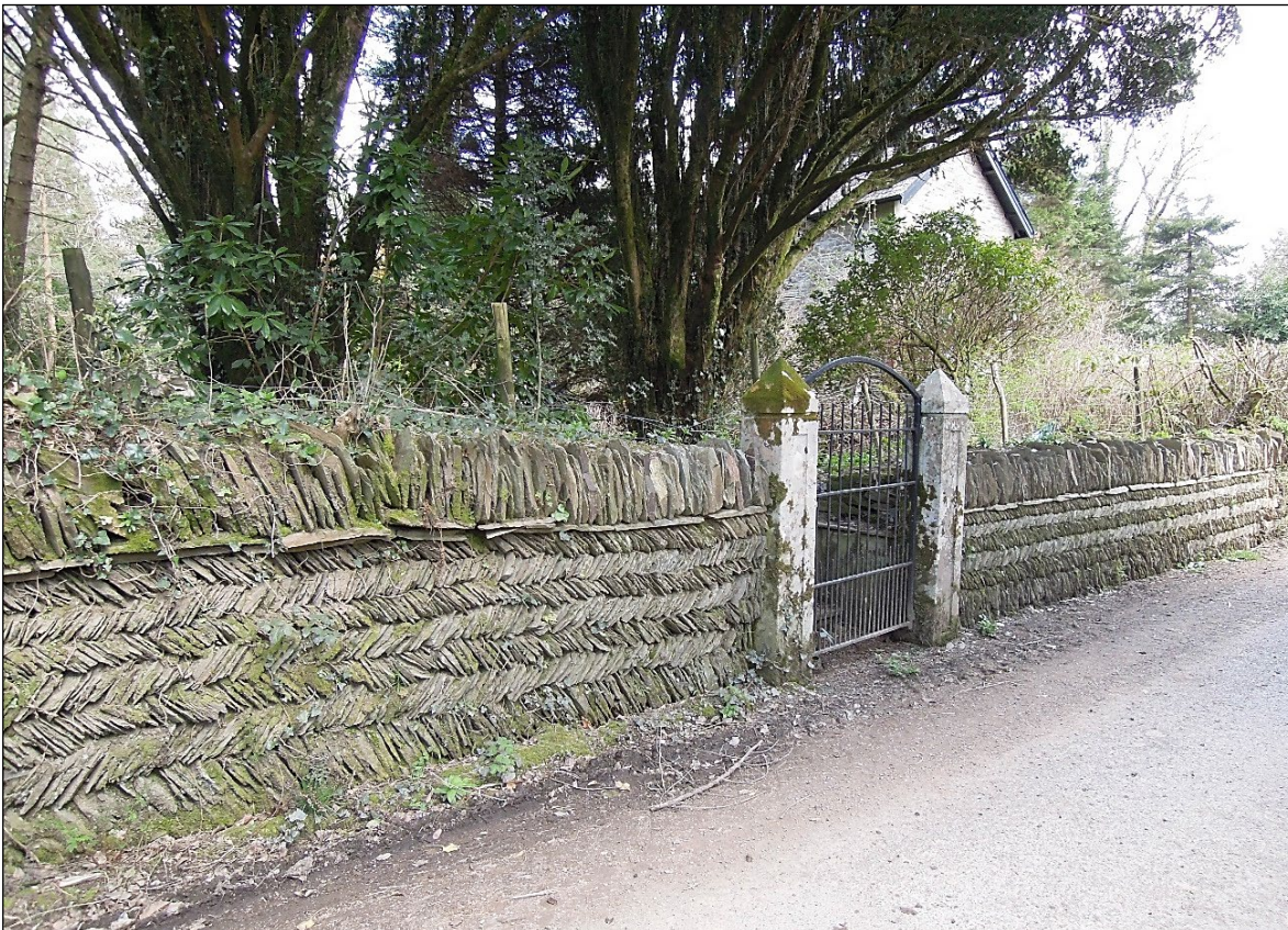
Figure 6. Wall of Morte Slate laid in a herring-bone pattern. Roadside wall, Arlington village.
