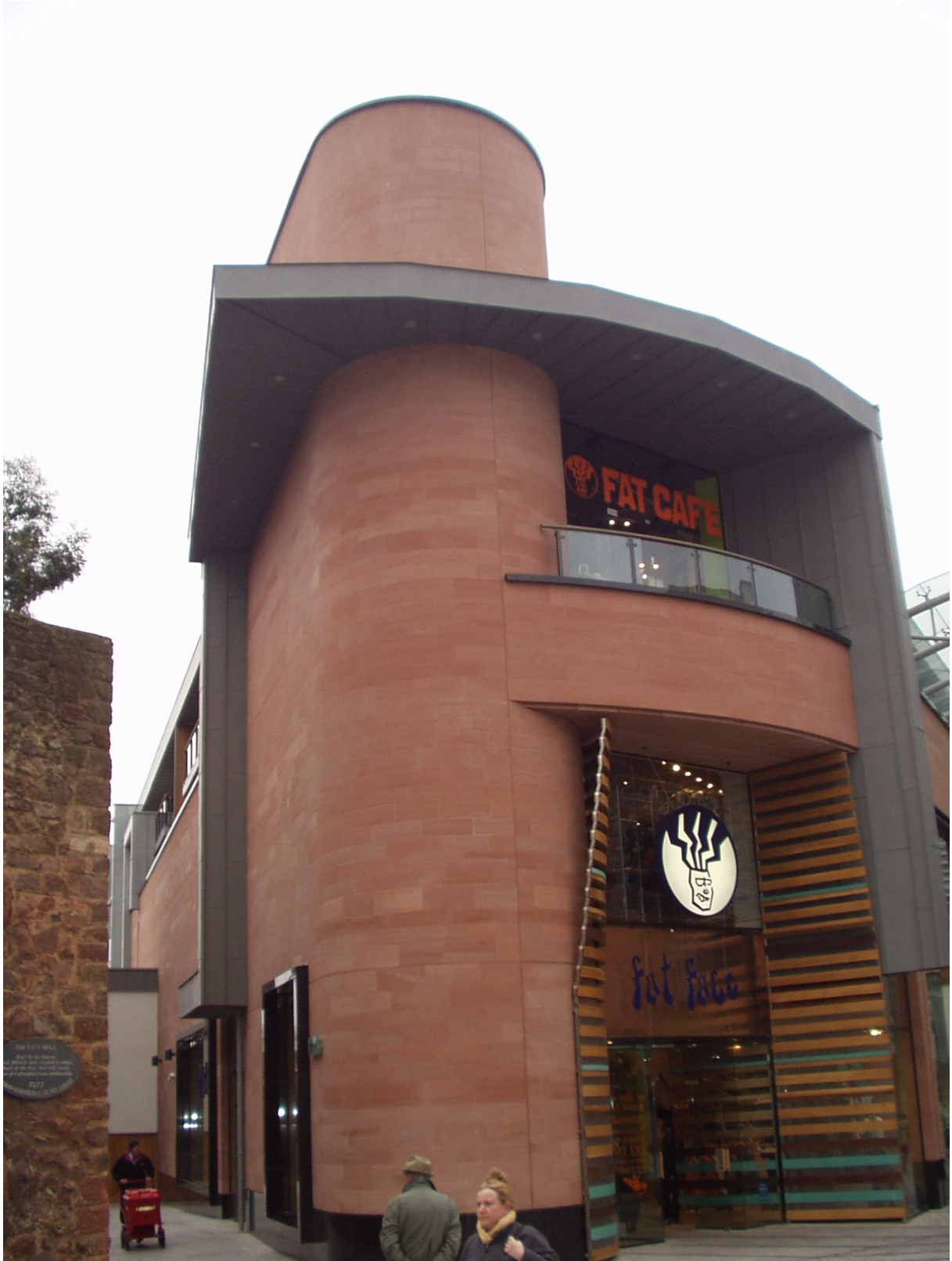
Figure 5. Part of the Southernhay development, Exeter. The beams and roof support are of concrete. The cladding is of Plumpton Red Lazonby sandstone from Stencliffe Stone of Penrith.
