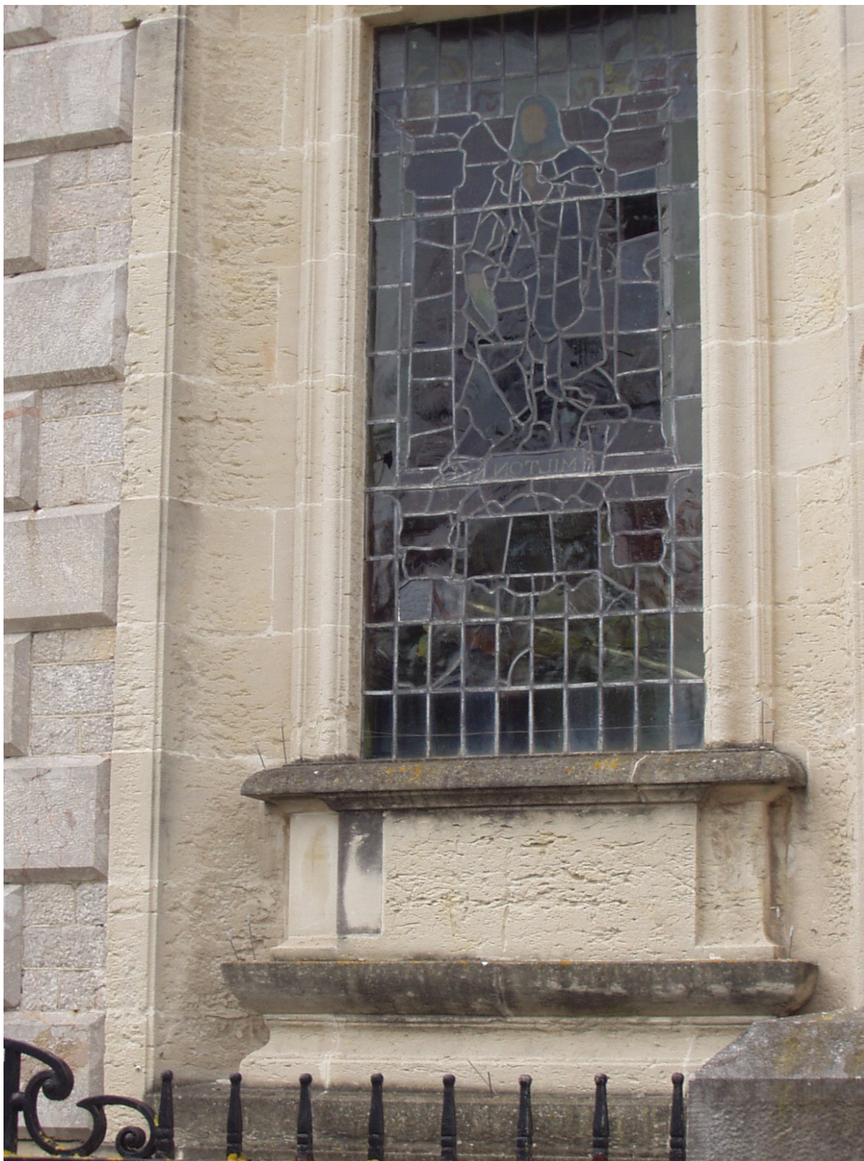
Figure 13. Detail of the Beer Stone window dressings of the Town Hall, Castle Circus, Torquay showing characteristic sub-parallel fractures defining the bedding.
