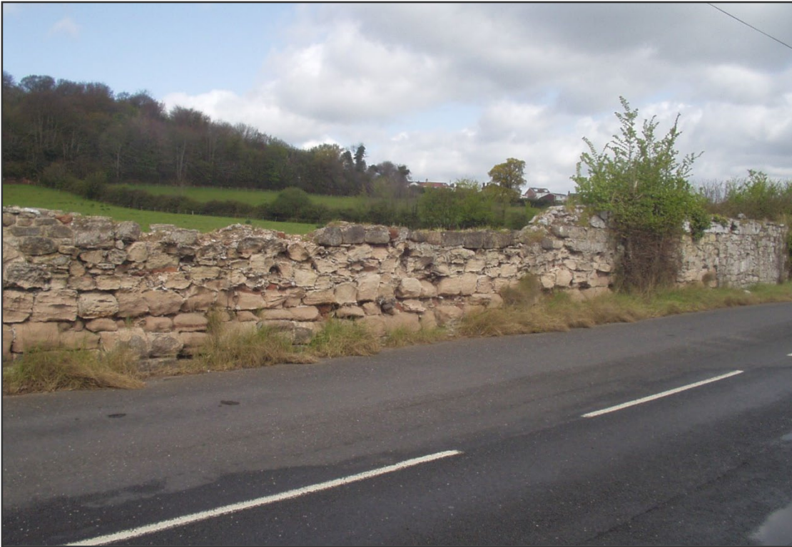
Figure 6. Roadside wall, Dawlish Warren. The closer part of the wall is made of easily eroded fawn sandstone. The further part is of limestone from Torbay.
