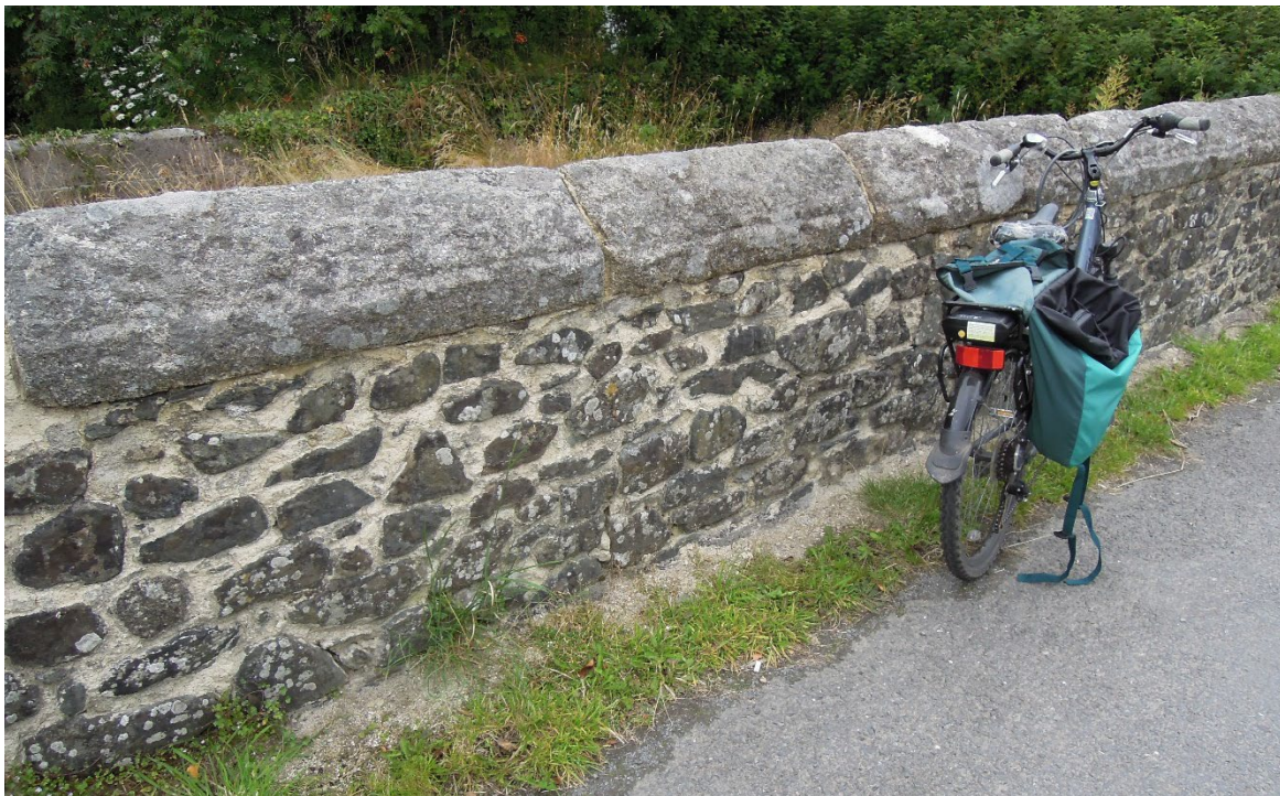
Figure 9. Parapet of the bridge over the Mill Leat in the centre of Peter Tavy. The coping is of Dartmoor granite.
