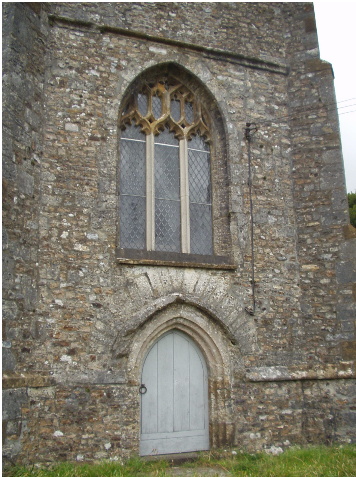
Figure 8. St Leonard's church, Birchwood. The dressings and relieving arch of the west door are of Beer Stone discoloured by weathering. The dressings of the west window were not identified. The walls are mainly made of chert rubble.
