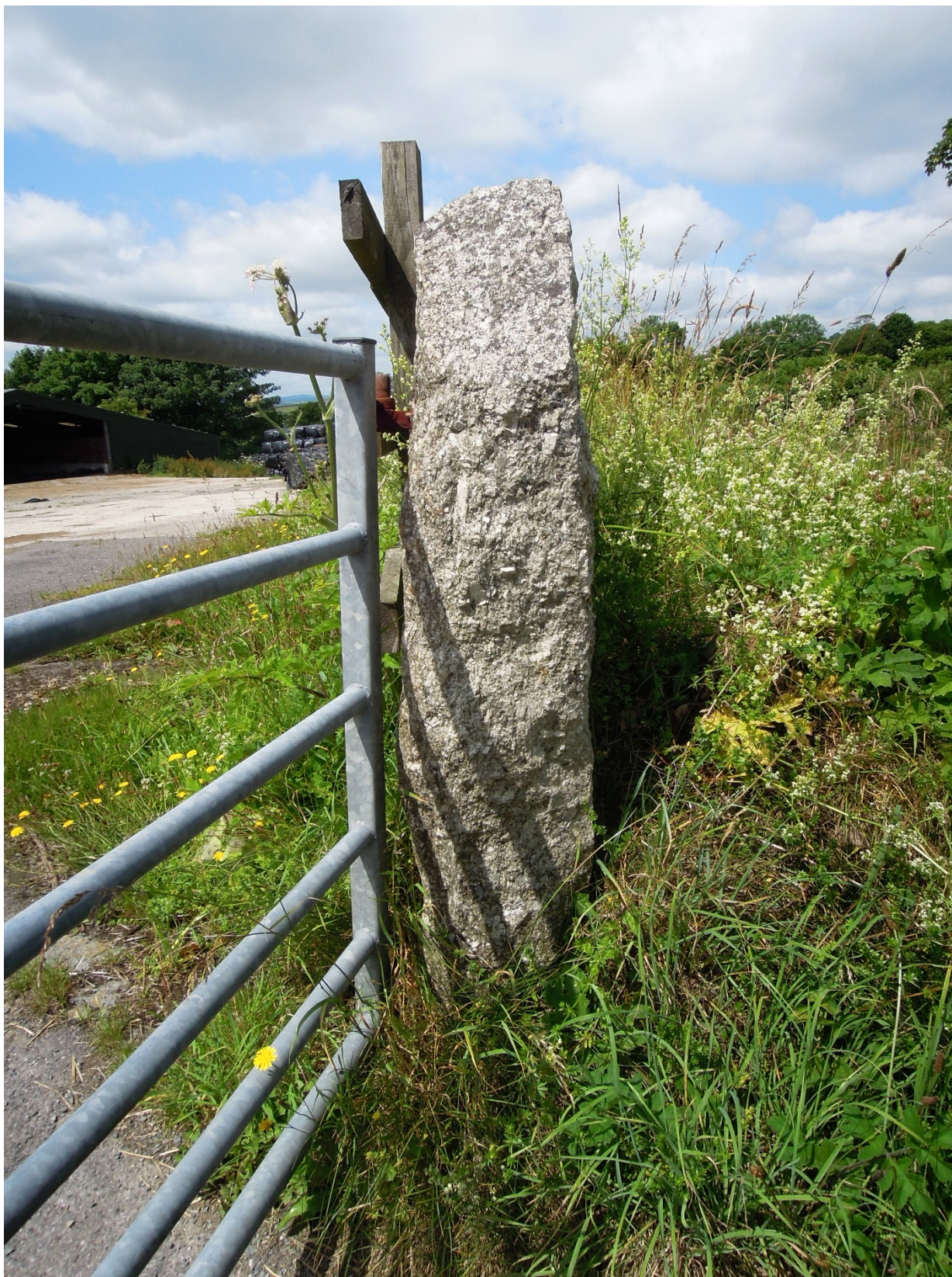
Figure 16. Typical rough-hewn monolith granite gatepost. David Ball Bull Hire, Milton Abbot.
