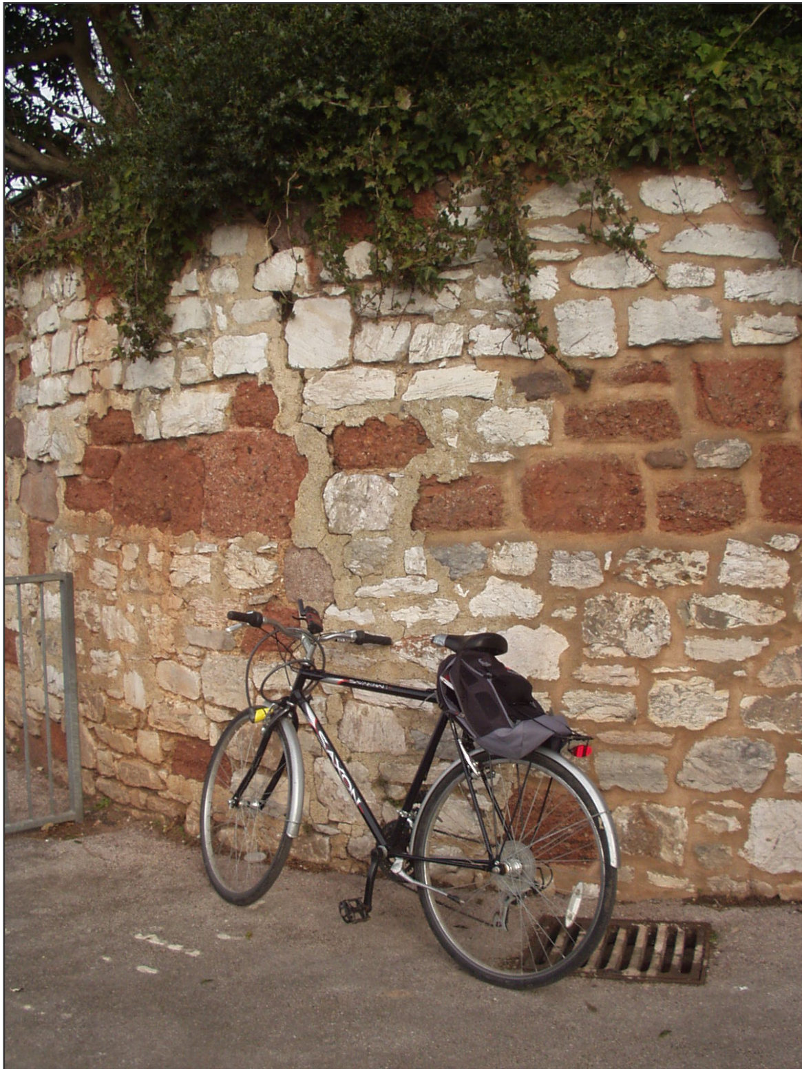
Figure 7. Junction of riverside walk with Larkbeare Road at Port Royal public house, Exeter. Heavitree Breccia and pale grey limestone from Torbay.
