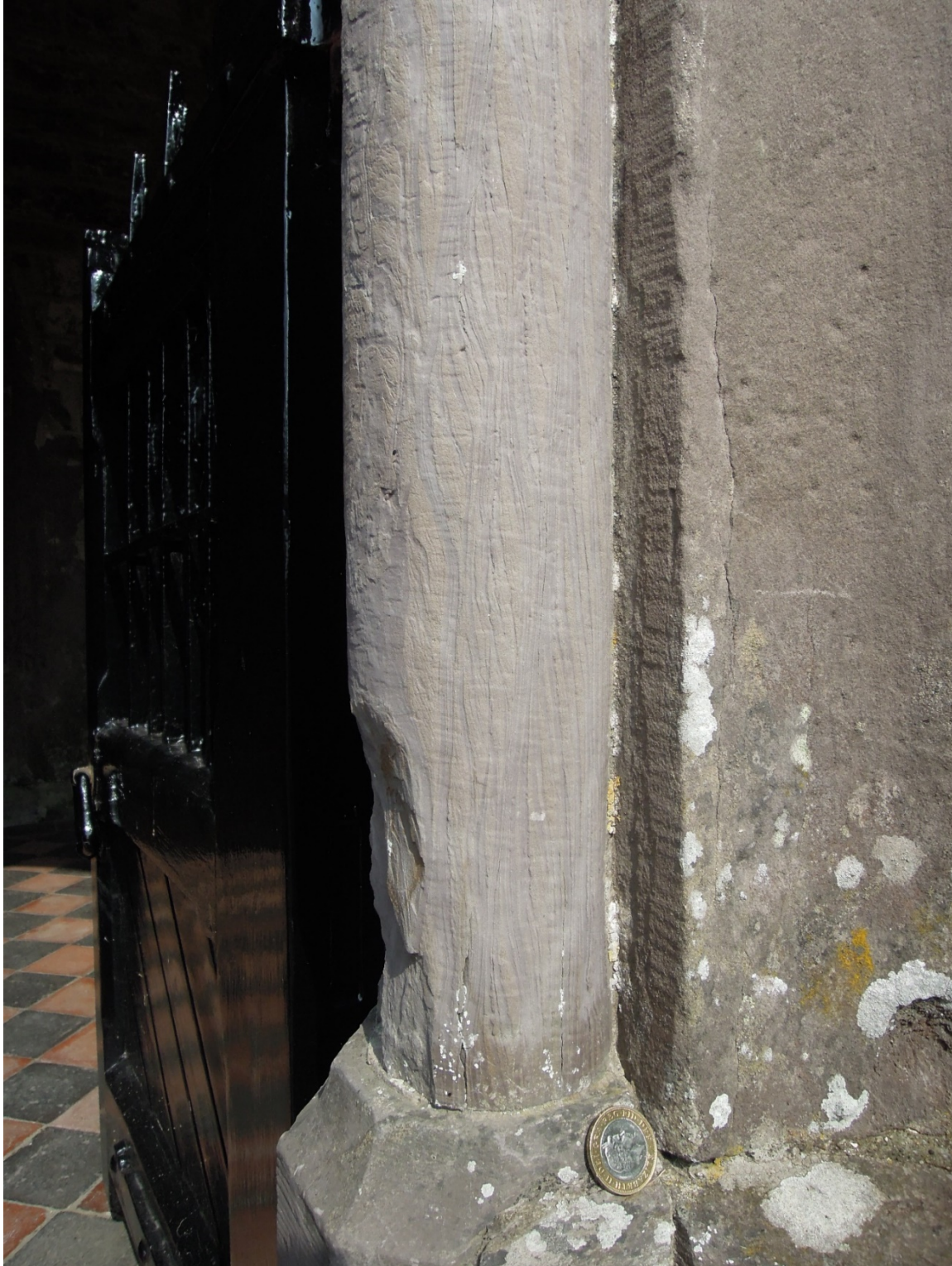
Figure 10. South porch of All Saints, North Molton. The door jambs are made of single slabs of purple cross-bedded sandstone set on edge, a very common usage of the stone in the dressings of medieval churches.
