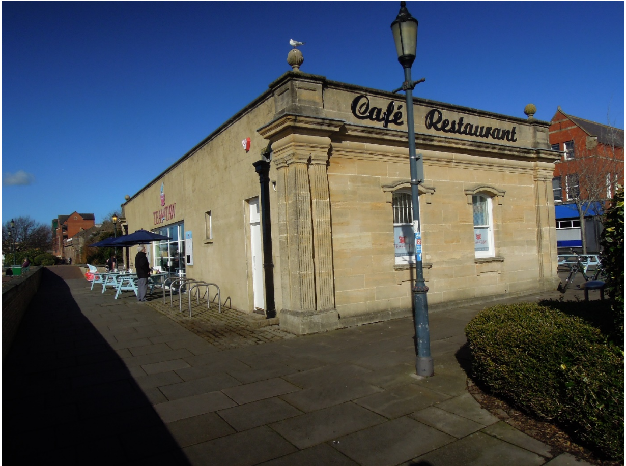
Figure 4. Tea by the Taw Restaurant, Barnstaple. Most of the building including the quoins and dressings is of Douling Stone but the wall facing the river (on the left of the photo) is of artificial stone carefully matched for colour with the Douling Stone.
