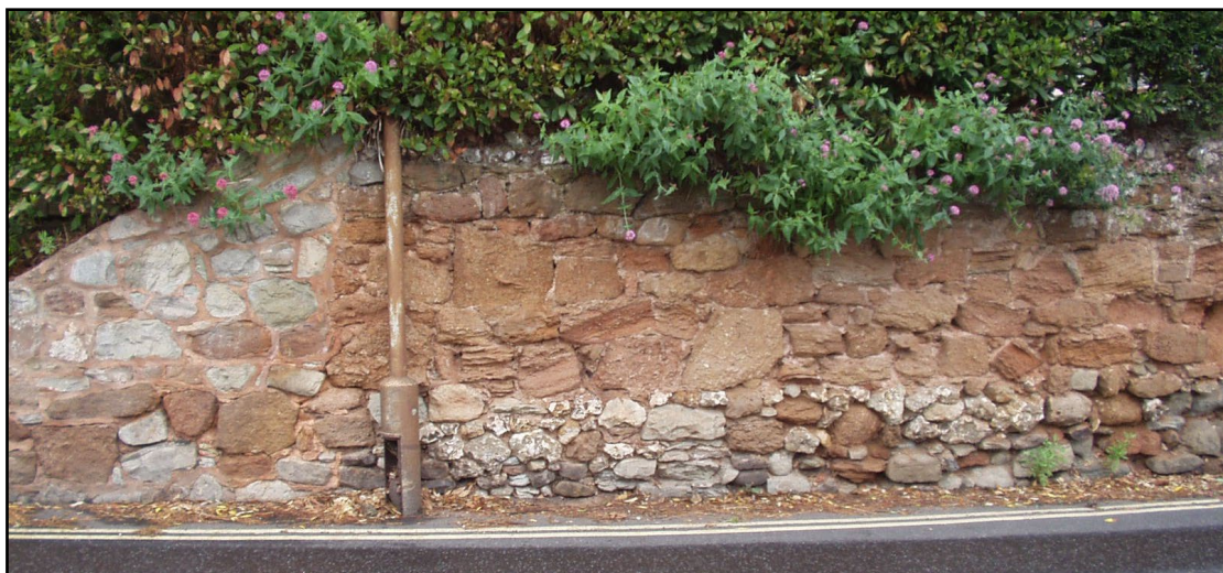
Figure 1. Cotmaton Road, Sidmouth. Otter Sandstone and conglomerate with glauconitic sandstone (Upper Greensand) in the footing.
