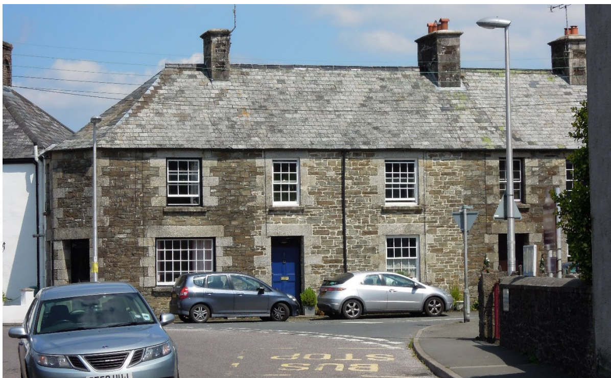
Figure 28. Nos 1 and 2 Rectory Road, Bridestowe. Crackington Formation sandstone with quoins and dressings of Dartmoor granite.
