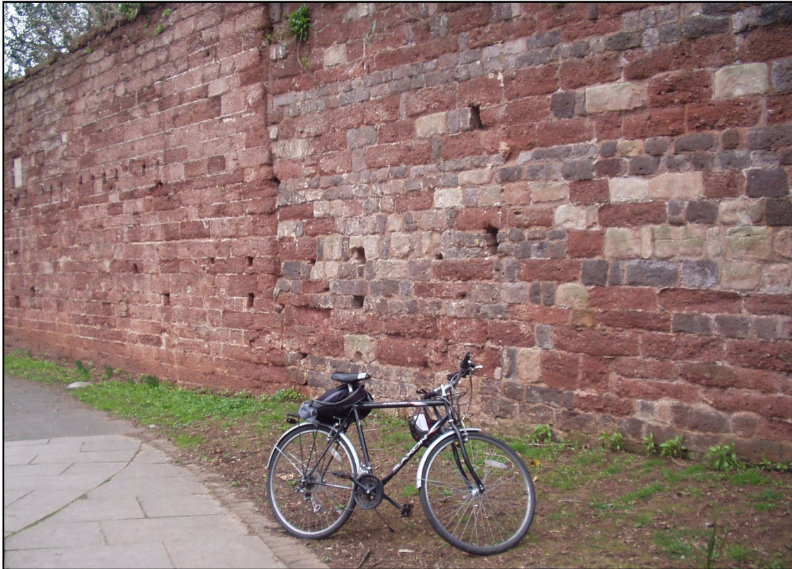
Figure 4. Exeter city wall. The red stones are of Heavitree breccia, the cream ones are of sandstone from the Exeter Group and the grey (with a touch of purple) stones are vesicular lava, probably from Rougemont or Northernhayes.
