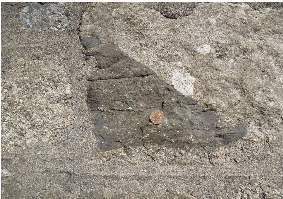
Figure 12. Inclusion of dark slate or hornfels attached to granite block. Church of St John the Baptist, Leusdon.
