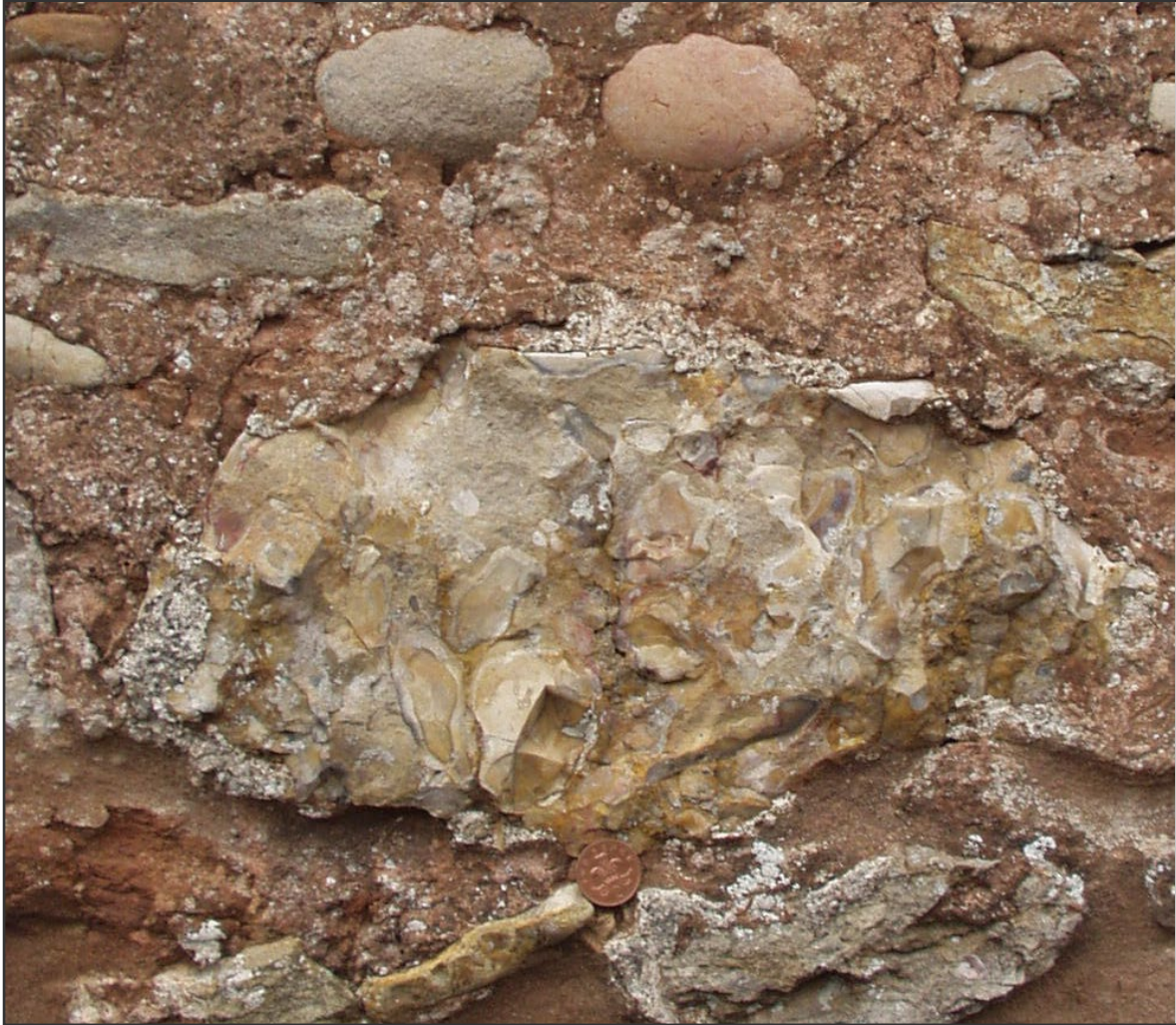
Figure 2. Block of chert breccia in the rubble wall of St Luke's church, Newton Poppleford. The wall is made of a mixture of materials including also Otter Sandstone and rounded cobbles of quartzite from the Budleigh Salterton Pebble Beds Formation.
