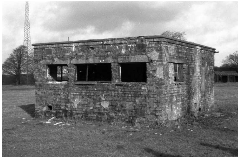
Figure 21: Battery Charging Room (Old Watch Office) 1a (32)
