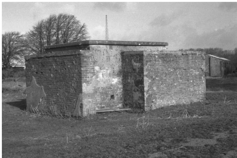
Figure 18: Main inlet electrical sub-station to drawing 12648/40. 6 (28)
