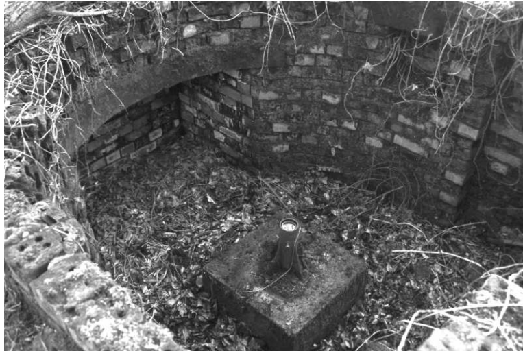
Figure 34: Gunpit showing gun mounting point. 530 (52)
