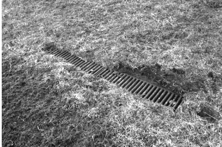
Figure 3: Cast-iron runway drain cover
