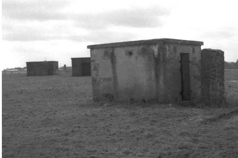
Figure 23: Aviation Petrol Installation – Pump House 8 (32)
