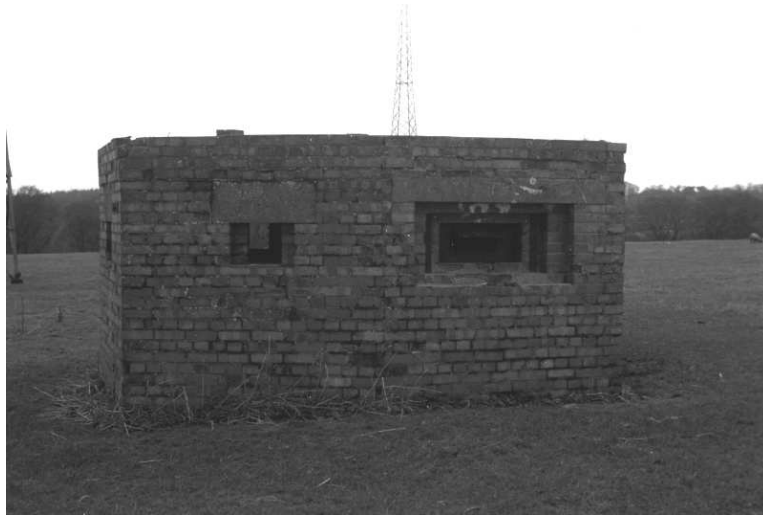
Figure 13: Pillbox. Note steel shutter fixed to large loophole. 518 (14)
