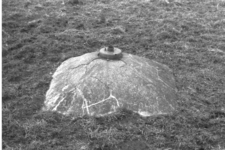
Figure 27: Signals Mast Fixing Block
