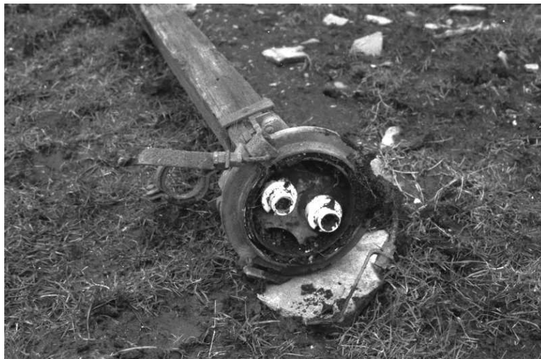
Figure 26: Control Tower Obstruction Lighting Fitting
