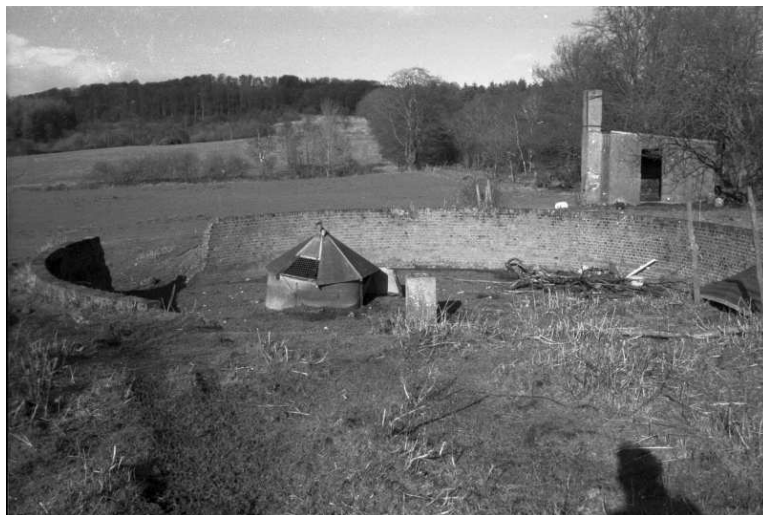
Figure 49: Septic Tank and Destructor House on the Sewage Disposal Site.
