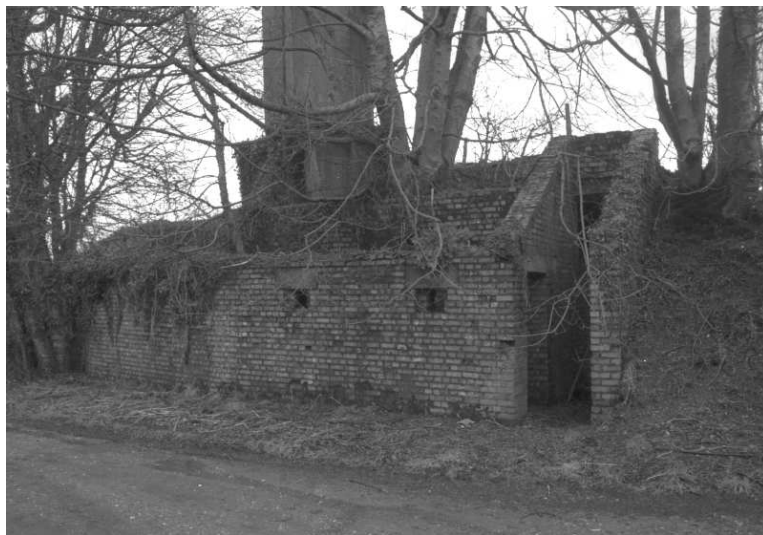
Figure 40: Angled Defended Wall at the rear of Pen 229 (57) and exit from air-raid shelter
