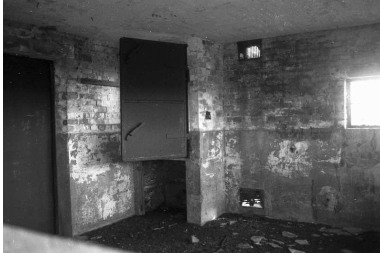
Figure 22: Interior view of Old Watch Office showing steel door of Pyro Cupboard. 1a (32)
