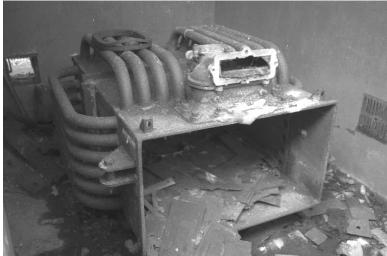
Figure 19: Transformer inside Main Inlet Electrical Sub-Station 6 (28)
